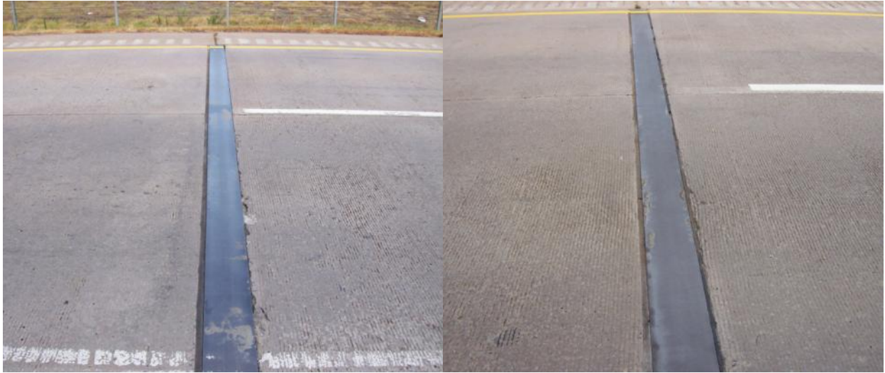
Figure 3.52 – Terminal joints at north bound beginning and end
