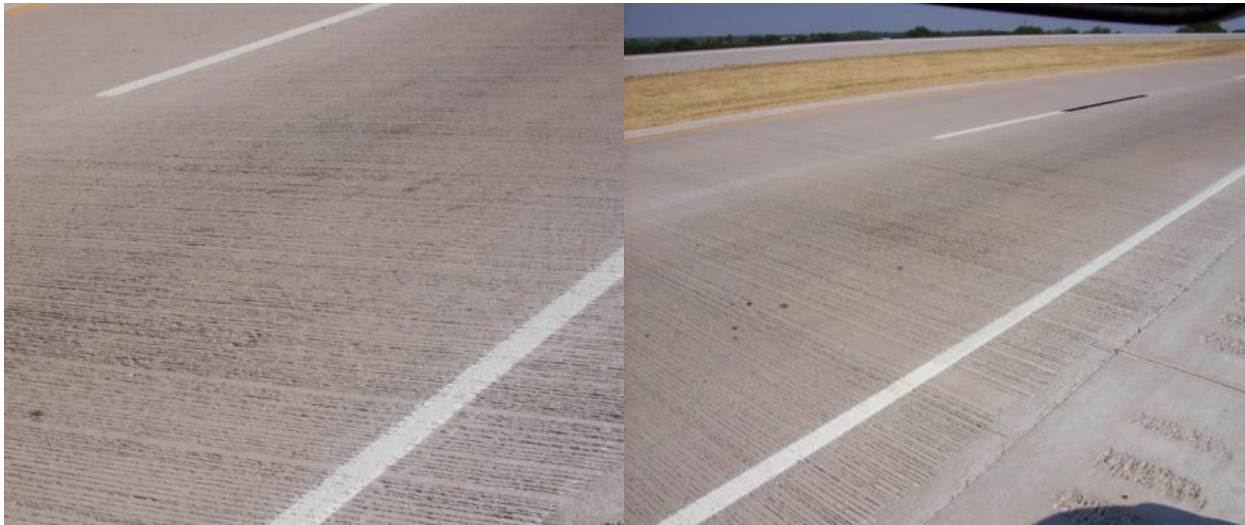
Figure 3.18 – Two images showing the glossy pavement surface with little wear
