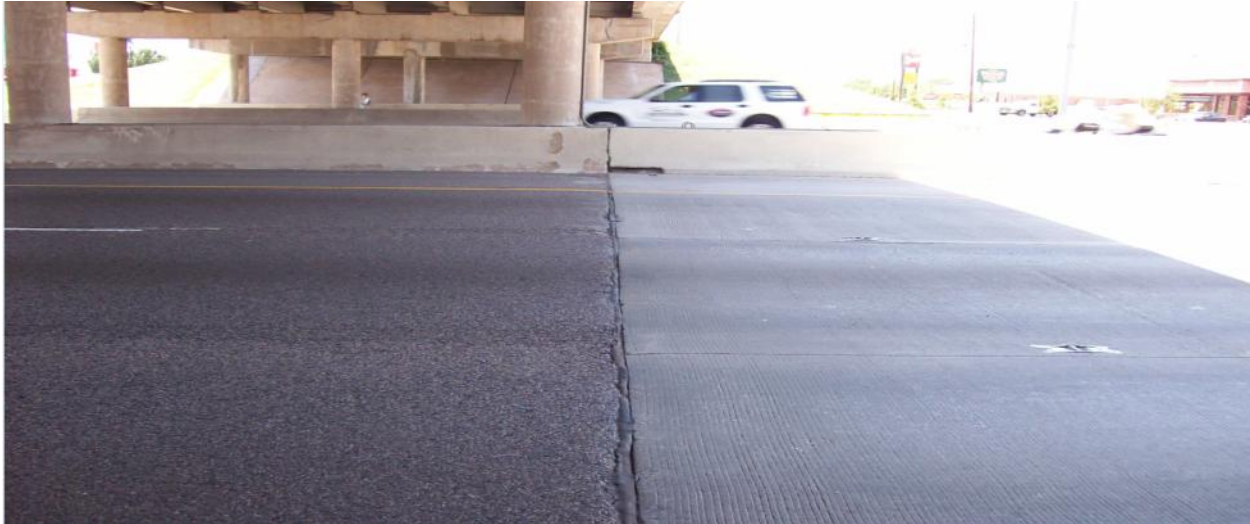
Figure 3.13 – Joint at the Southern end of North bound lane
