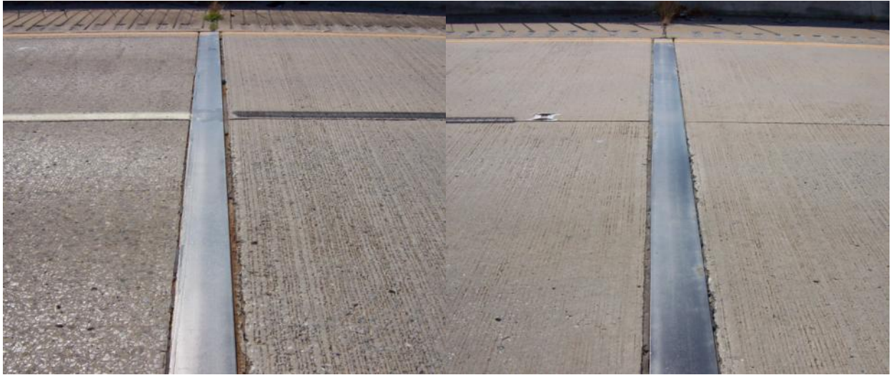
Figure 3.63 – Terminal joints at the project beginning and end
