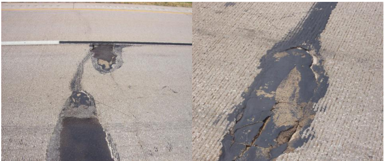
Figure 3.27 – Y-shaped patches
