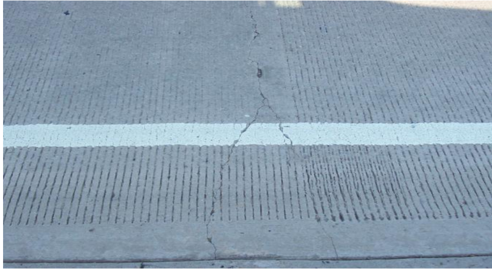
Figure 2.2 - Y-cracking example
