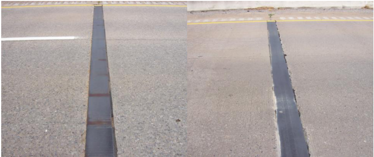
Figure 3.61 – Terminal joints on each end of the project
