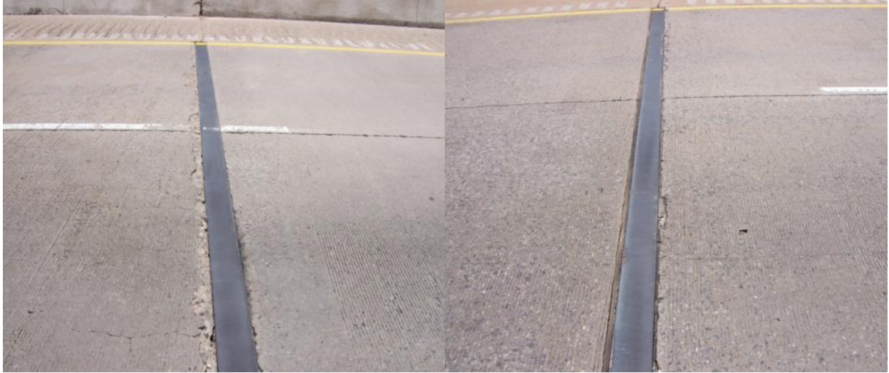
Figure 3.66 – Terminal joints at project beginning and end
