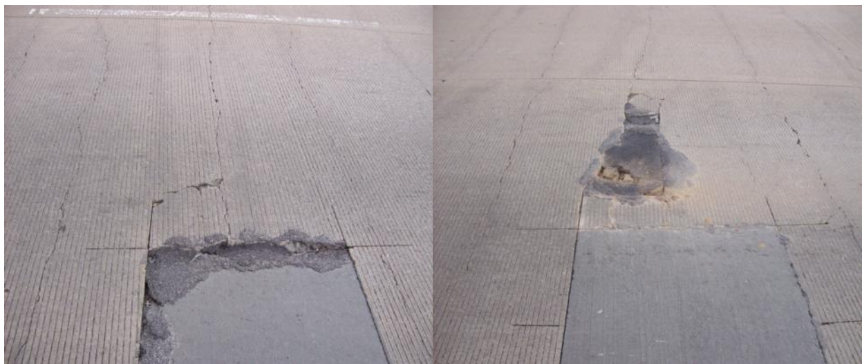
Figure 3.32 – Small patch with distress developing close by
