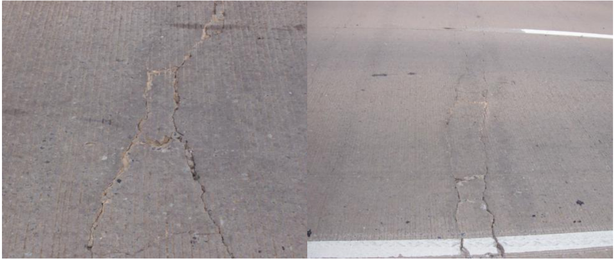
Figure 3.54 – Two developing punch-outs
