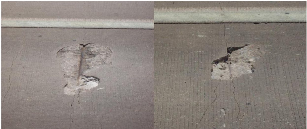
Figure 3.11 – Possible Y-crack over shallow transverse steel
