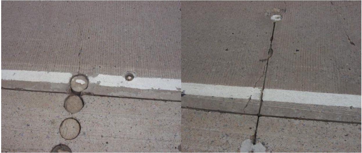
Figure 3.58 – (left) cores taken from shoulder, (right) core with censor wire extending to shoulder
