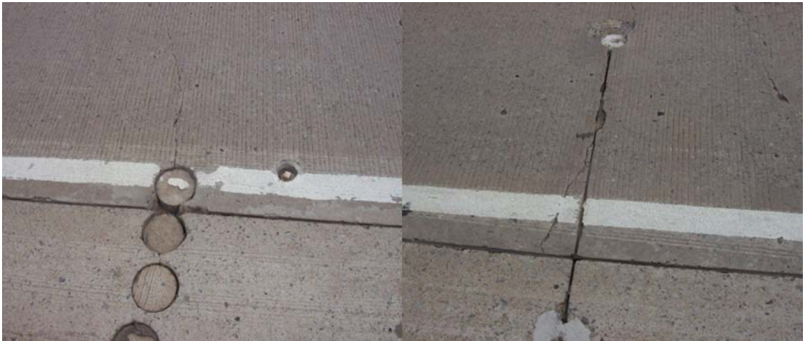
Figure A.58 (left) cores taken from shoulder, (right) core with censor wire extending to shoulder
