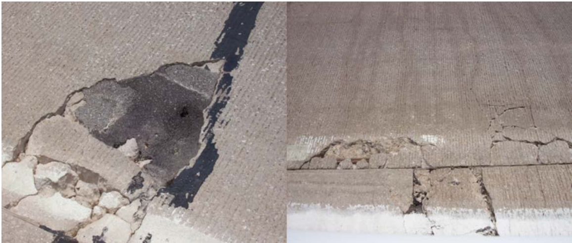
Figure A.30 (left) Y-crack breaking up, (right) distress caused by close transverse cracking
