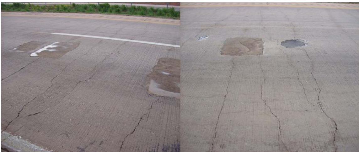
Figure A.82 Roadway patches with exposed steel
