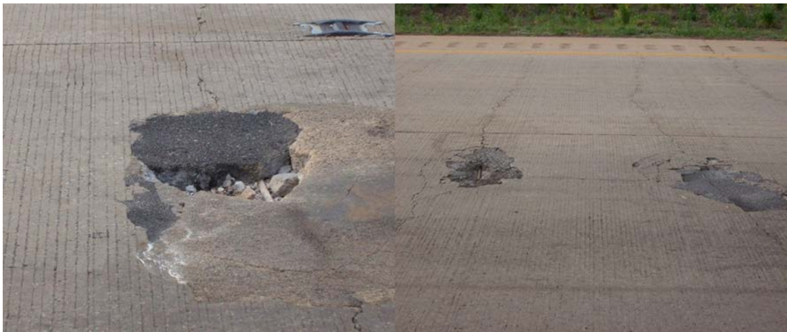
Figure A.82 Roadway patches with exposed steel
