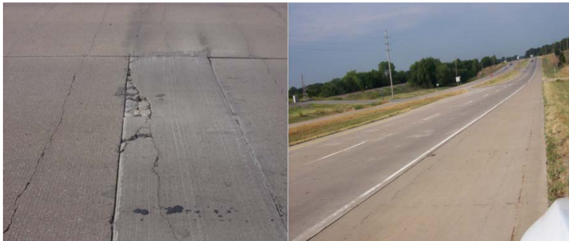
Figure A. 38 (left) patch showing signs of distress (right) area of road where crack survey was taken.
