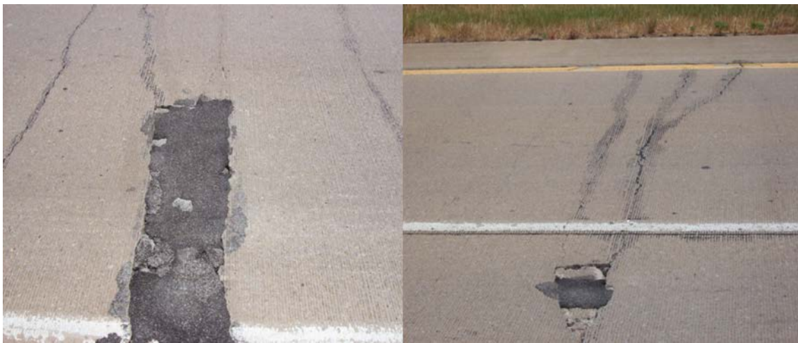
Figure A.50 Patches that appear to be the result of a failed Y-crack
