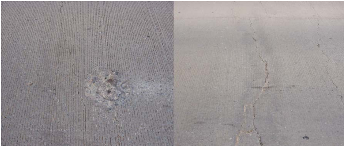
Figure A.53 (Left) Large circular distress, (right) Spalled Y-crack beginning to break up
