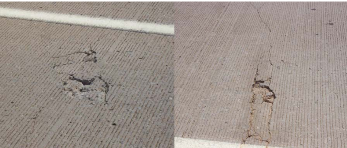
A.60 (left) Two closely spaced transverse cracks, (right) Y-crack developing into a punch-out
