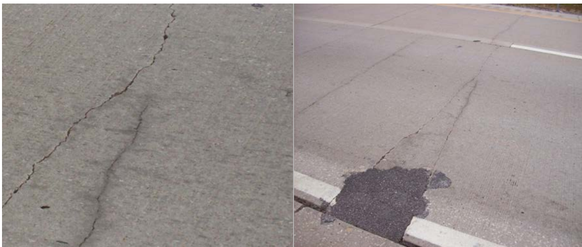
Figure A.72 A transverse crack stopping just short of a “Y” intersection with another transverse crack.
