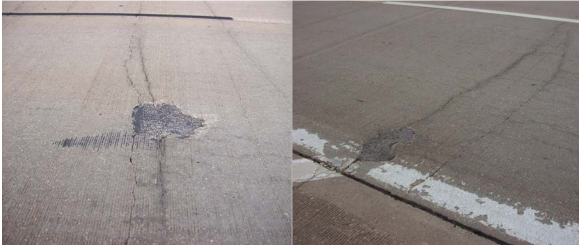
Figure A.71 Meandering cracks with small patches stopping just short of a “Y” intersection
