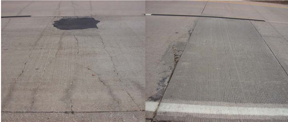
Figure A.79 (Left) Patch at construction joint, (Right) closely spaced transverse cracks with a patch
