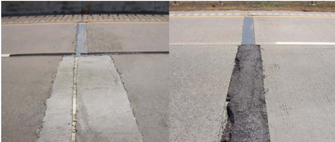
Figure A.59 Terminal joints at the beginning and end of the project
