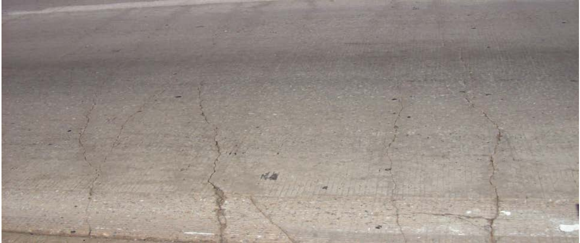
Figure A.7 Closely spaced transverse connected by longitudinal cracks
