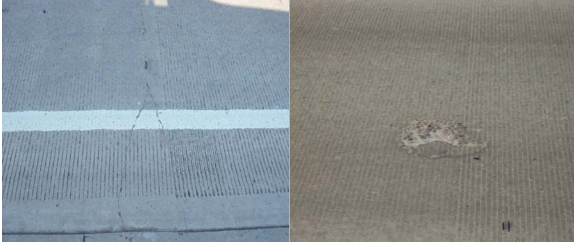
Figure A.15 (Left) Typical Y-crack for the region, (right) circular spalled area
