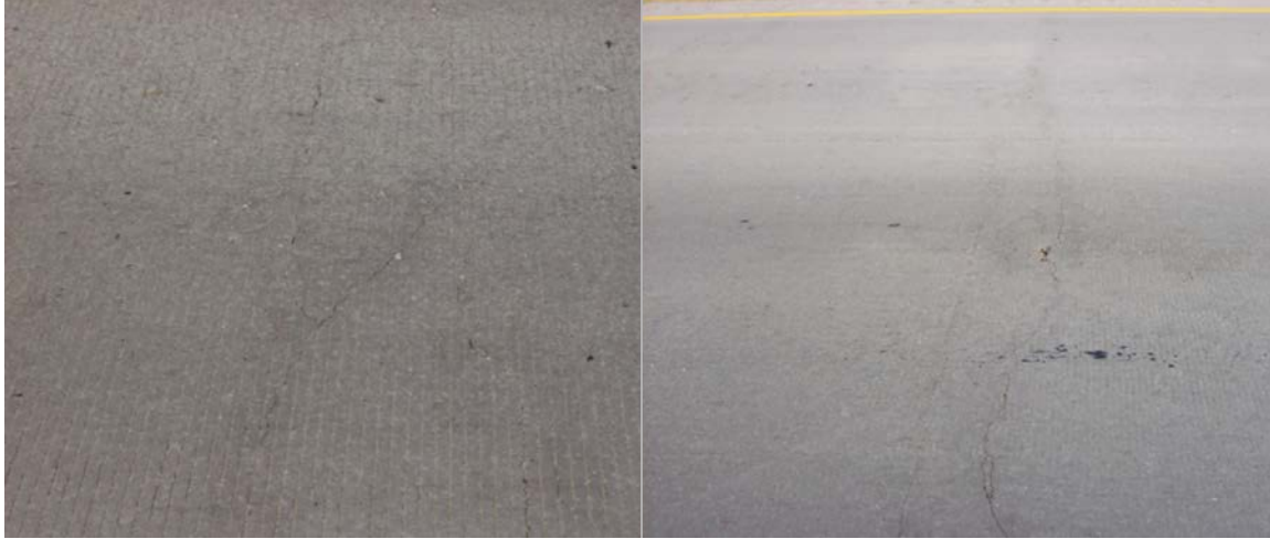
Figure A.17 (Left) Y-crack located in the region; (right) two close transverse cracks showing distress
