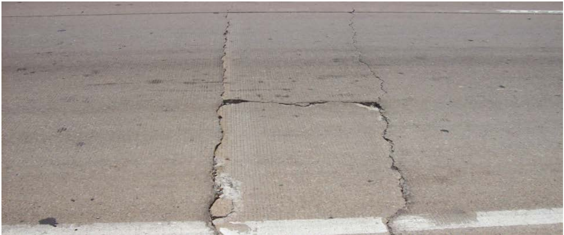
Figure A.48 Two transverse cracks intersected by a longitudinal crack
