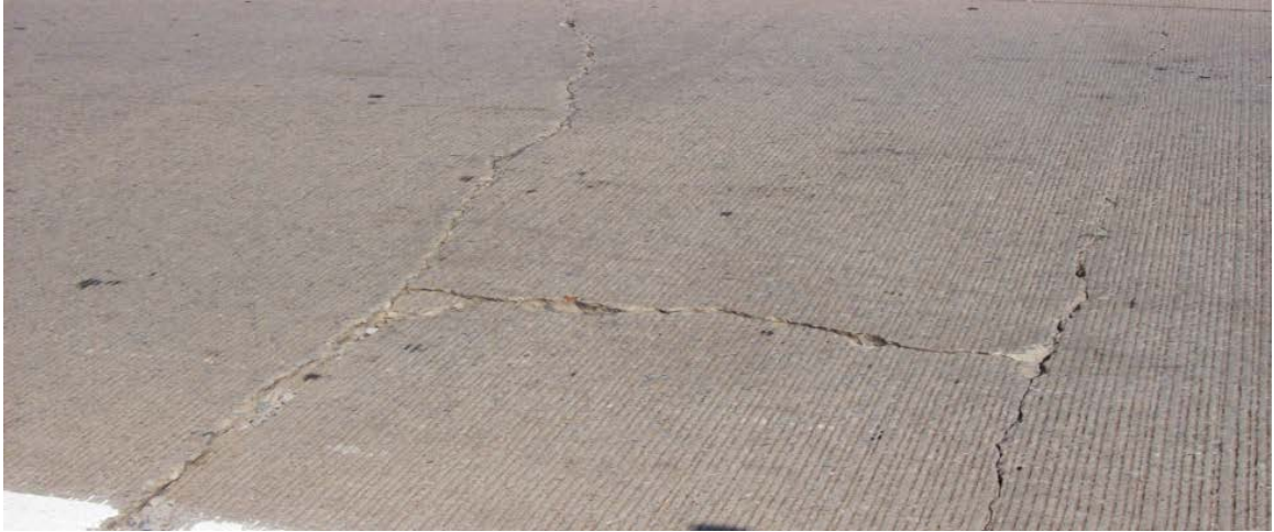
Figure A.44 Two transverse cracks intersected by a longitudinal crack
