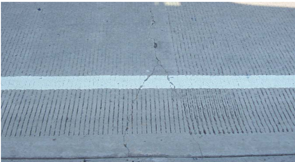
Figure 2.2 Y-cracking example
