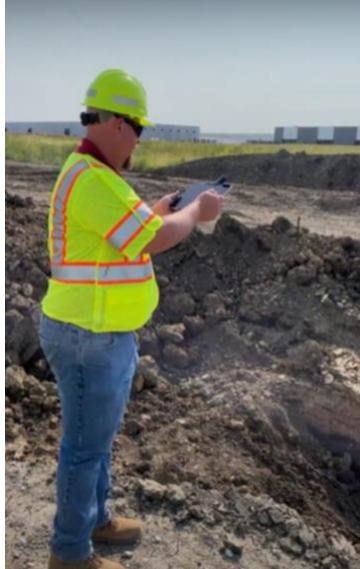
Figure 33. Utility as-built creation using Vigram viDOC
