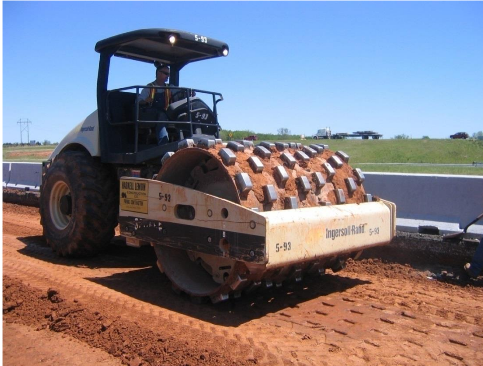
Figure 3-50 Compaction of Subgrade Soil
