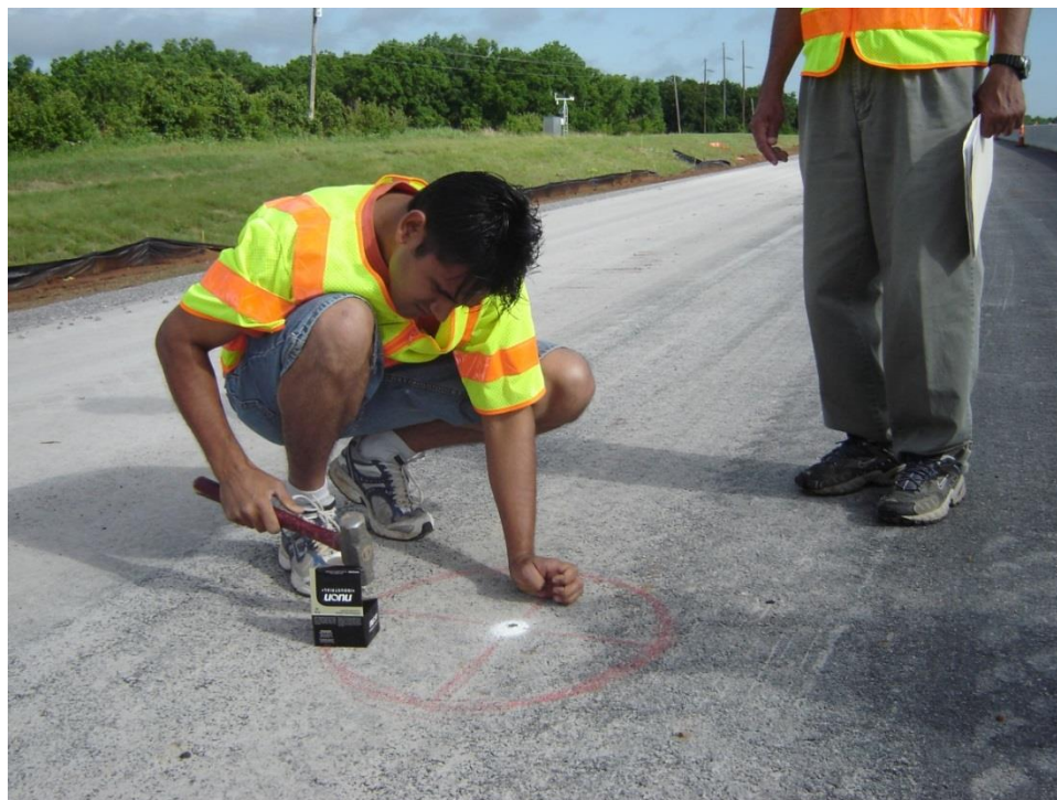
Figure 3-78 Driving Nails on the Identified Stations
