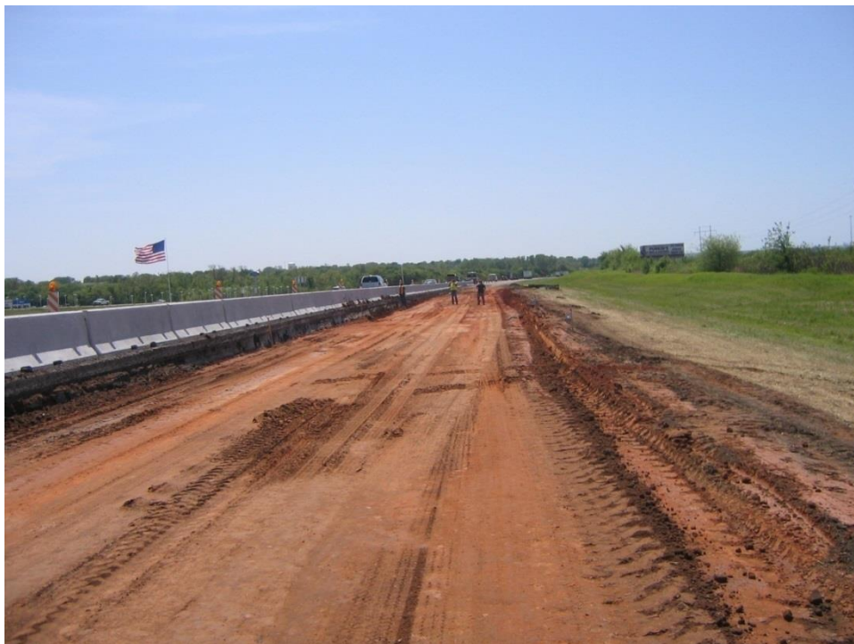
Figure 3-2 Instrumentation Site Before Construction, Looking South
