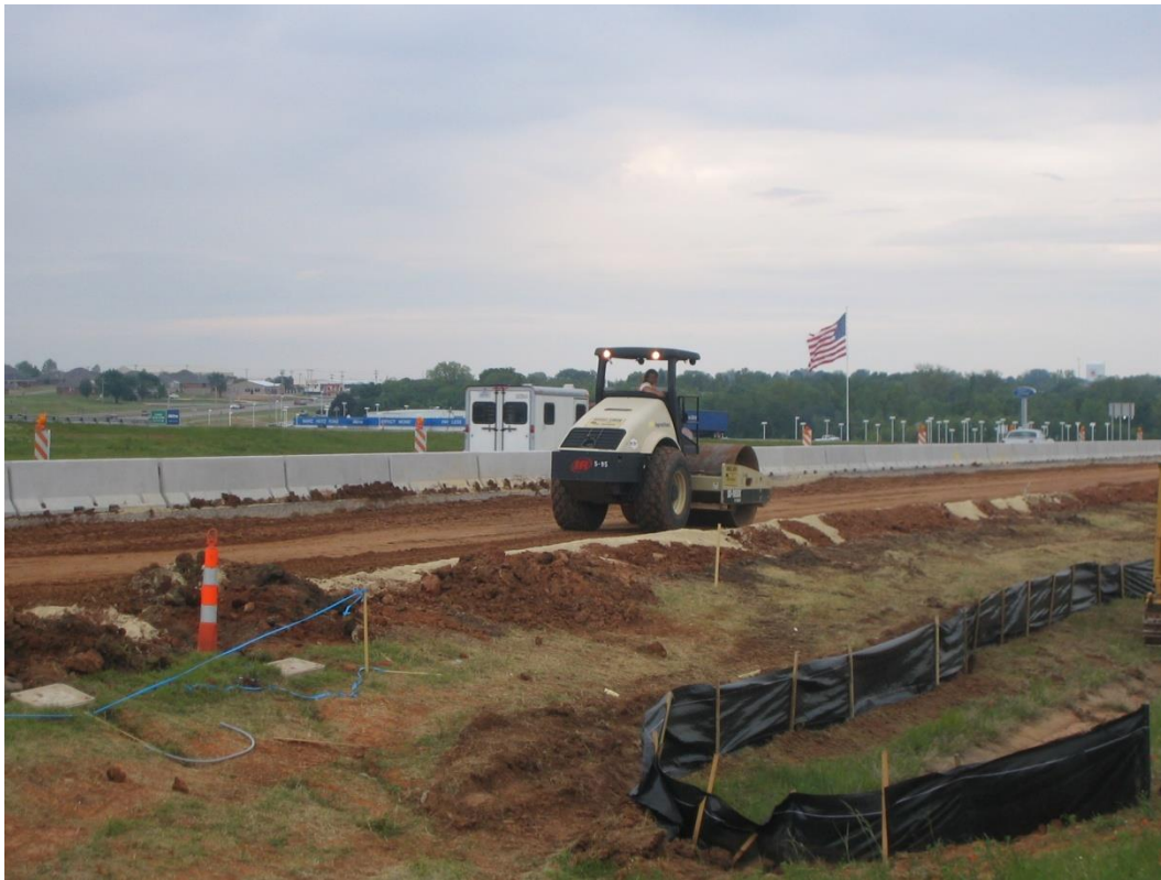
Figure 3-59 Compaction of Stabilized Subgrade Layer
