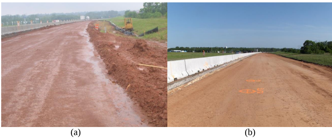
Figure 3-59 Compaction of Stabilized Subgrade Layer
