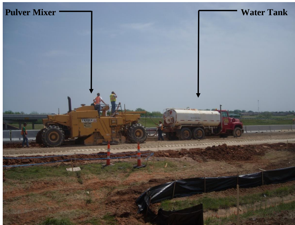
Figure 3-54 Water Tanker and Pulver Mixer Working at the Site
