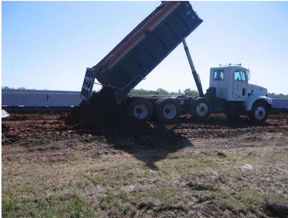
Figure 3-48 Backfilling with Imported Soil
