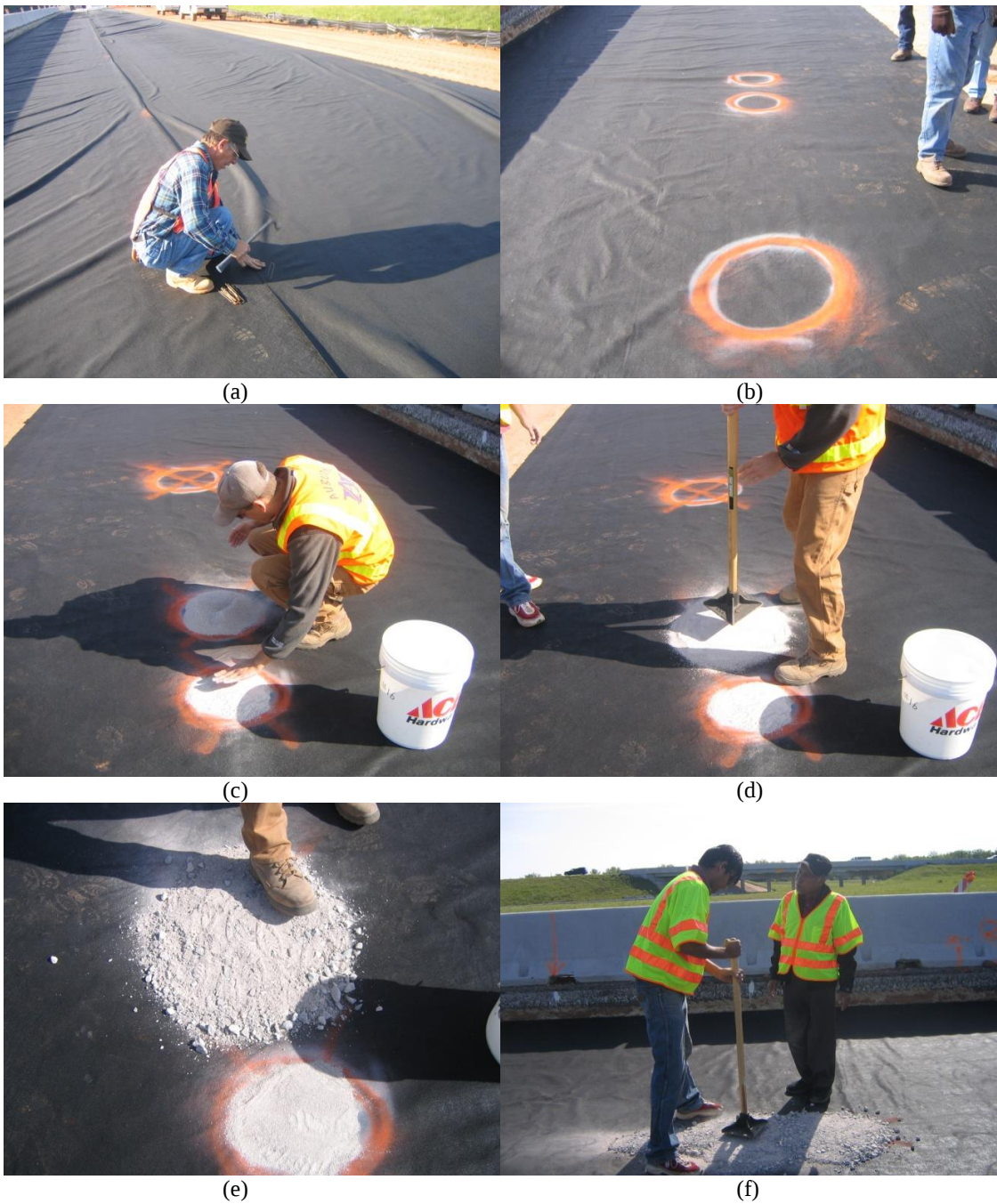
Figure 3-63 Hand Placement of Aggregate Base Material
