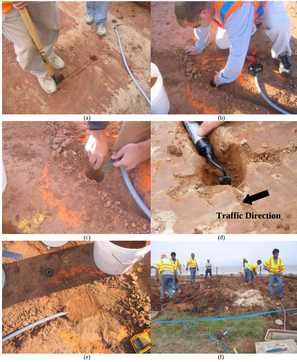
Figure 3-58 Installation of Moisture Probe on Subgrade
