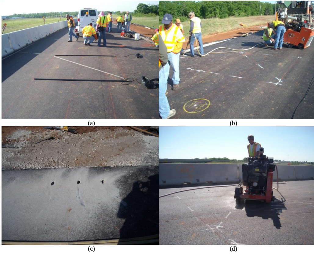
Figure 3-70 Installation of Dynax ® Axle Sensors
