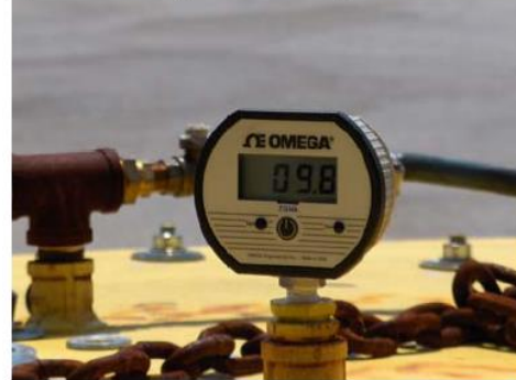
d) External Pressure Gauge on Chamber
