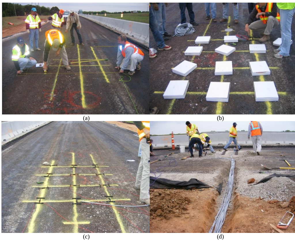
Figure 3-65 Installation of Asphalt Strain Gauges
