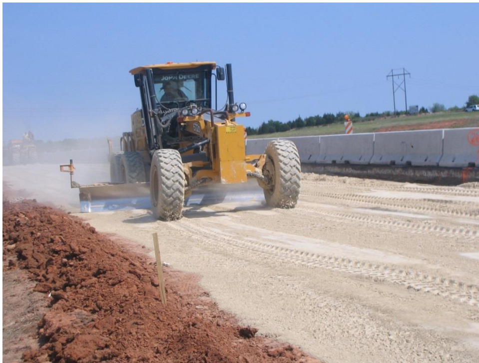
Figure 3-53 A Motor Grader Spreading CFA
