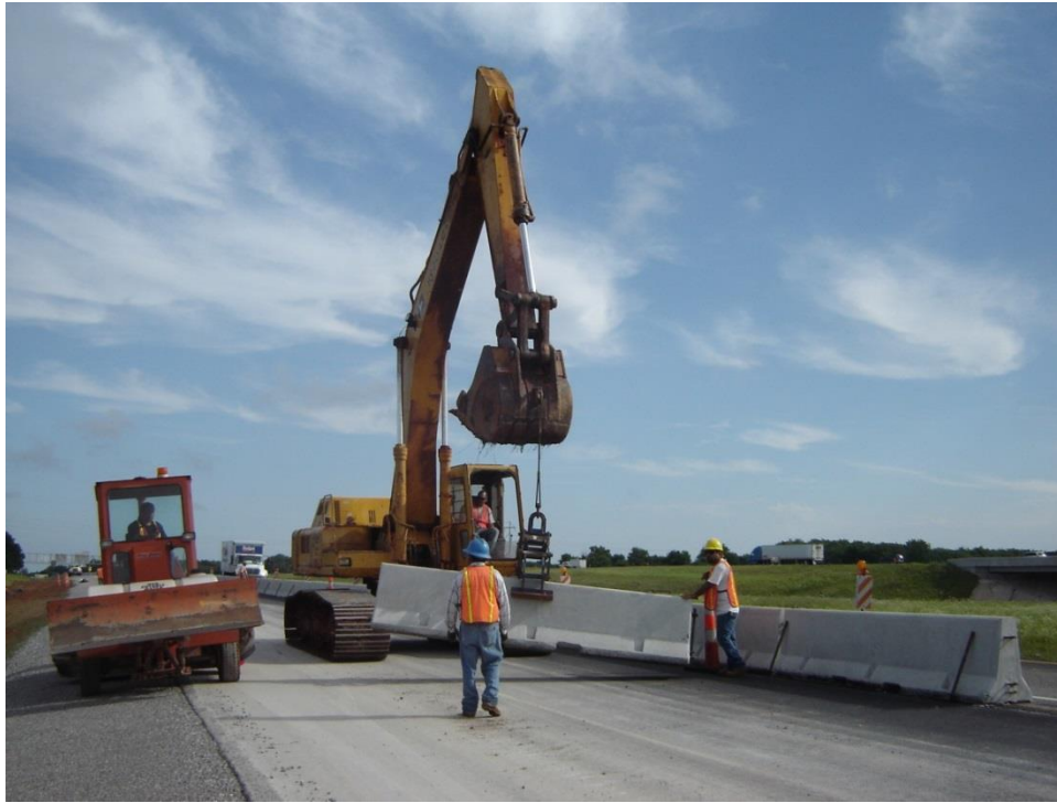
Figure 3-79 Removal of Concrete Barriers
