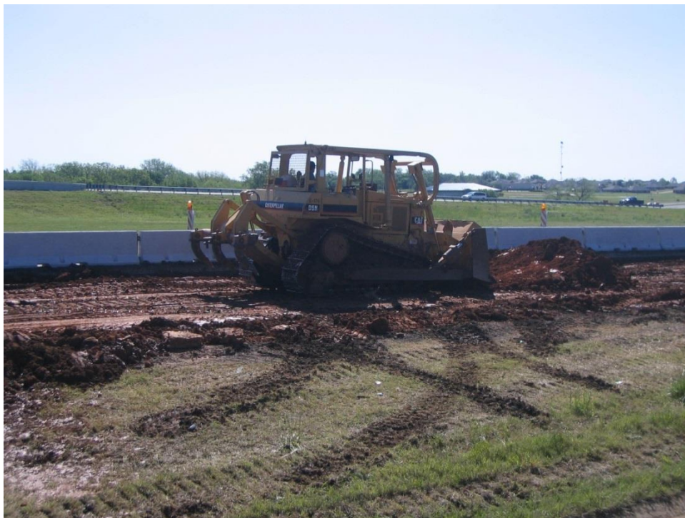
Figure 3-49 Grading of Subgrade Soil
