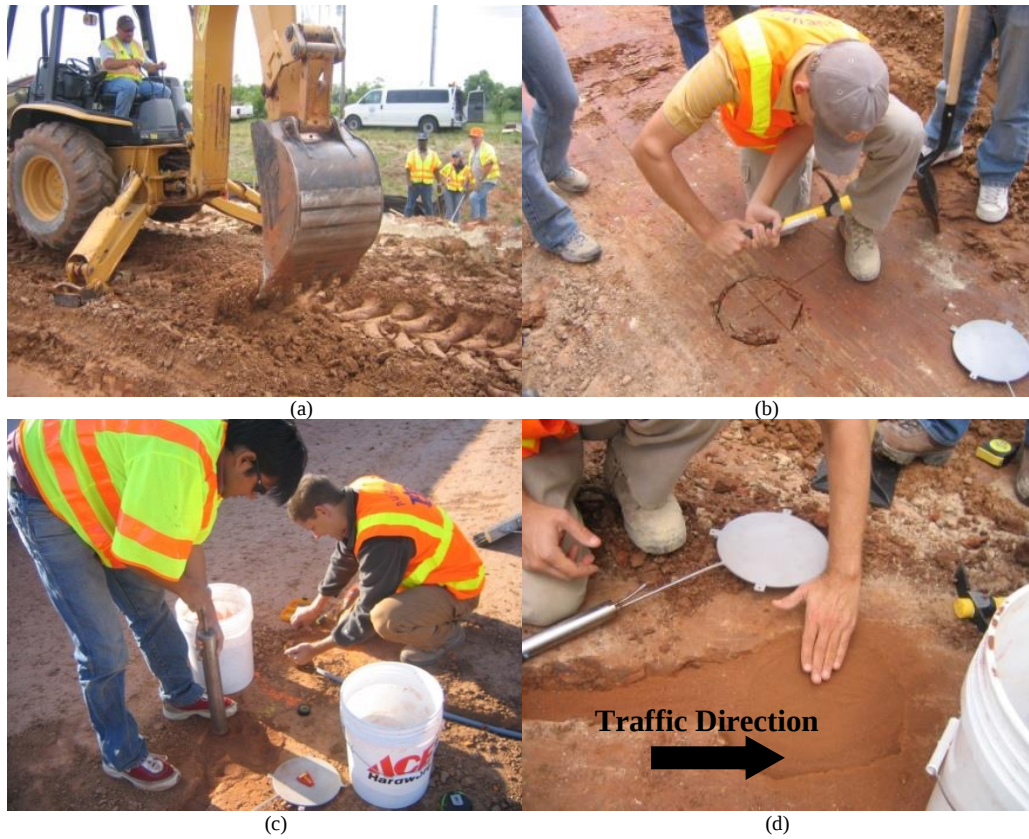
Figure 3-56 Installation of Earth Pressure Cell on Subgrade
