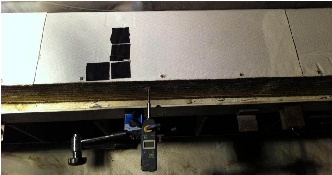
Figure 5: Plan View Of The Test Setup Showing The Holes Covered By Tape, Deflection Gauge Secured To The Beam, And Demec Points Glued On The Surface Of The Concrete
