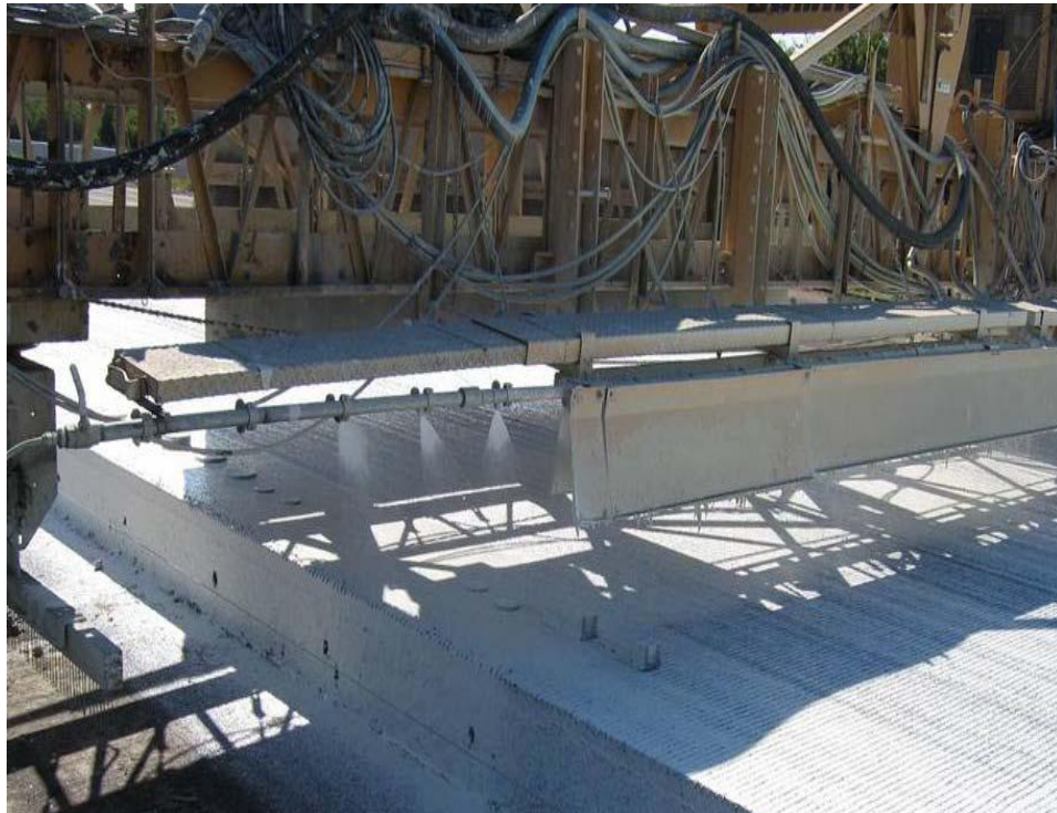
Figure 23: The Power-Driven Spray To Perform A Uniform Application On A Tinned Surface (Ye et al, TxDOT 2009)
