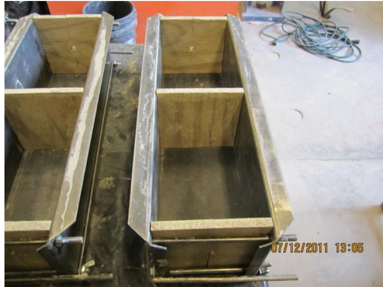
Figure 36: Assembled Formwork With Plywood Separators In Place
