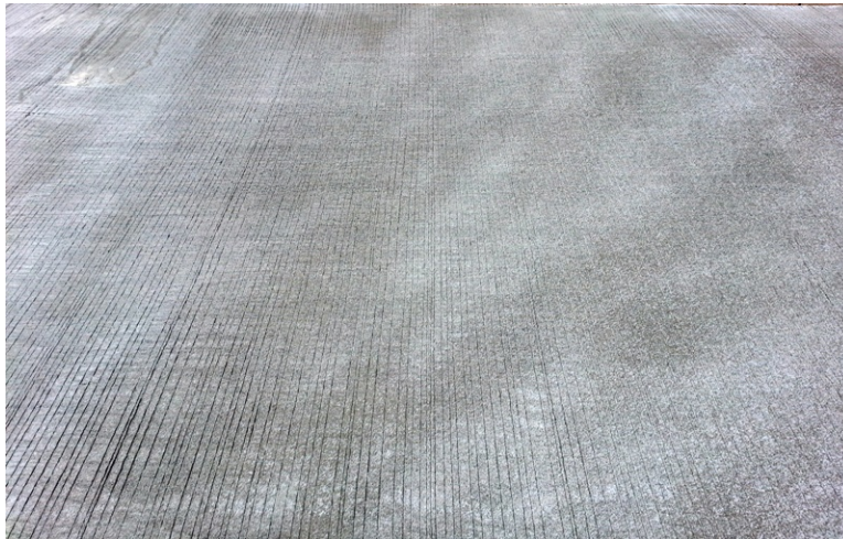
Figure 7.7 The water-wax based curing compound applied by the contractor approximately 30 minutes after paving
