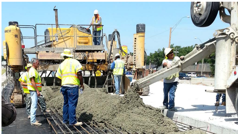
Figure 7.1 Casting the concrete pavement
