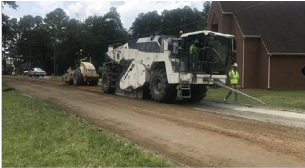
Figure 5. Conventional Full-Depth Reclamation Project on Route 216 Guinea Road in Gloucester County, Fredericksburg
