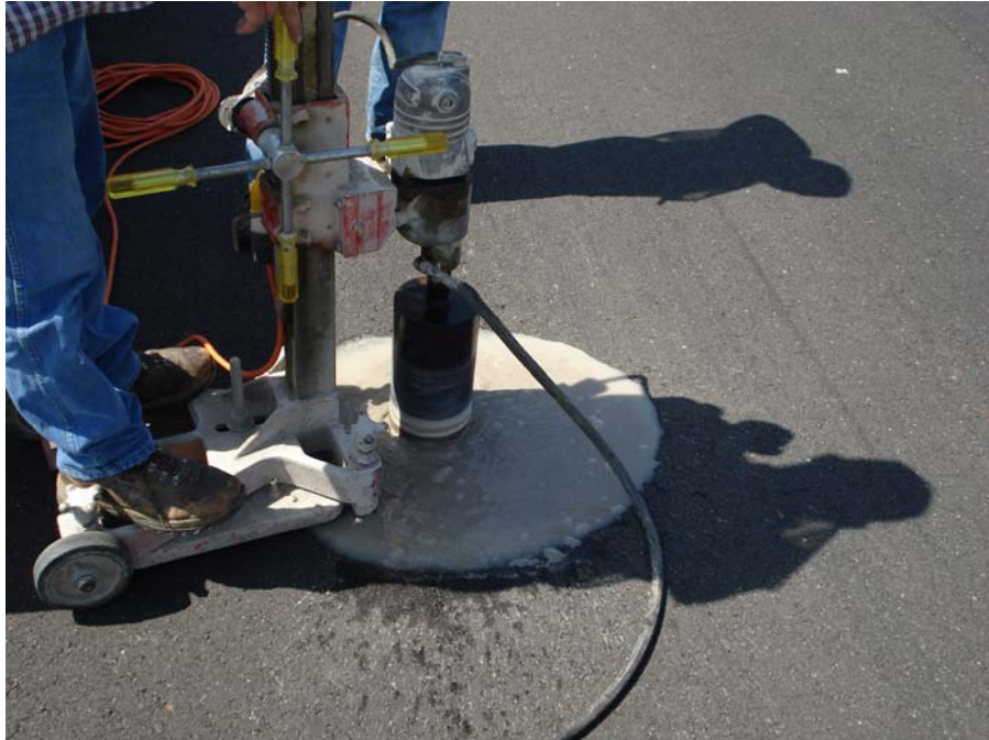
Figure 11 Obtaining field core for testing.
