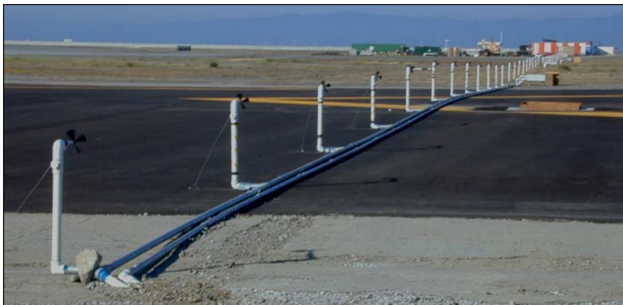
Figure 3-5. WL1 at Threshold of Runway 28L after Apron Construction
