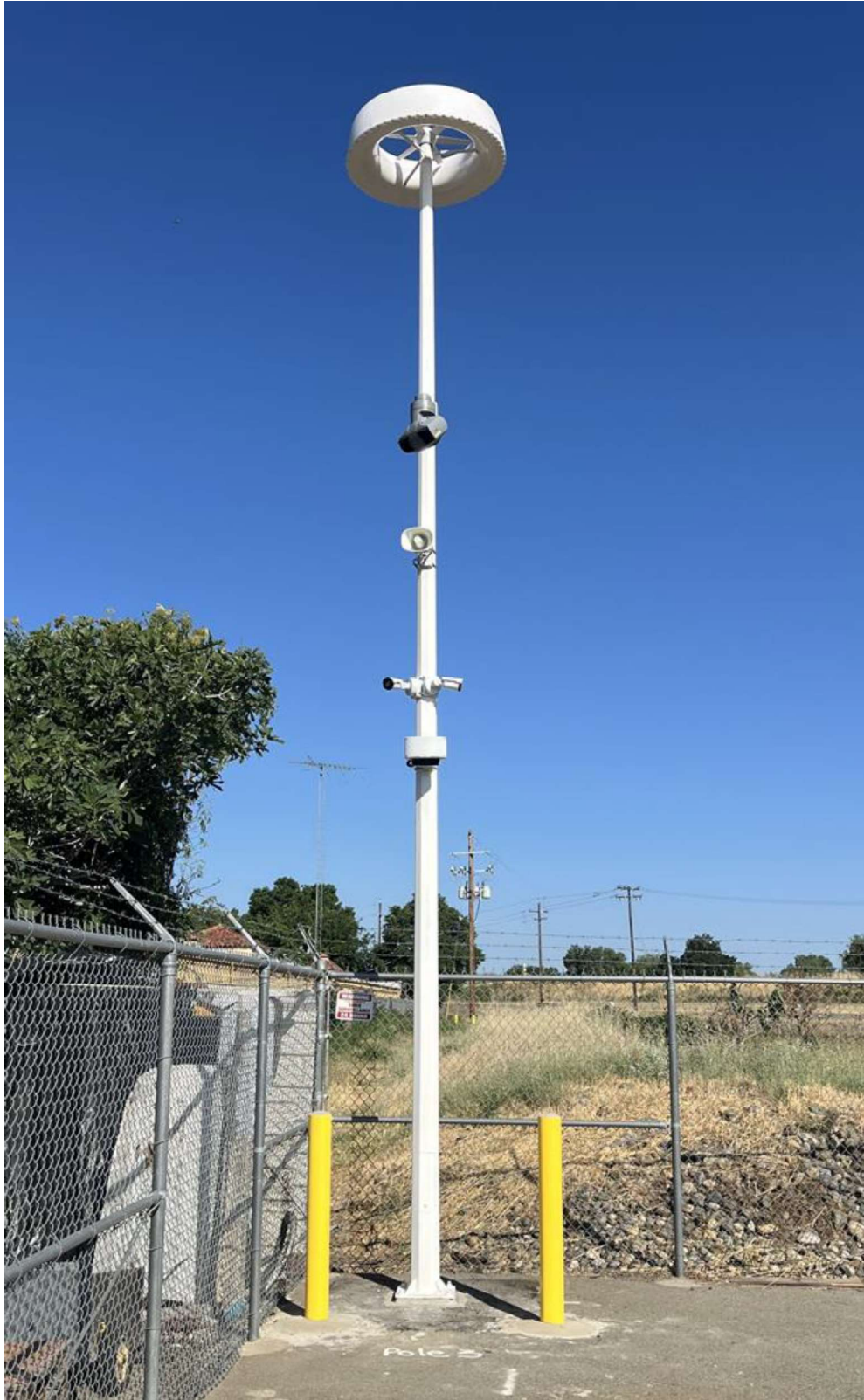
Figure B.3: Pole 3 at Marysville yard with OmniLED 07 on top in addition to one PTZ camera, two thermal cameras, one radar, and one audio horn
