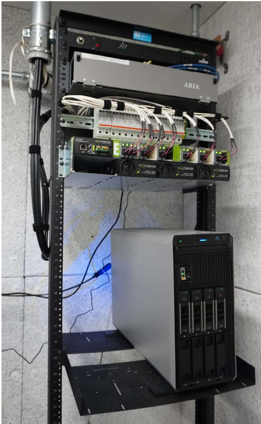
Figure B.4: AXIS VMS server and network switch inside the server room at Marysville yard
