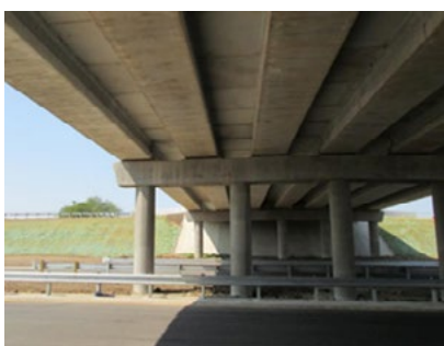
Figure 1 Texas bridge substructure
