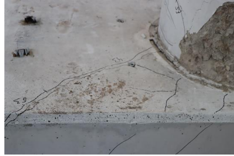
(b) Torsional cracks
