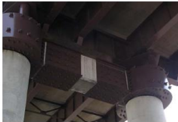
Figure 2-23. Steel jacketing application on a bent cap in Missouri (Wright et al. (2011))
