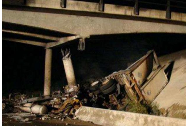
Figure 2-2. Failure of a pier located in bent cap connection caused by truck impact in Colorado (Gallegos and McPhee, 2007)
