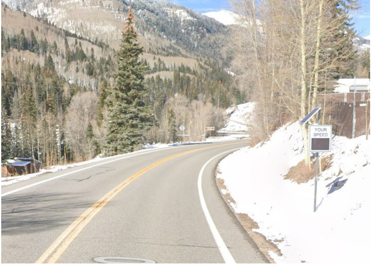
Figure 4-144: Dynamic Speed Warning Approaching MP 51 US550 SB, Nov. 2024
