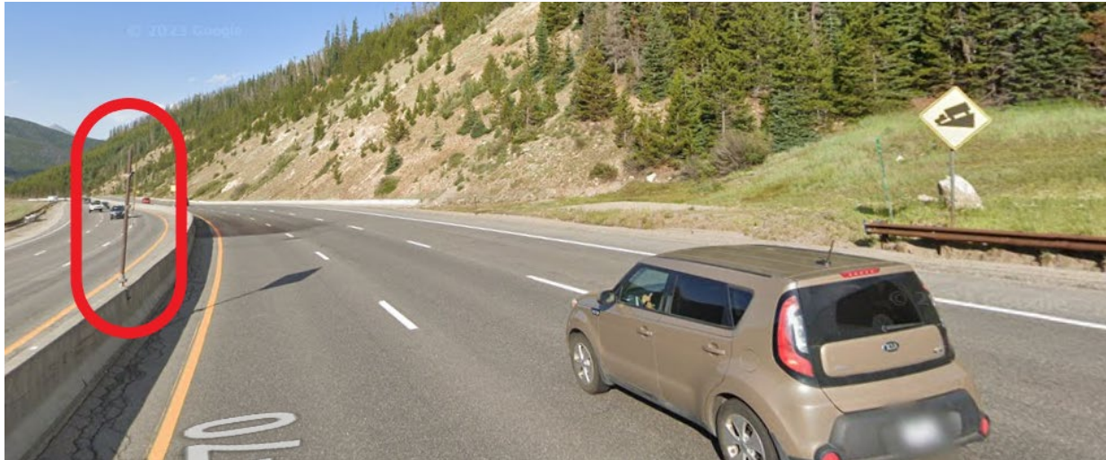
Figure 4-86: W7-1 Sign Twisted, WB I-70 MP 211.57, Aug. 2023 (facing West)
