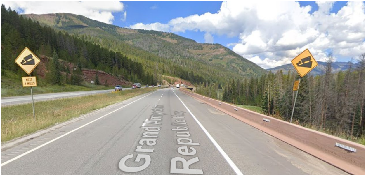
Figure 4-68: Grade Warning with Supplementary Plaque, MP 184.15, Aug. 2022
