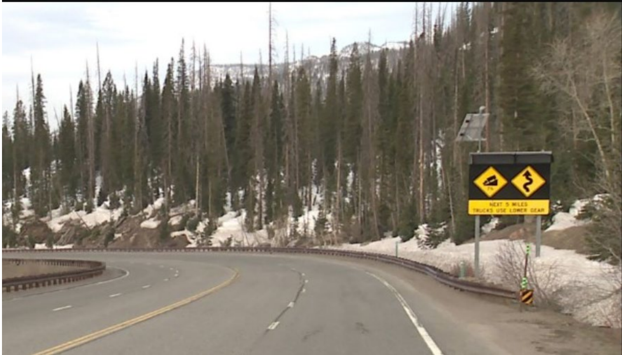
Figure 3-3: Enhanced Grade & Curve Warning Sign with Blank-Outs, Approx. MP 163.39 (OTIS 2022)
