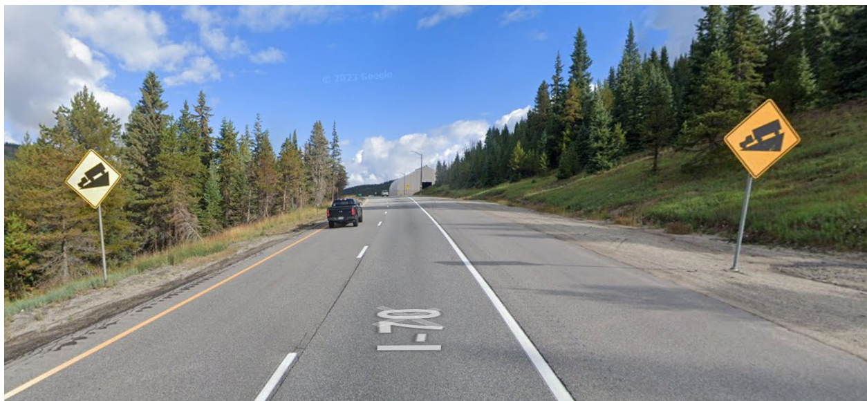
Figure 4-60: Gated Grade Warning for Trucks, MP 189.49
