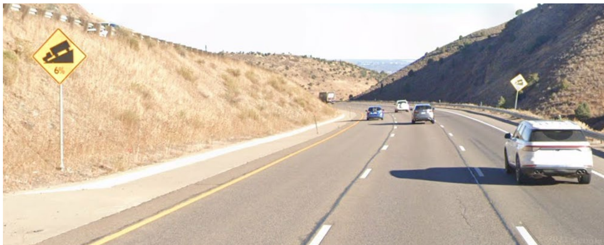
Figure 4-119: Staggered Gated Grade Warnings, MP 257.71, Oct. 2021
