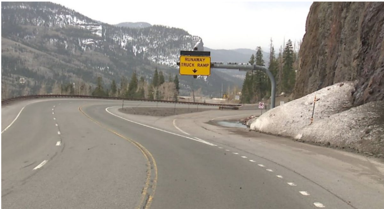
Figure 3-10: 2nd WB Escape Ramp with Enhanced Guidance, Approx. MP 160.87 (OTIS 2022)
