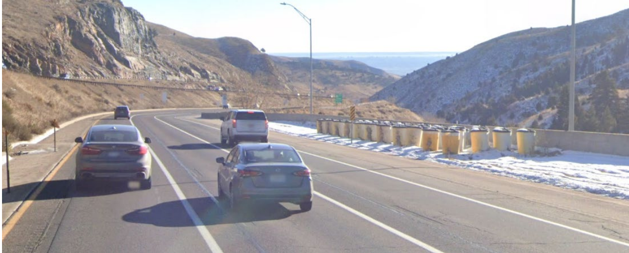
Figure 4-125: Impact Attenuators at end of Escape Ramp
