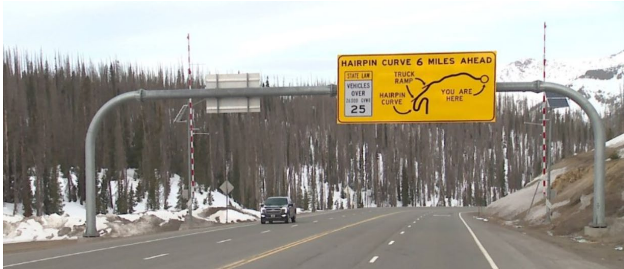
Figure 4-3: Diagrammatic Warning Sign, MP 166.60 US160
