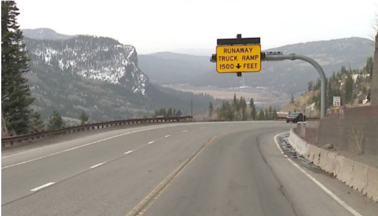
Figure 3-9: 2nd WB Escape Ramp Warning Sign Enhanced with Blank-Outs, Approx. MP 161.18 (OTIS 2022)
