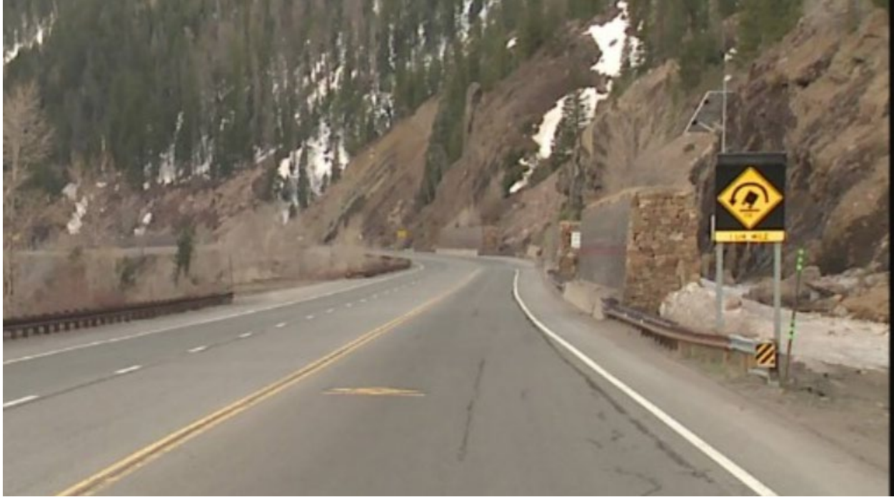
Figure 3-7: Enhanced Overturning Warning Sign with Blank-Outs, Approx. MP 161.82 (OTIS 2022)
