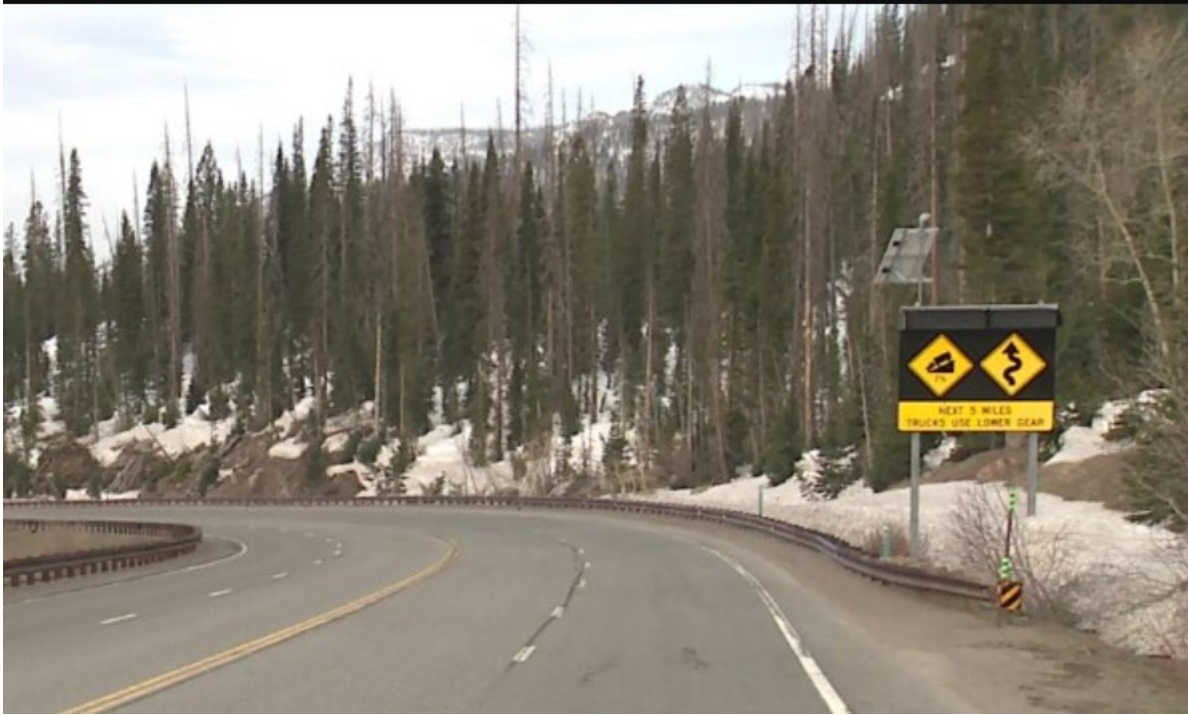
Figure 4-1: Dynamic Warning Sign with Blank-Outs, MP 163.39 US160
