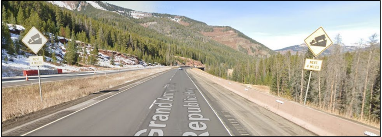
Figure 4-67: Grade Warning with Supplementary Plaque, MP 184.15, Oct. 2021
