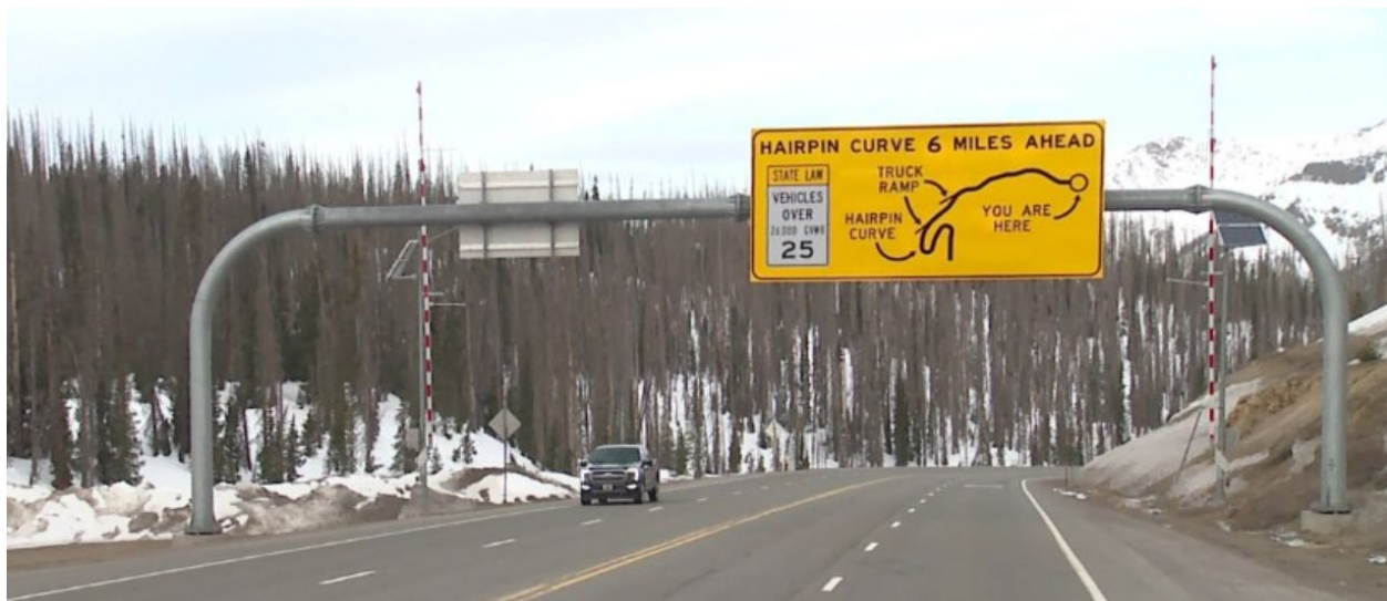
Figure 3-2: 1st WB Diagrammatic Warning Sign, Approx. MP 166.60 (OTIS 2022)
