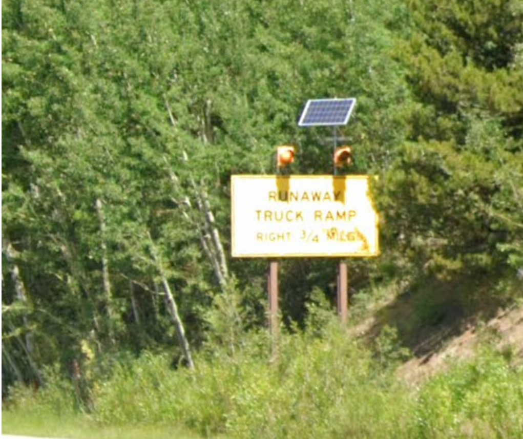
Figure 4-26: Advance Warning MP 143.08, Partial Foliage Obstruction, Jul. 2023
