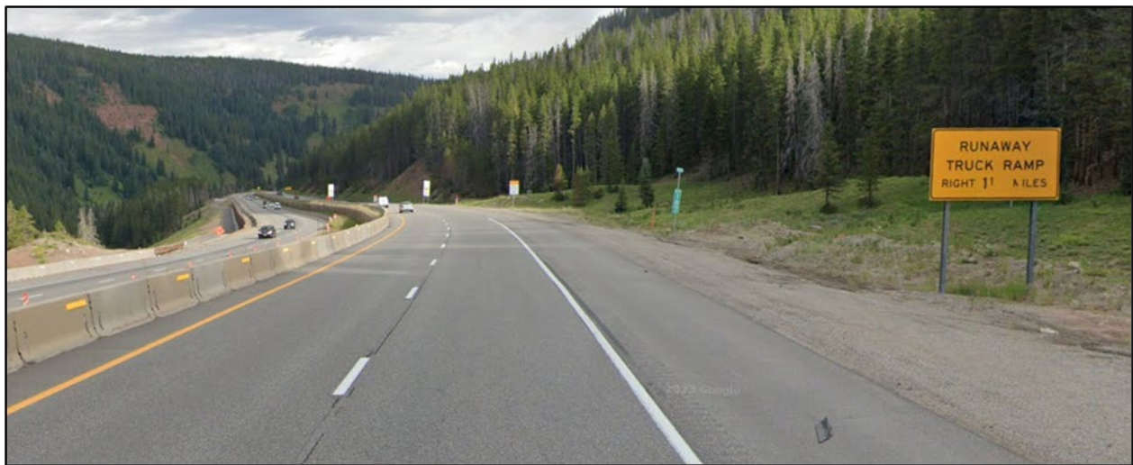
Figure 4-64: Upper Escape Ramp Advance Warning MP 187.11 (Faded), Aug. 2023
