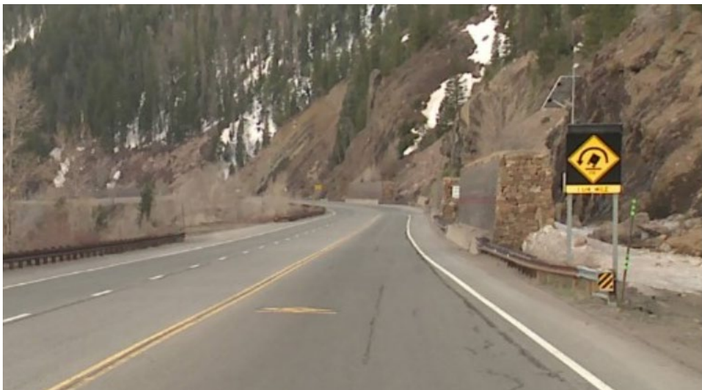
Figure 4-2: Dynamic Overturning Warning Sign, MP 161.82 US160
