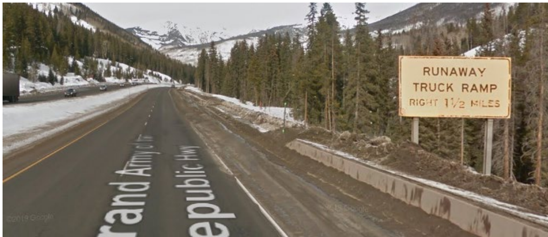
Figure 4-51: WB I-70 MP 183.72 Escape Ramp Advance Warning (Faded), Dec. 2018
