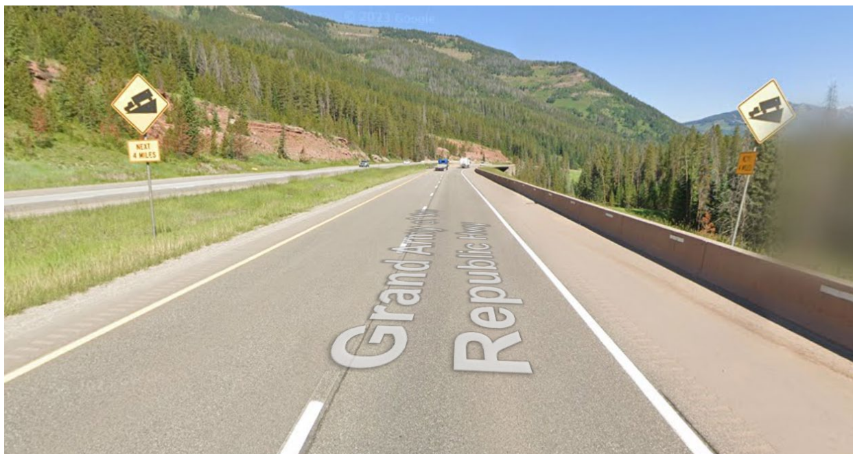
Figure 4-69: Grade Warning with Supplementary Plaque, MP 184.15, Jul. 2023
