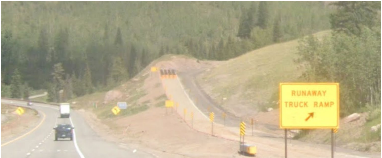
Figure 4-56: Lower Truck Escape Ramp, Aug. 2022
