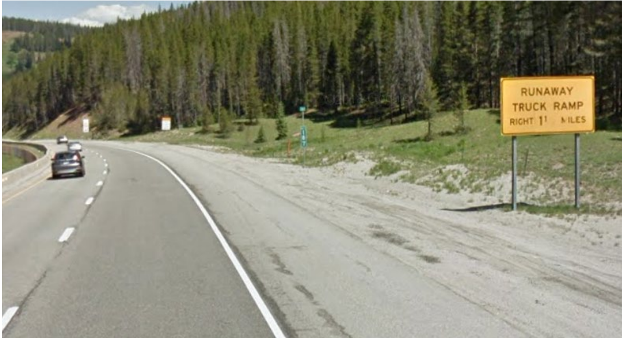
Figure 4-63: Upper Escape Ramp Advance Warning MP 187.11 (Faded), Jun. 2018
