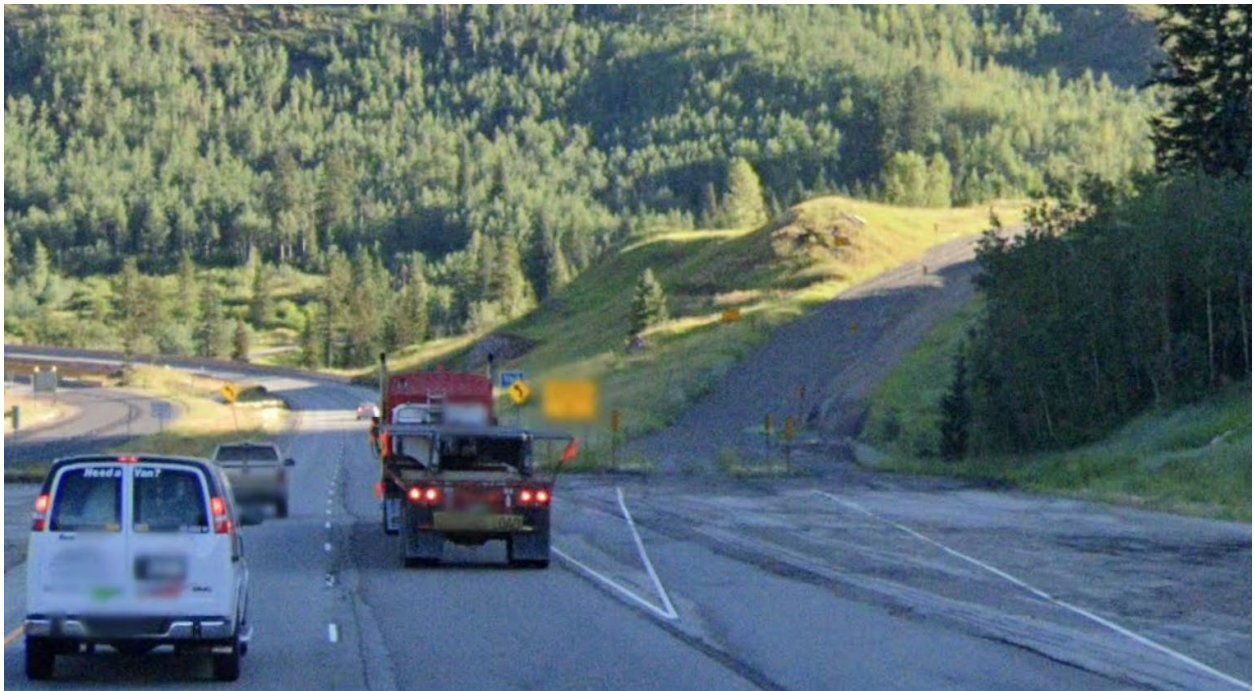
Figure 4-54: Lower Truck Escape Ramp (MP 182.36), Aug. 2019
