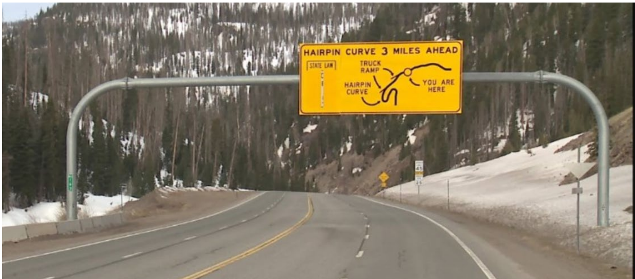
Figure 3-4: 2nd WB Diagrammatic Warning Sign, Approx. MP 163 (OTIS 2022)
