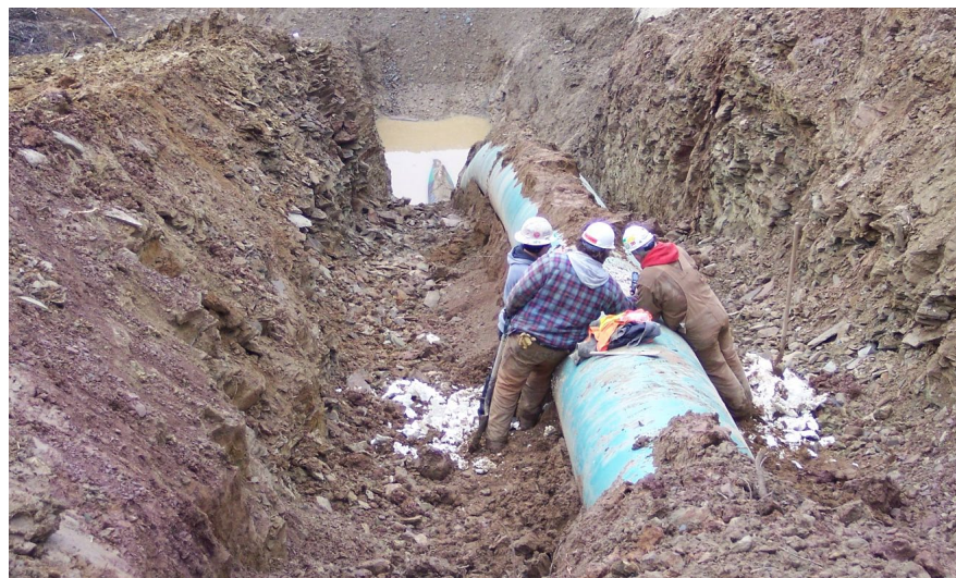
Workers near excavated pipeline
