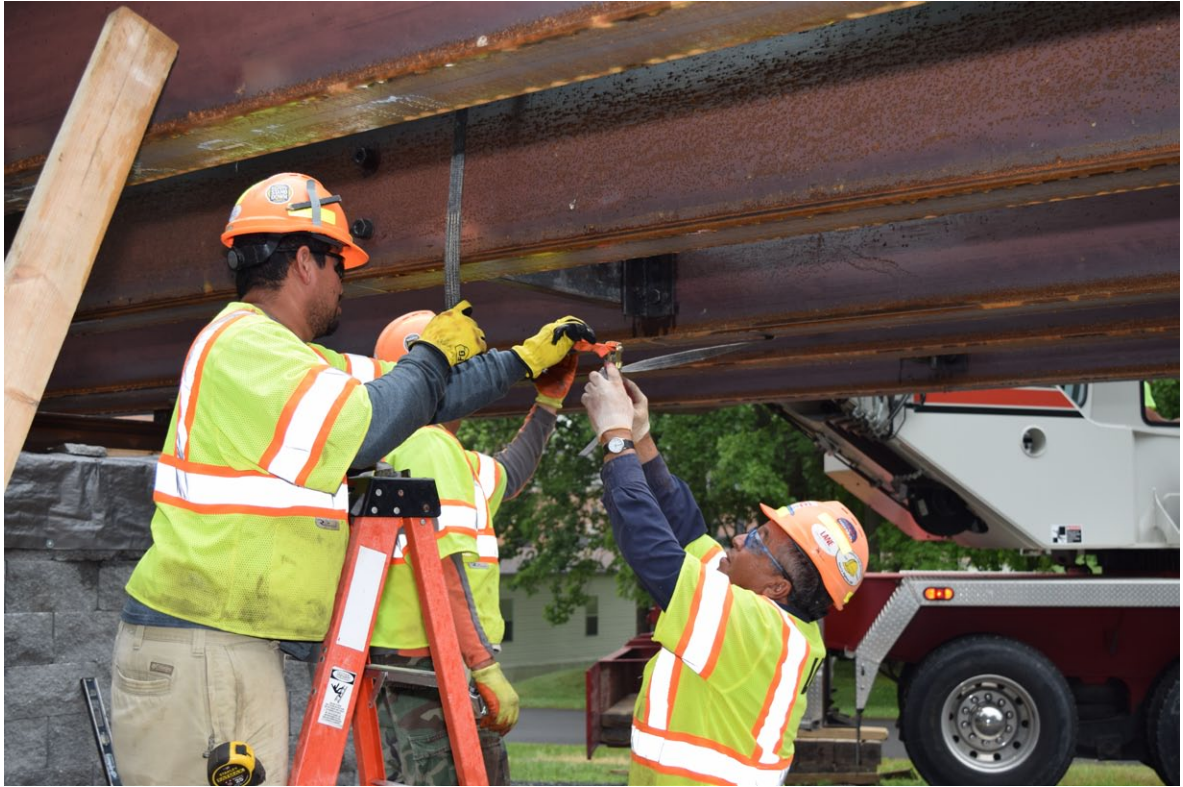
Workers prepare to transport bridge components
