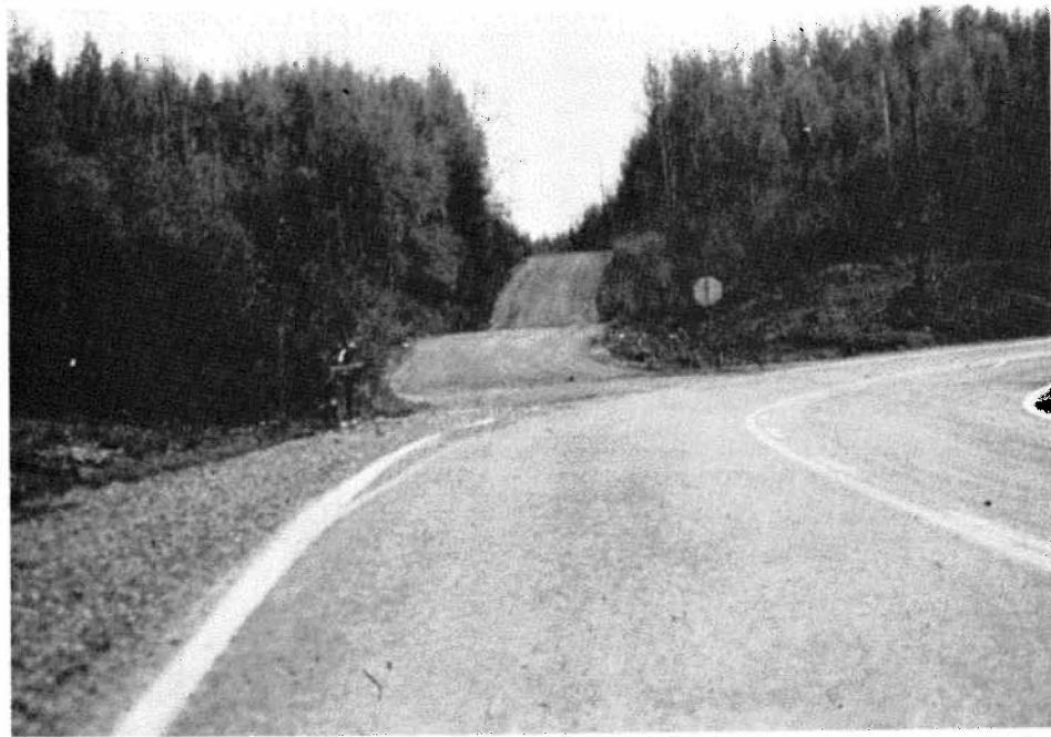
Figure 15. Tangential Road at Point of Curve e
