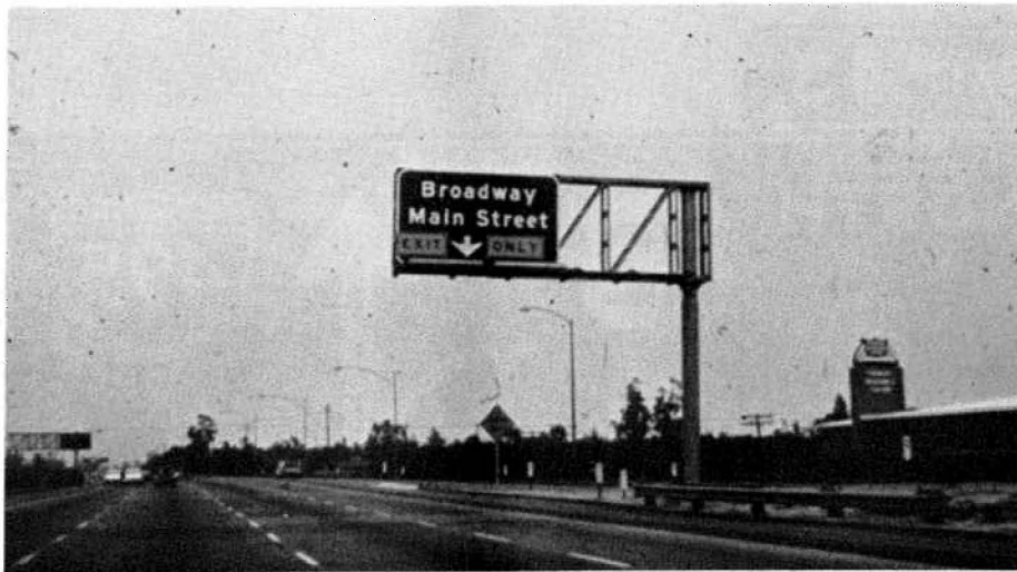
Figure 10. Interchange Lane Drop "EXIT ONLY" Treatment
