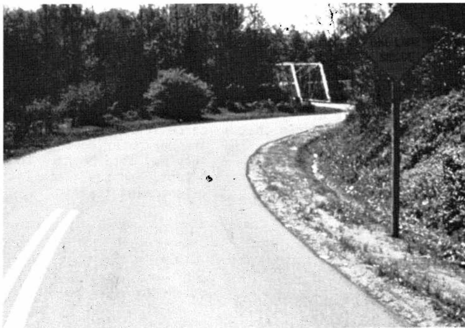
Figure 23. Narrow Bridge on Curve
