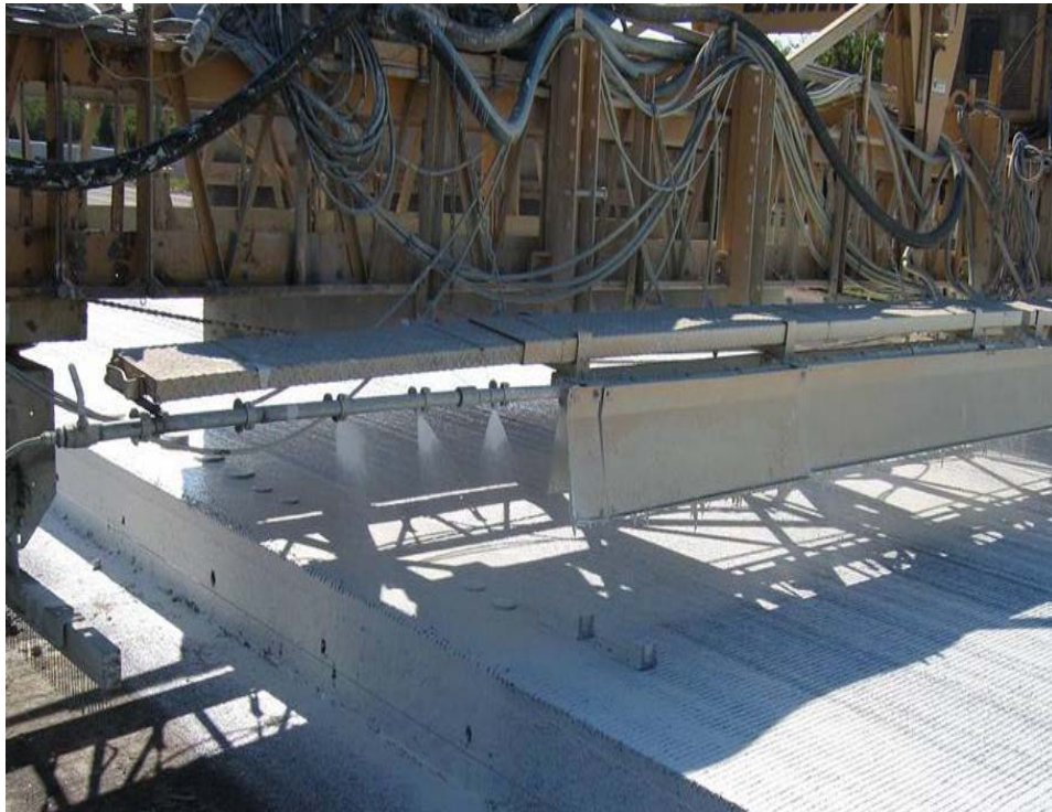
Figure 5.23 The power-driven spray to perform a uniform application on a tinned surface (Ye et al, TxDOT 2009)
