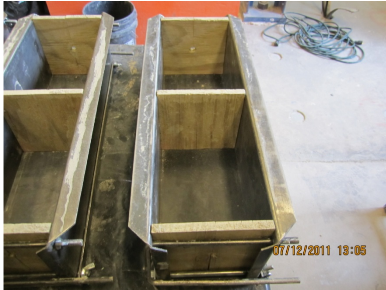
Figure 5.36 Assembled formwork with plywood separators in place
