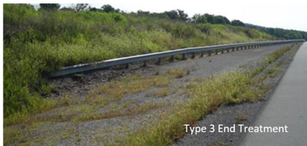
Figure A11: Preferred Guardrail End Treatments
