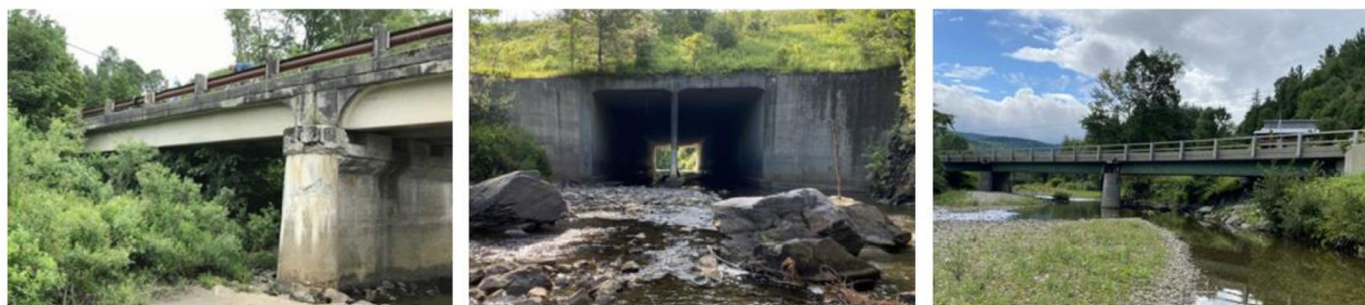
Figure 21: Examples of selected optimal representative bridges of concrete tee-beam (left), concrete culvert (middle), and short-span steel (right) bridges
