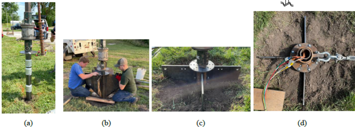
Figure 4. Collar Vane installation sequence for CV2-type vanes. a.) Helical pile and lead sections are installed by a conventional torque motor. b.) Two collar vane sections are connected via bolts around the central shaft, but are not yet connected via flanges. c.) Helical pile installation continues and contact between the flanges pulls the collar vane into the ground without rotating. d.) The Collar Vane and helical pile are structurally connected via bolts through the flanges.
