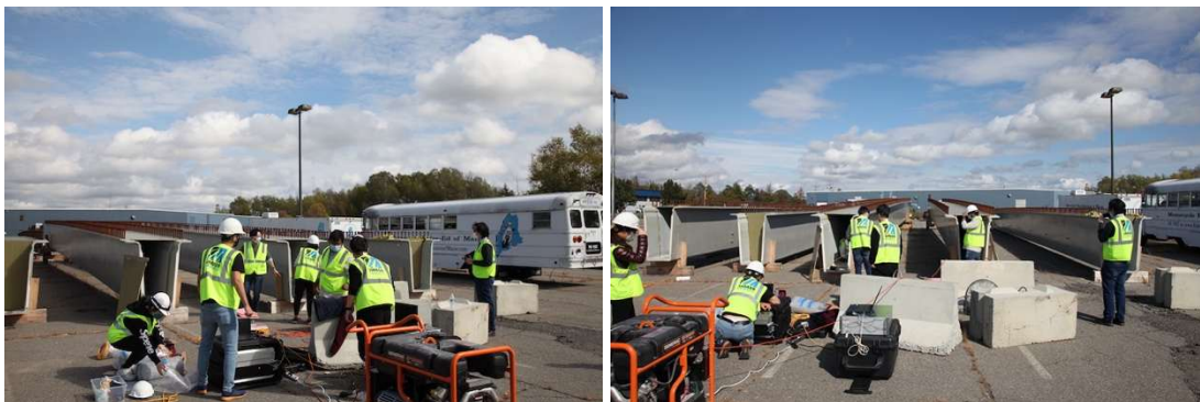
Figure 7. Installation of sensing textiles on three composite bridge girders (10/06/2020)
