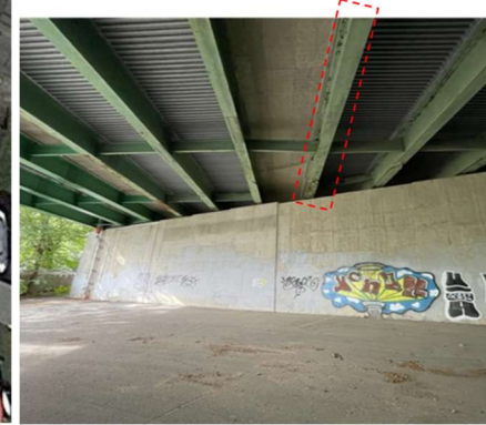
(b) Top-view of twenty-two girders of the bridge. (c) Selected steel girder.
