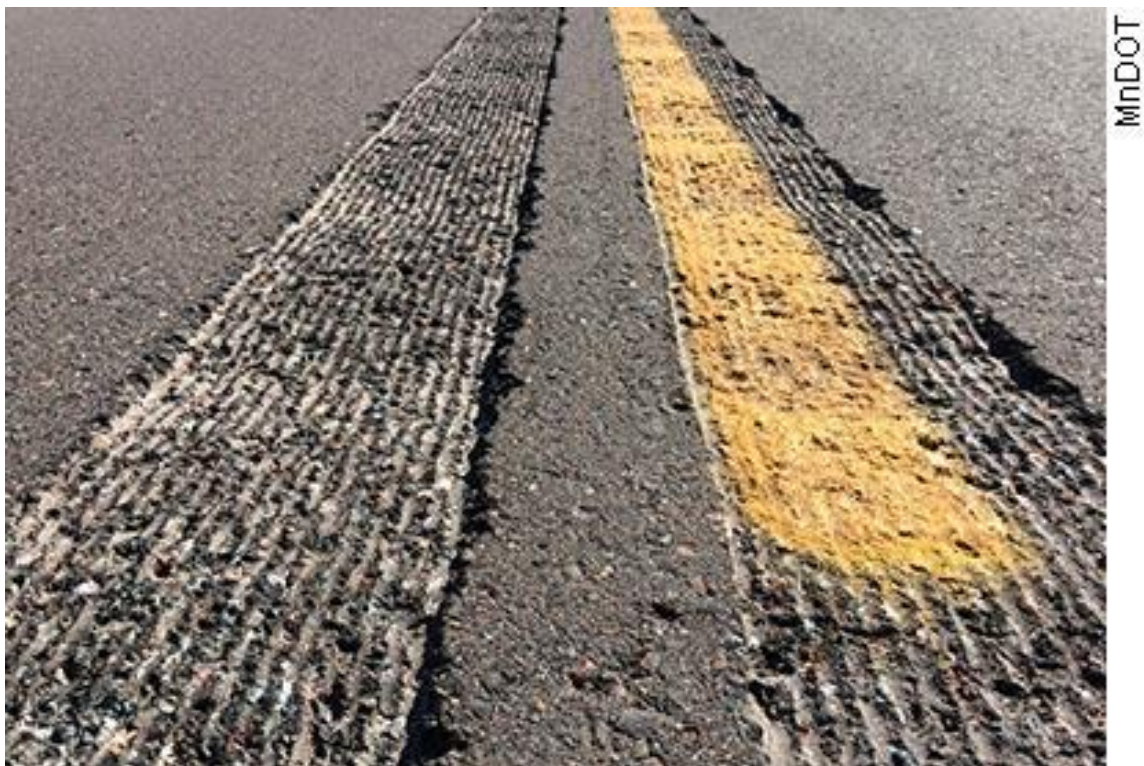
Figure 10. Photo. Sinusoidal Rumble Strip (16)
