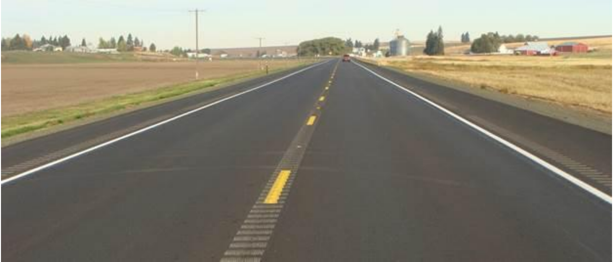
Figure 4. Photo. Centerline Rumble Strips (8)
