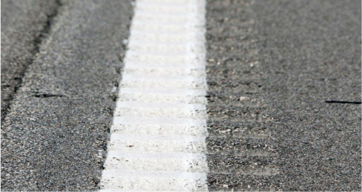
Figure 3. Photo. Edge line Rumble Strips (6)
