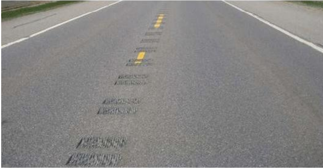
Figure 9. Photo. Alternating (Segmented) Rumble Strip (15)
