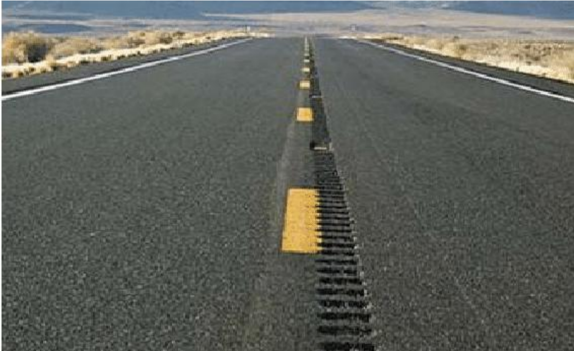
Figure 8. Photo. Continuous Rumble Strip (15)
