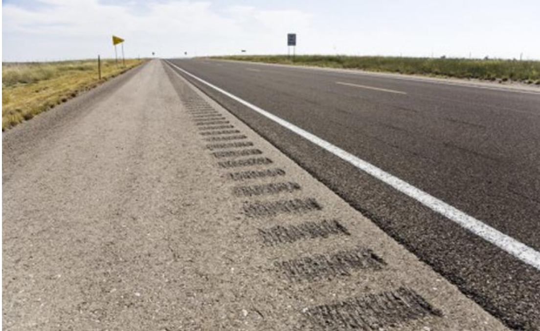
Figure 2. Photo. Shoulder Rumble Strips (4)
