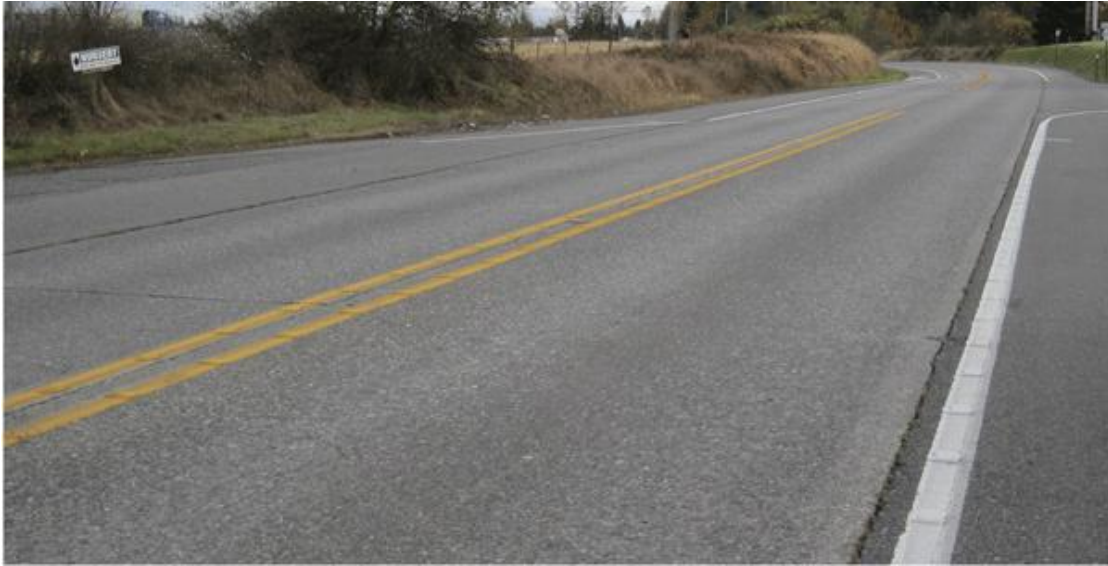
Figure 5. Photo. Plastic Raised Rumble Strip (11)
