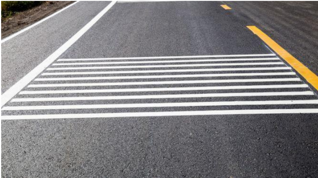
Figure 1. Photo. In Lane Rumble Strips (2)
