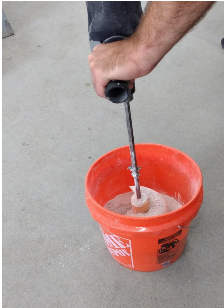
Figure 2.1: Mixing material in a 5-gallon bucket and drill-mounted mixer
