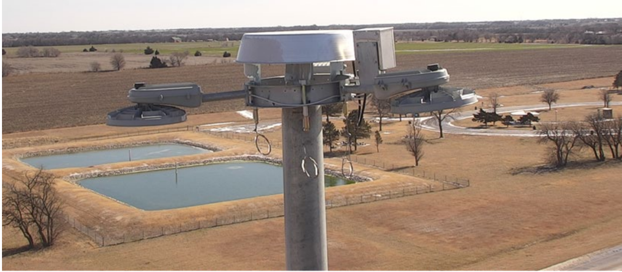
Figure 1.1: High Mast Illumination Pole Lighting Assembly with LED Luminaires (K. Peterson [KDOT], personal communication, March 13, 2019)
