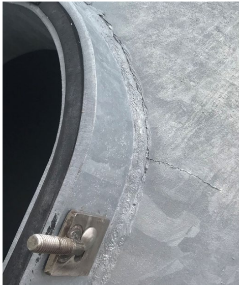
Figure 1.2: Cracking Observed at the Handhole Weld (K. Peterson [KDOT], personal communication, March 13, 2019)
