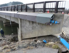
Settlement of backfill behind the abutment
