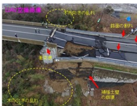
Failure of reinforced soil wall
