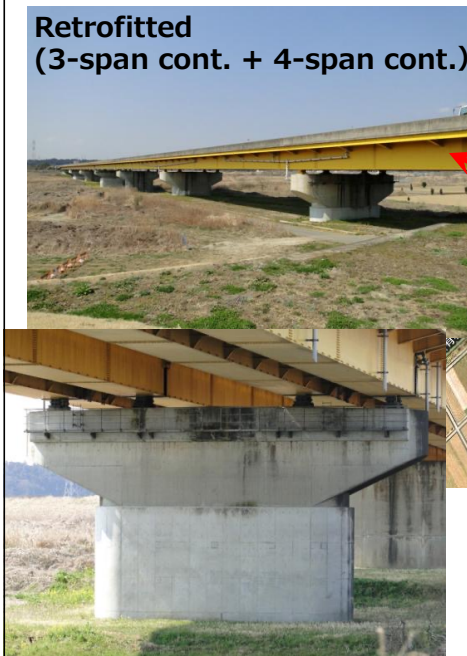
No Damage to Piers and Bearings
