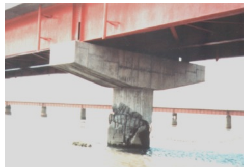
Damage to low-stiffness areas like RC bridge piers or bearing area
