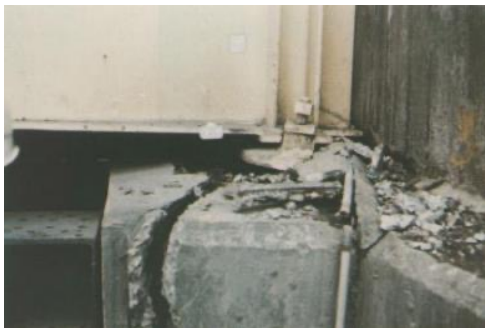
Damage to low-stiffness areas like RC bridge piers or bearing area
