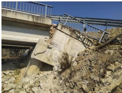
Liquefaction induced failure of abutment piles in 2023 Turkey Earthquake
