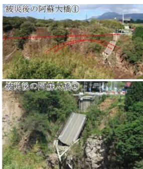
Collapse of Aso Bridge
