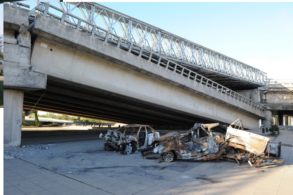
Temporary bridging installed in Chile after 2010 Maule EQ
