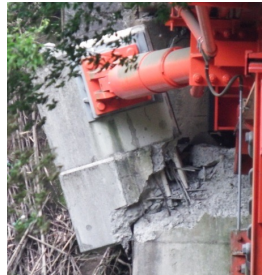
Photo-3 Failure of Attachment of Damping Device
