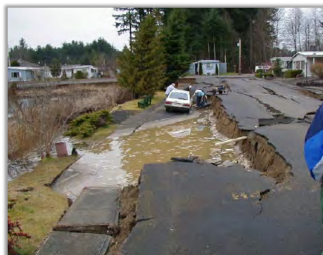
Liquefaction Example 2001 Nisqually Earthquake
