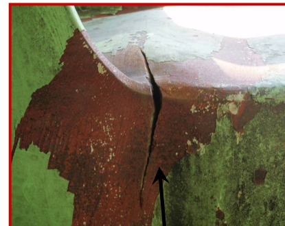
Slight Buckling and Crack Observed in Lower Chord Member
