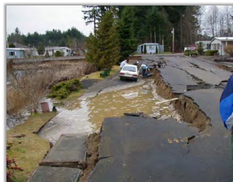
Liquefaction Example 2001 Nisqually Earthquake
