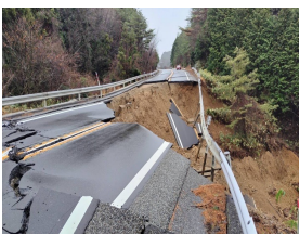
Large-scale embankment collapses
