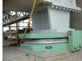
FRICTION PENDULUM BEARING SR99 Aurora Ave Bridge in Seattle
