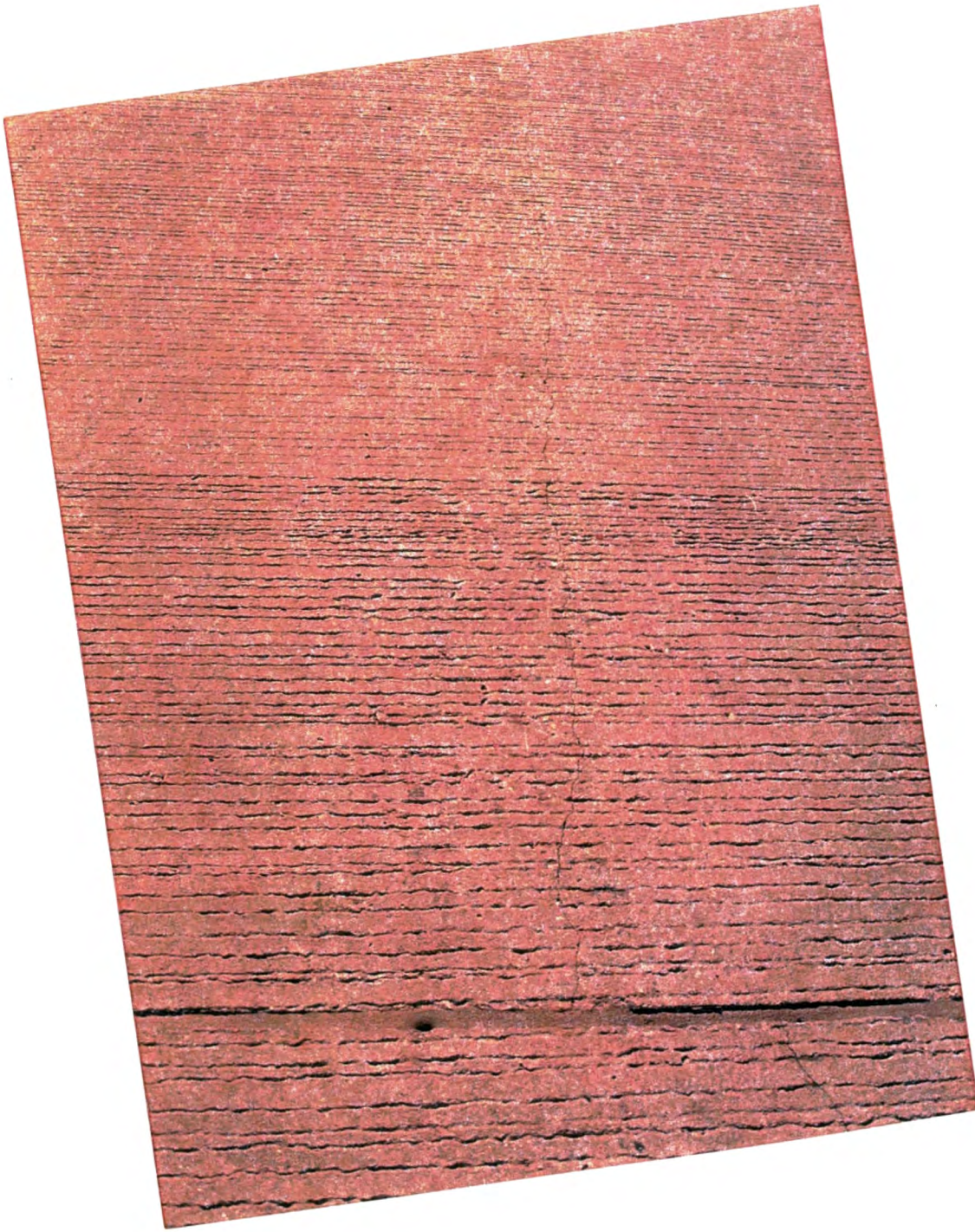
Figure 2 Longitudinal Cracking
