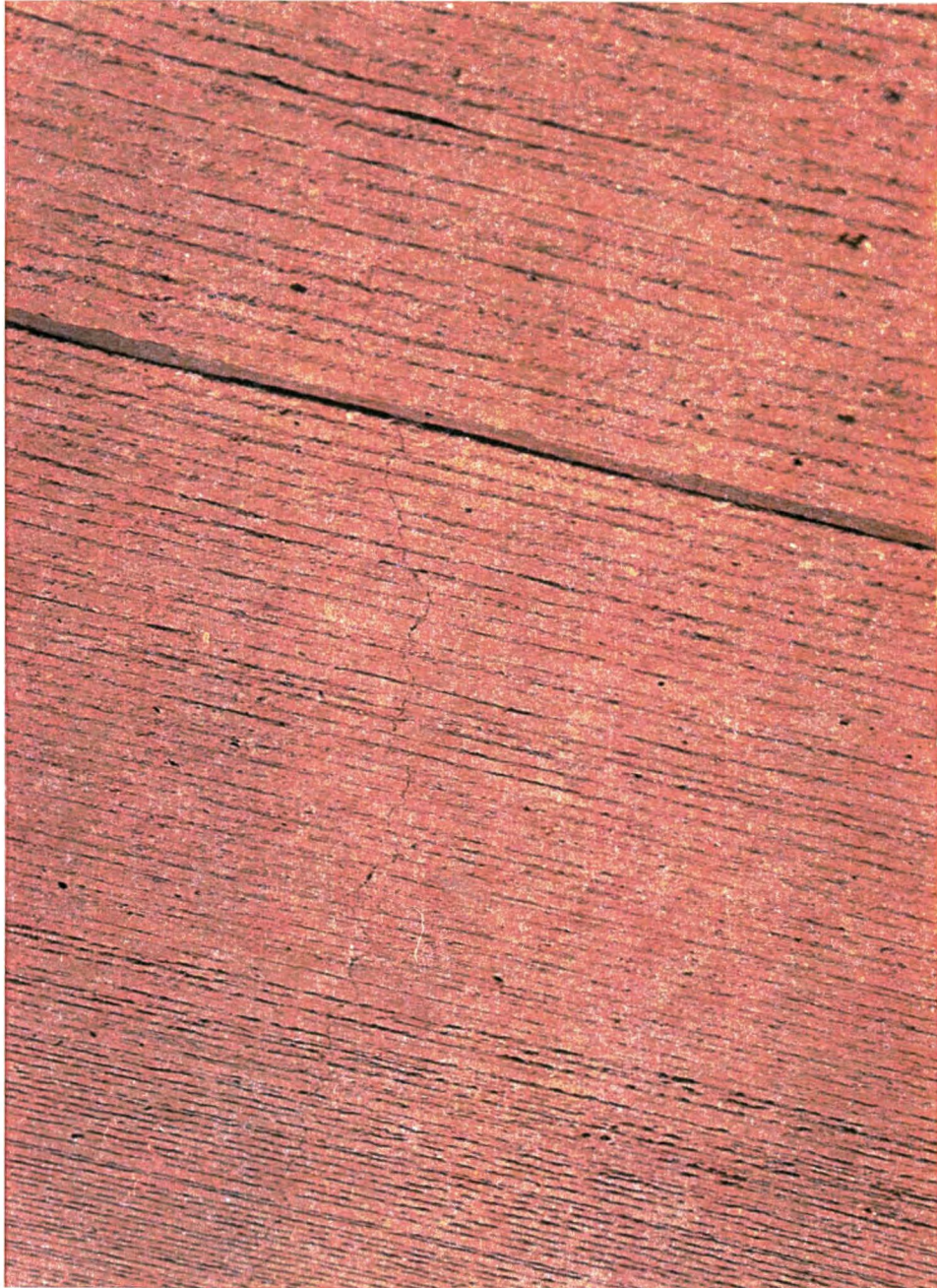
Figure 4 Longitudinal Cracking
