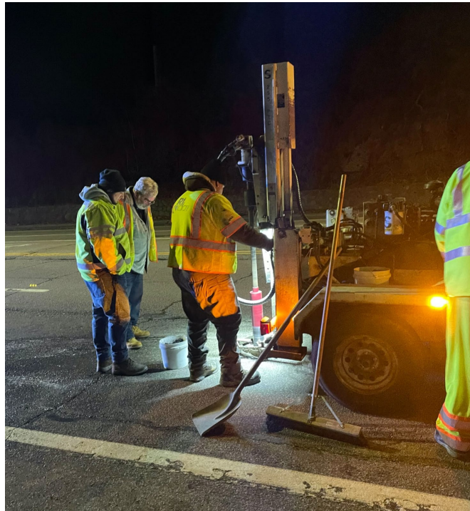
Figure 10: RIDOT taking core of Route 117
