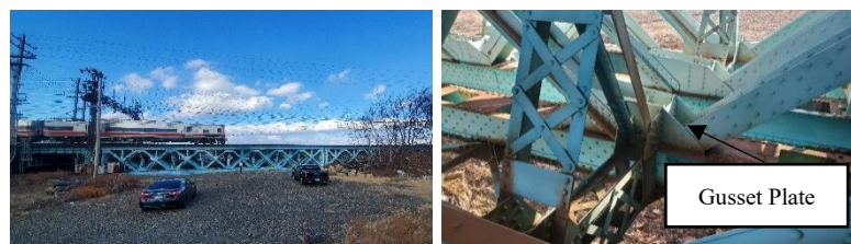
Figure 2 - Cos Cob Bridge Span 3 (left), and Gusset Plate Connection (right)
