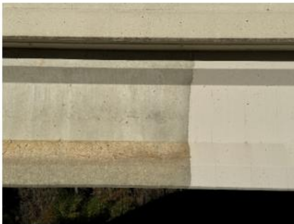
(c) The condition of the exterior beam without surface coating
