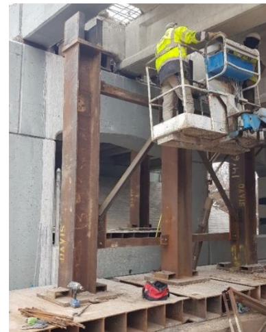
(c) Framing up the support using horizontal members
