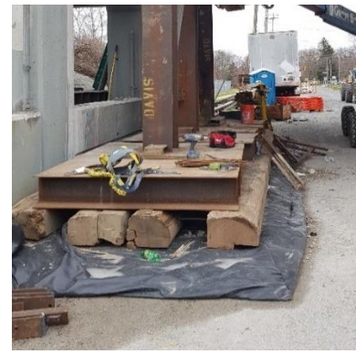
(b) Completed base support
