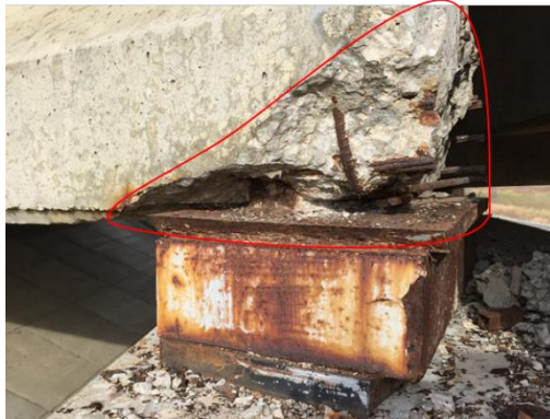
(c) Severe spall
