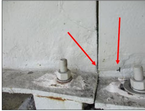
Figure 2-3. Welded repair recommended for the beam end because of \frac{1}{4} to \frac{1}{2} -in. web and flange buckling with a 3-in. long crack in the web closer to the bottom flange.
