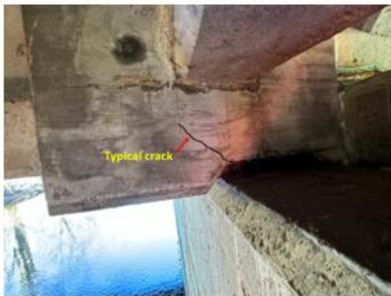
(c) Typical crack observed on unreinforced concrete overcasts
