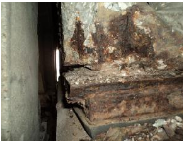
(a) Beam 3w in span 6s at pier 5s – 45% LOB due to beam end spall
