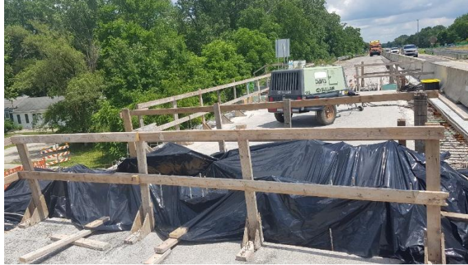
Figure F-18. Covering the concrete after placement.
