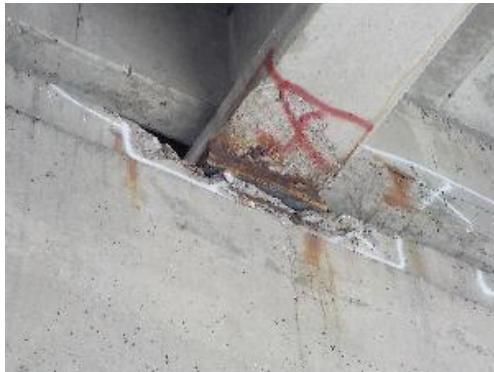
(a) Beam 3w in span 1s - undermining
