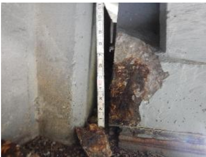
(a) Beam 7s in span 2w at pier 1w - spall on the south side of beam
