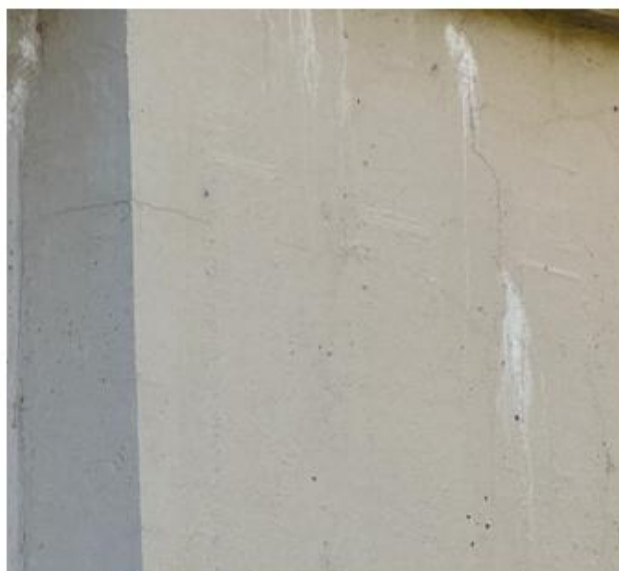
(b) A close-up view showing concrete cracking
