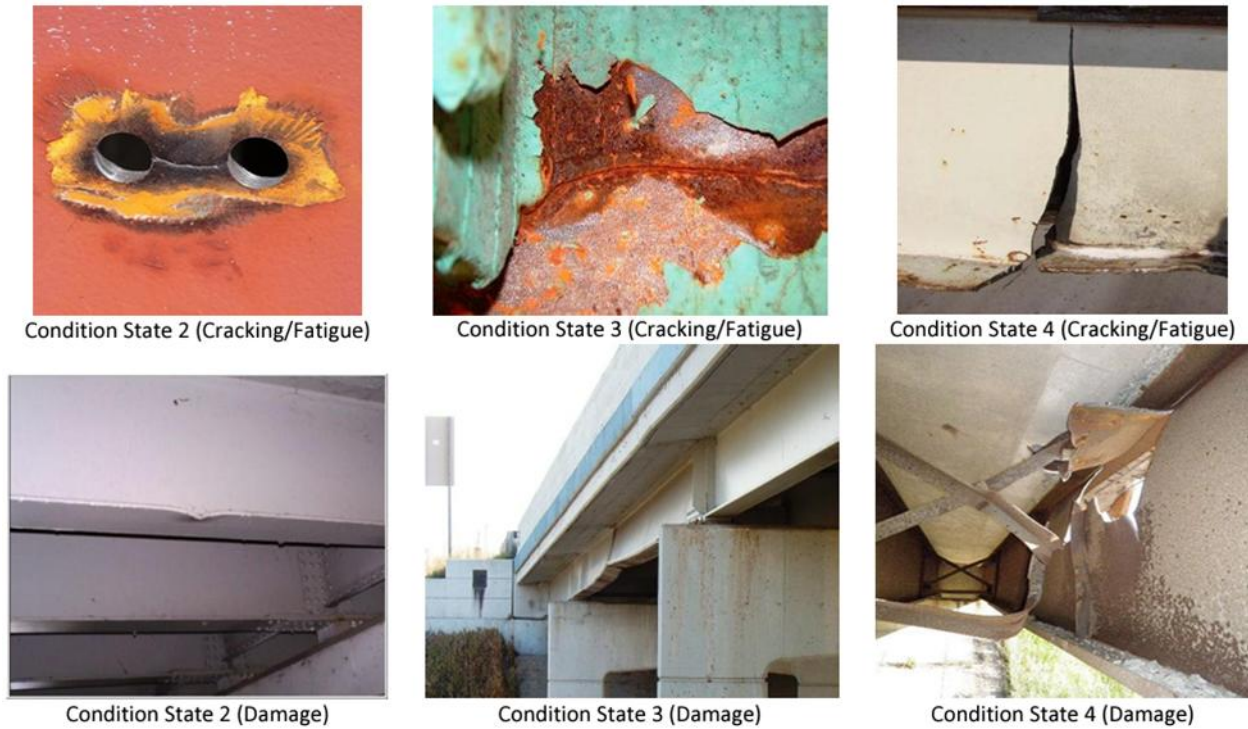
Figure 1-4. Photographs showing CS of cracked or damaged beams (Source: MiBEIM 2017).
