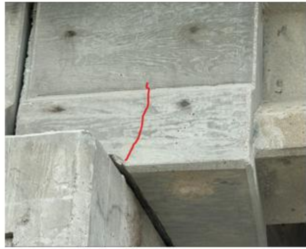
(b) Cracking on the overcast
