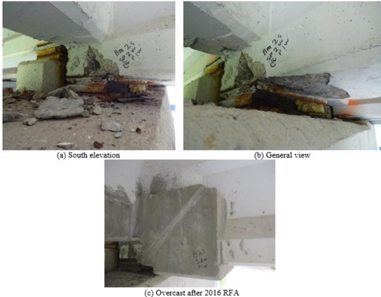
Figure D-62. The condition of beam 2s in span 2w at pier 1w as of 06/09/2016 and the subsequent repair of the beam end.
