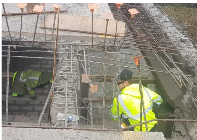
Figure F-12. Drilling holes at the beam end for adhesive anchors.
