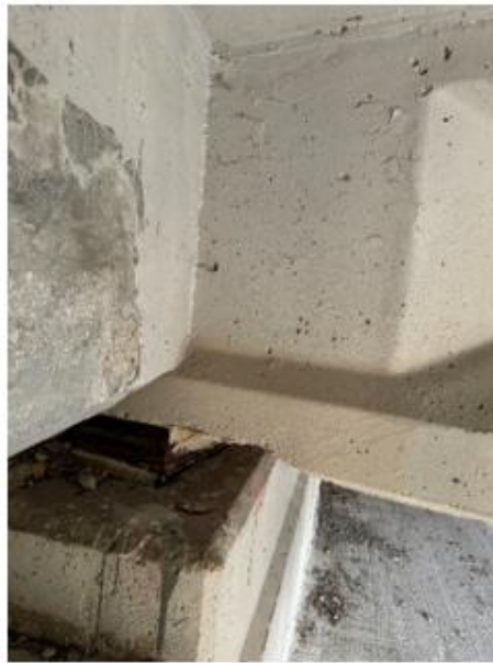
(a) Isometric view showing beam end, bearing, and end diaphragm
