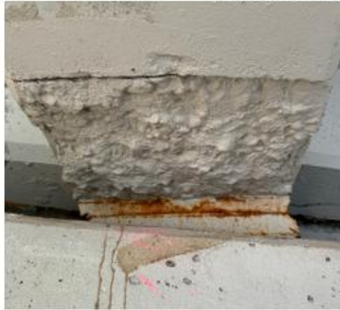
(c) Bottom flange showing the area cleaned and protected with concrete surface coating
