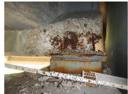
(c) Beam 3s in span 3w at pier 2w - spall with exposed steel/LOB
