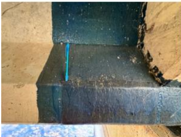
(e) Inadequate bond length leading to delamination
