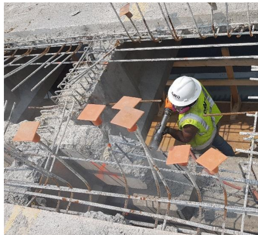
Figure F-10. Removal of an end diaphragm using a jackhammer.
