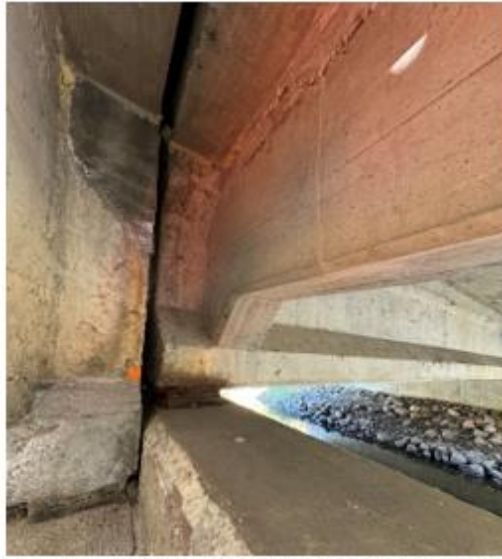
(a) Latex modified concrete repair in good condition
