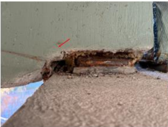
(c) Typical cracking observed in overcasts without bearing replacement
