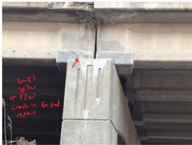
(a) Cracking of beam end repair
