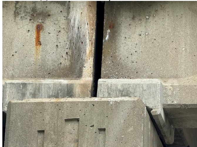
(d) Overcast with map cracking and significant moisture exposure
