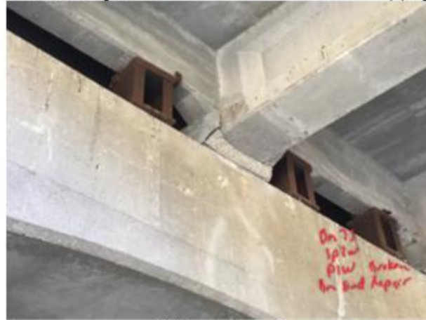
(c) Spalled repair
