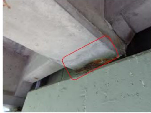
(b) Corroded sole plate
