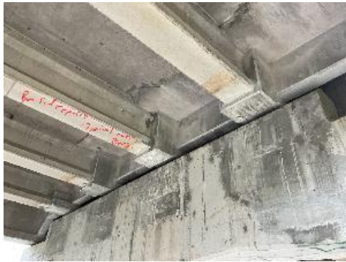
(a) Typical beam end repairs at the piers
