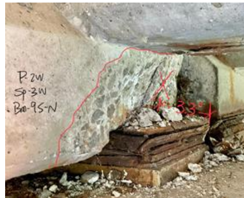
(b) Extensive spall
