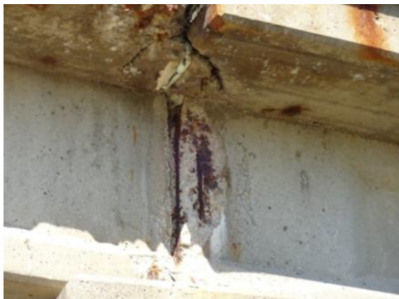
(c) STS along the vertical edge of the web and corroded stirrups
