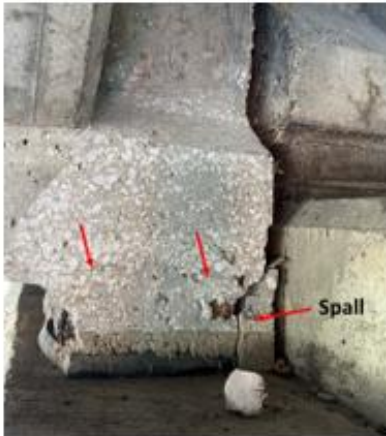
(c) An example of a poorly completed beam end repair showing cracking and spalling
