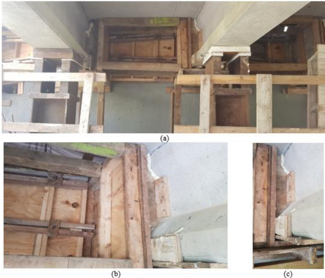
Figure F-14. Formwork for an interior beam end overcast with an end diaphragm.
