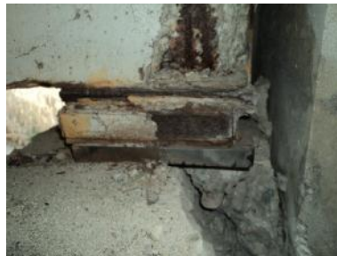
(b) Beam 4w in span 1s at pier 1s – 47% LOB due to bolster block spall
