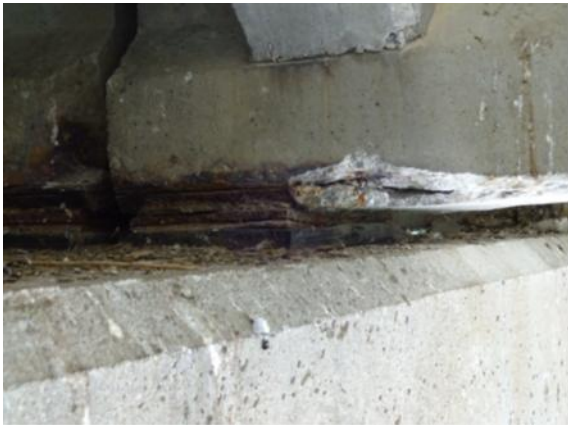
(a) Corroded sole and bearing plates and delamination in front of the sole plate
