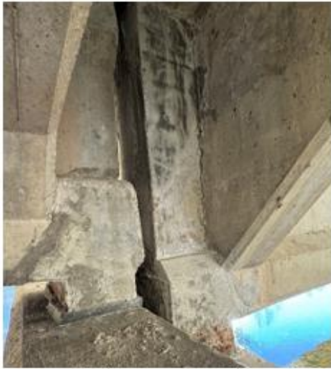
(a) Latex-modified concrete repair in good condition
