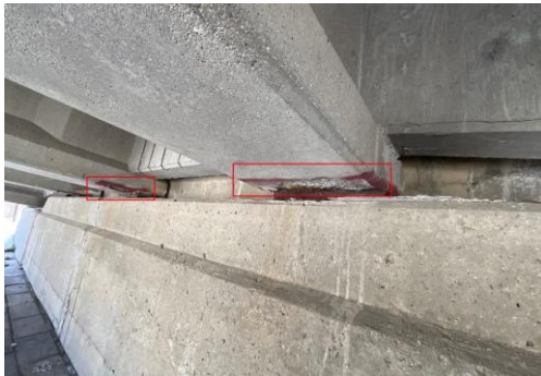
(a) Shallow delamination/spall at the beam end bottom flanges over the west abutment
