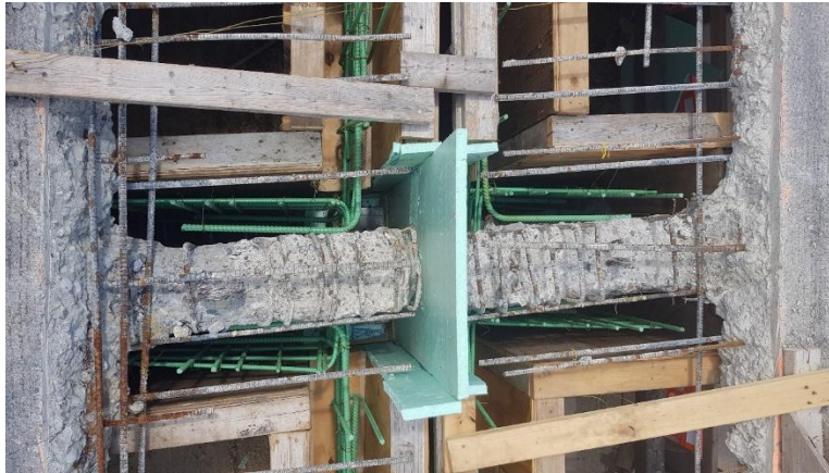
Figure F-13. Beam ends prepared for overcasts with additional reinforcement.
