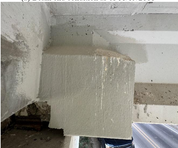
(c) Condition of beam end with CFRP wrapping as of 10/04/2024
