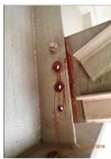
Condition State 3 (Connections)
