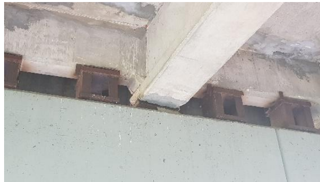
Figure G-13 Temporary supports and end diaphragm over the pier
