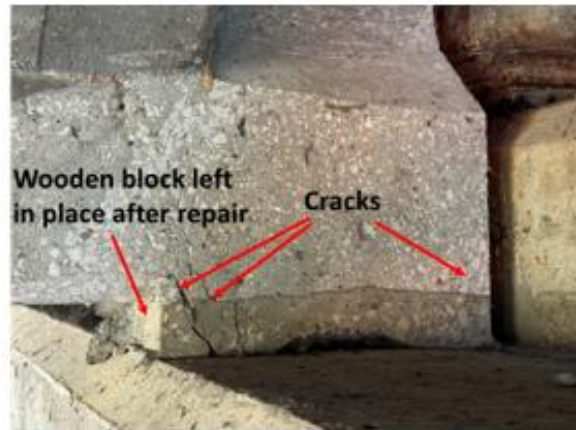
(d) Inadequately cleaned and finished repair with cracking
