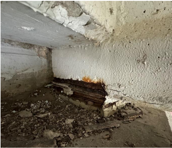
(a) Concrete cracking and delamination in front of the bearing plate
