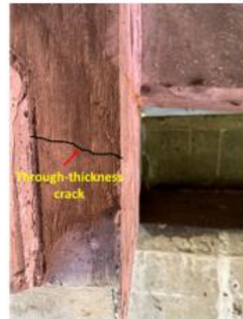
(d) Through-thickness crack in the unreinforced overcast
