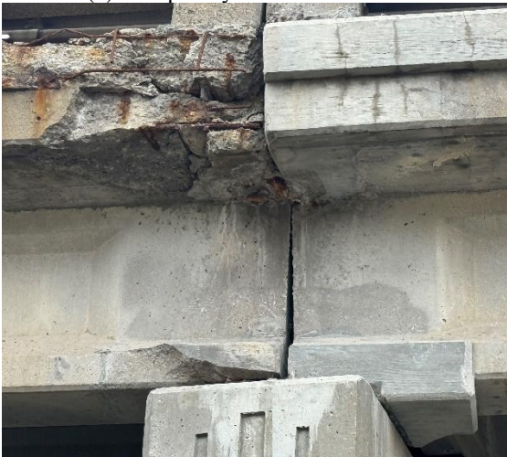
(c) Delaminated and spalled overcast
