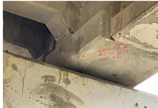
(b) Beam 1w in span 3s over pier 2s – open crack
