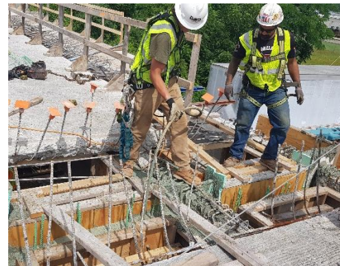
(b) Consolidation of concrete using a poker vibrator
