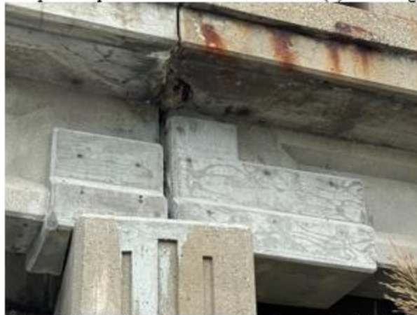
(c) South fascia beam end repairs at pier 2W
