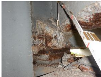
(b) Beam 5s in span 1w at pier 1w - spall with exposed steel/LOB
