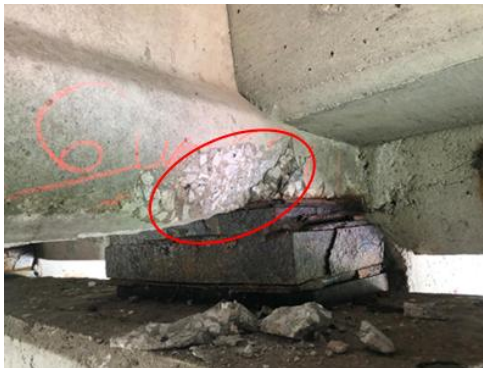
(a) Section loss in front of the bearing
