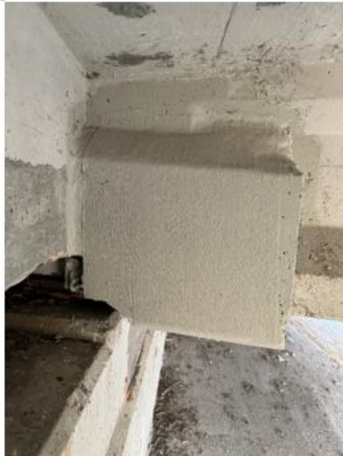
(a) Isometric view showing beam end with overcast, bearing, and end diaphragm
