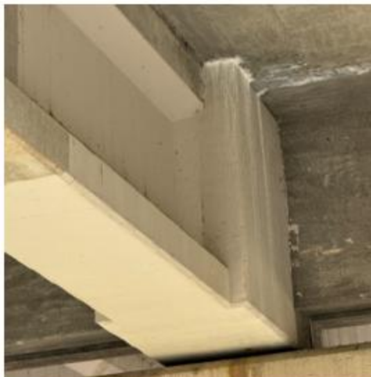
(b) Beam end with overcast exposed to moisture due to leaking bridge deck
