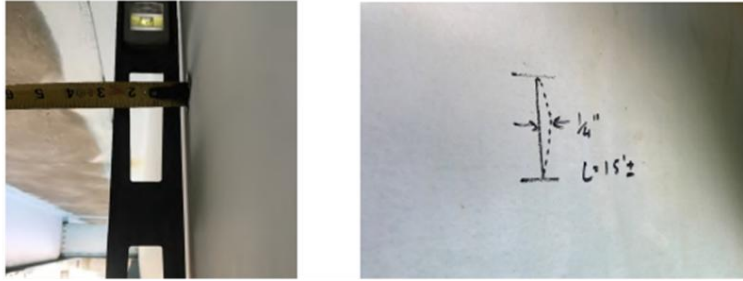
Figure 7-5. Web out-of-plane deformation measured during field inspection.
