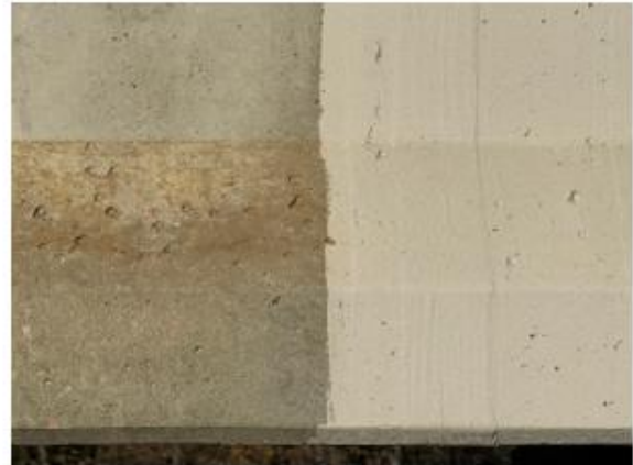
(b) A close-up view showing the effectiveness of concrete surface coating and the quality of FRP bonding
