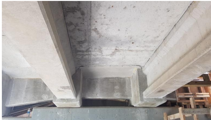
Figure F-19. Repaired beam ends after removing formwork.
