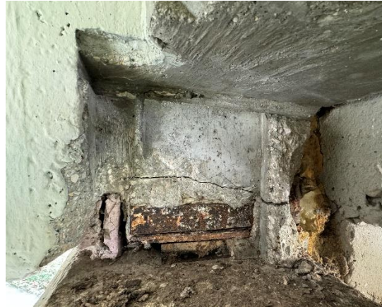
(b) Beam end cracking over the corroded bearing
