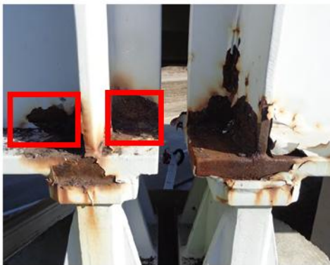
(c) Web section loss on both sides of the stiffener
