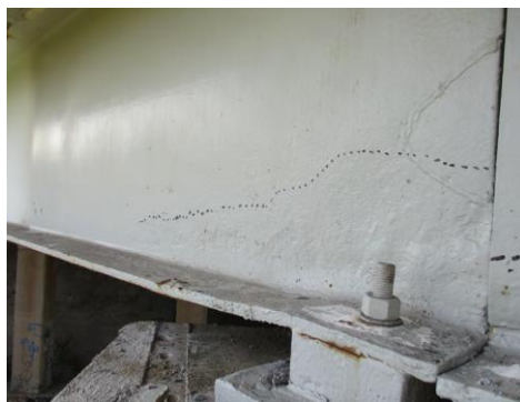
Figure 2-2. Welded repair recommended for the beam end because of ¼ to ½-in. web and flange buckling.
