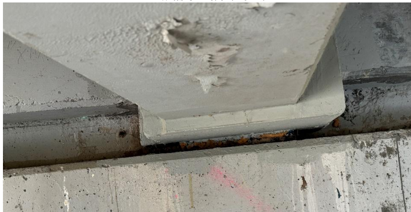
(a) Uneven thickness of the overcast and damaged concrete surface coating
