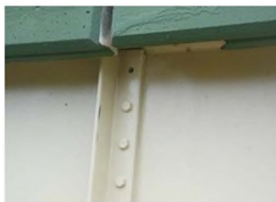
Condition State 2 (Connections)
