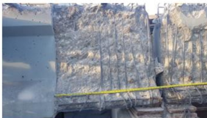
(c) Chipped out and cleaned beam ends
