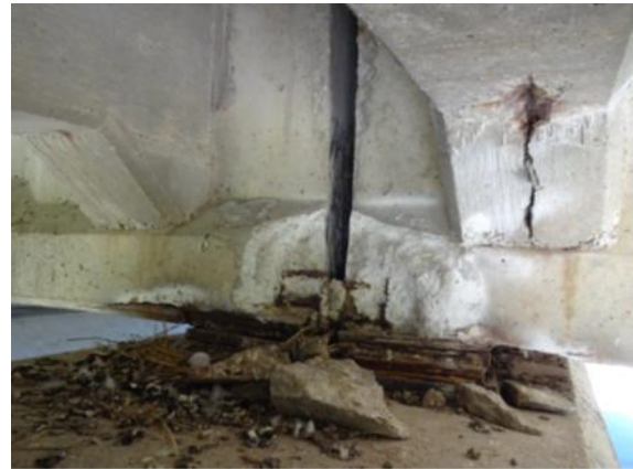
(b) Corroded sole and bearing plates, delamination and spall front of the sole plate, STS at beam ends and over the bearing, and corroded stirrups and strands
