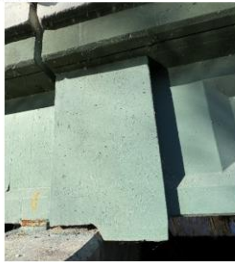
(c) Overcast protected with CSC without FRP
