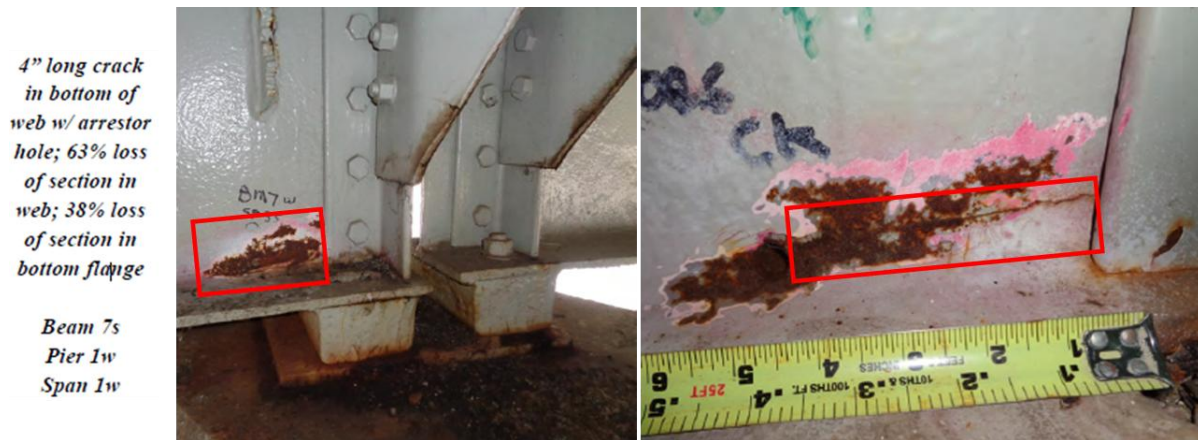
Figure 8-1. Beam end with a 4 in. long crack (STR 10907).
