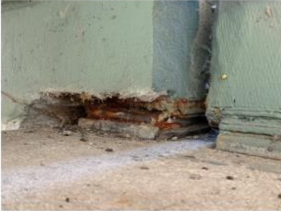
(a) Corroded sole plate and bearing plate promoting deterioration
