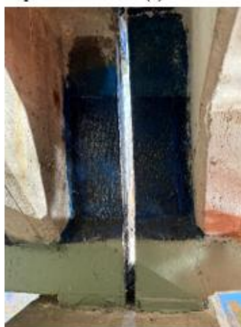
(d) Beam end with partial-height repair, FRP, and CSC
