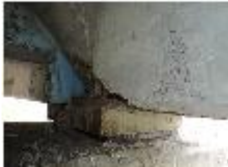
(a) Beam 1w in span 3s at pier 2s - spall with 14% LOB
