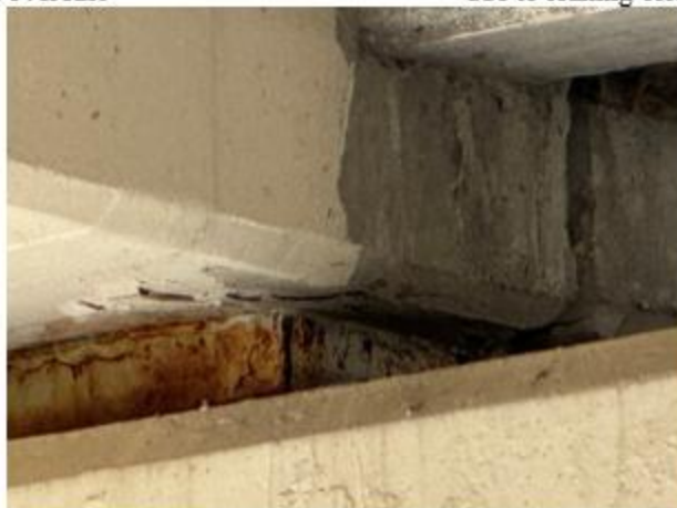
(c) Delamination over the bearing plate
