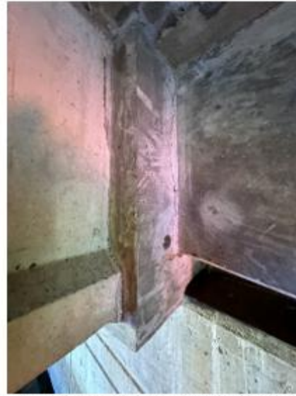
(b) Unreinforced concrete full-depth overcast
