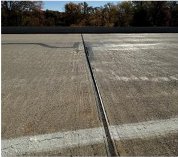
(a) An expansion joint over a pier filled with debris
