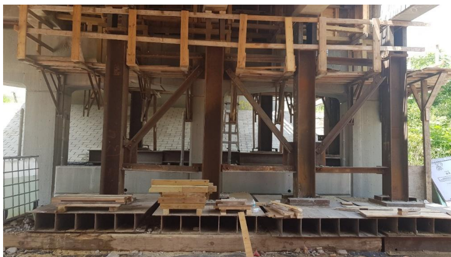
Figure F-7. Temporary support system with a working platform.
