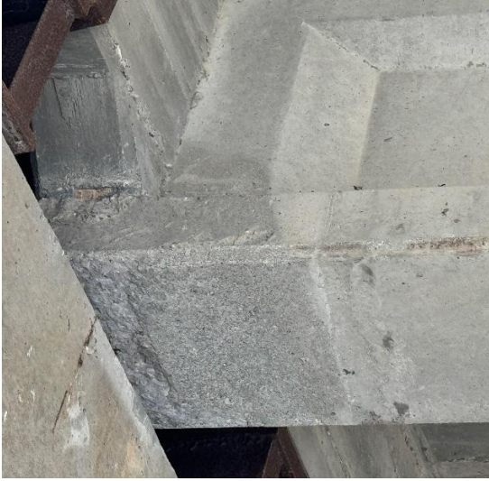
(a) Completely removed overcast
