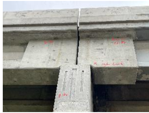
(b) Beam 6w in span 5s at pier 4s – tight crack
