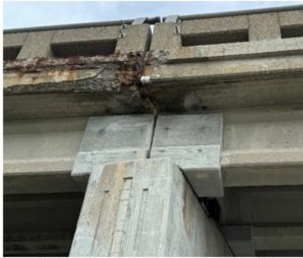
(a) South fascia beam end repairs at pier 1W
