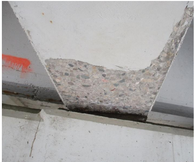
(b) Shallow spall at the bottom flange soffit
