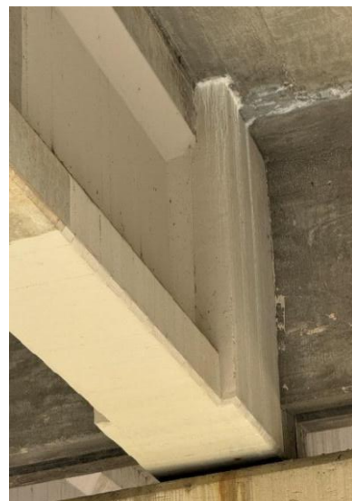
(b) Isometric view showing a leaky deck
