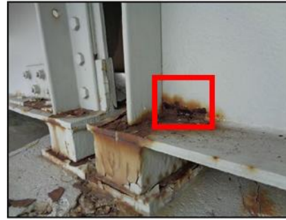
(b) Web section loss towards the span of the stiffener
