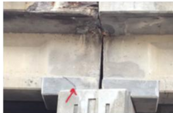
(b) Overcast at the bottom flange
