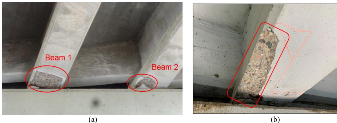
Figure 4-23. Section loss at the beam soffit without exposing strands or reinforcement.
