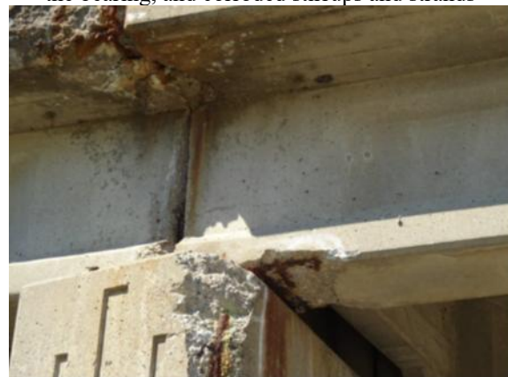
(d) STS in front of the sole plate and corroded stirrups and strands
