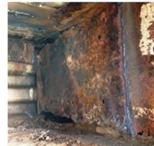
Condition State 4 (Corrosion)
