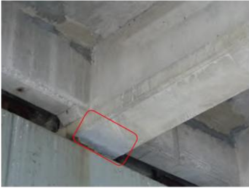
(a) The sole plate is in good condition
