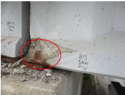
(a) Moderate spall
