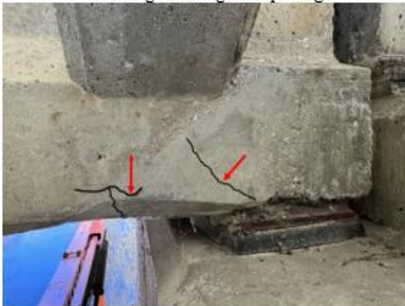
(e) Typical cracks in beam end repairs
