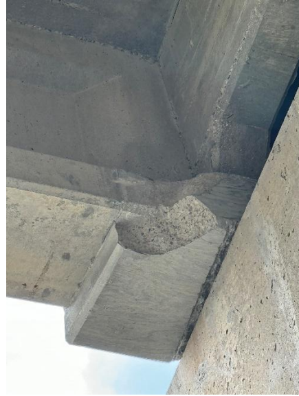
(b) Delaminated and spalled overcast
