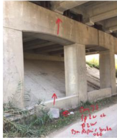
(b) Spalled repair
