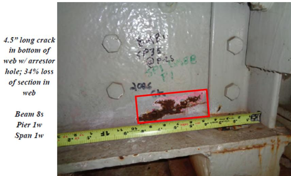
Figure 8-2. Beam end with a 4.5 in. long crack (STR 10907).
