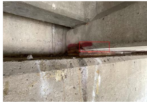
(b) Shallow delamination/spall at the beam end bottom flanges over the east abutment
