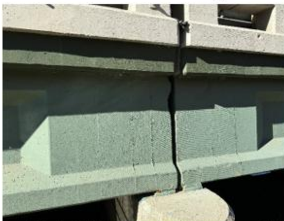
(b) Partial-height repair with FRP U-wraps and CSC
