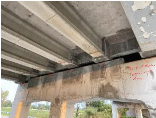
(a) Typical beam end repair at the piers
