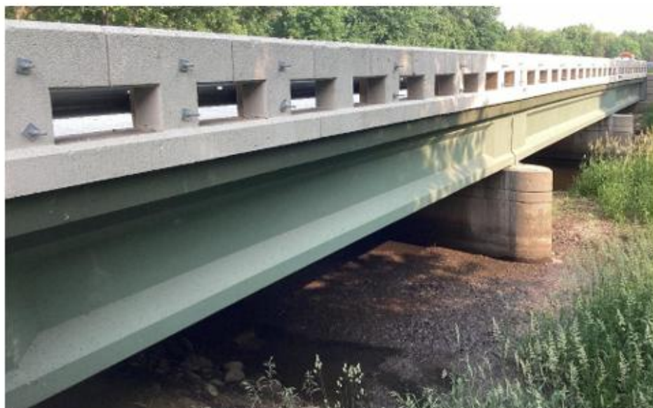
(a) Fascia beam protected with CSC
