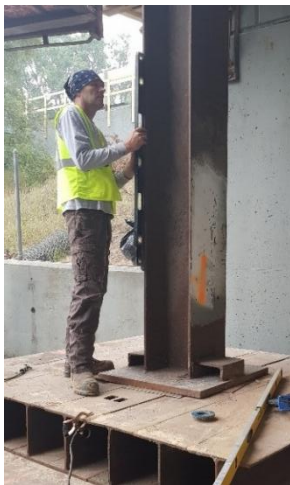
(a) Column alignment check
