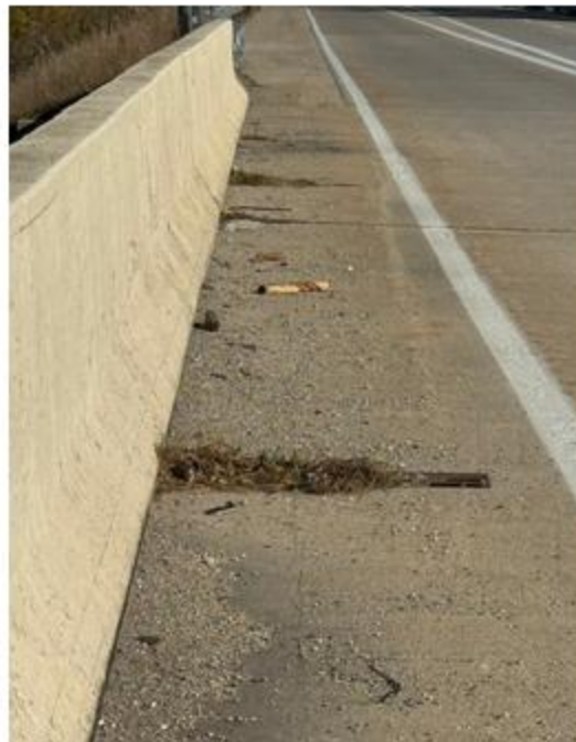
(c) Partially clogged deck drains
