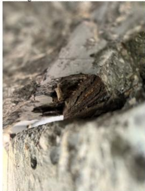
(d) Concrete spall between the overcast and the corroded bearing
