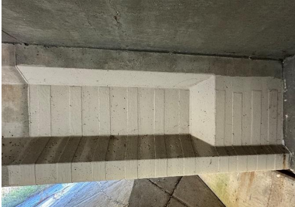
(a) Elevation view of an interior beam end
