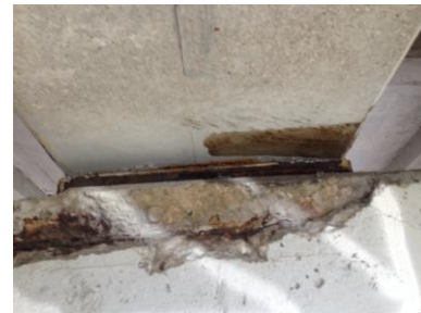
(c) Beam 5w in span 4s at pier 4s – 100% of bearing is on delaminated concrete
