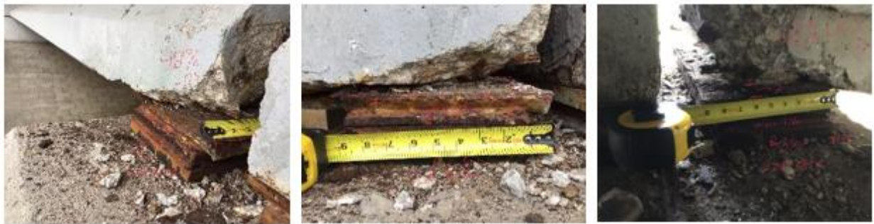
Figure D-13. The condition of beam 6w in span 1s over pier 1s with 48% LOB.
