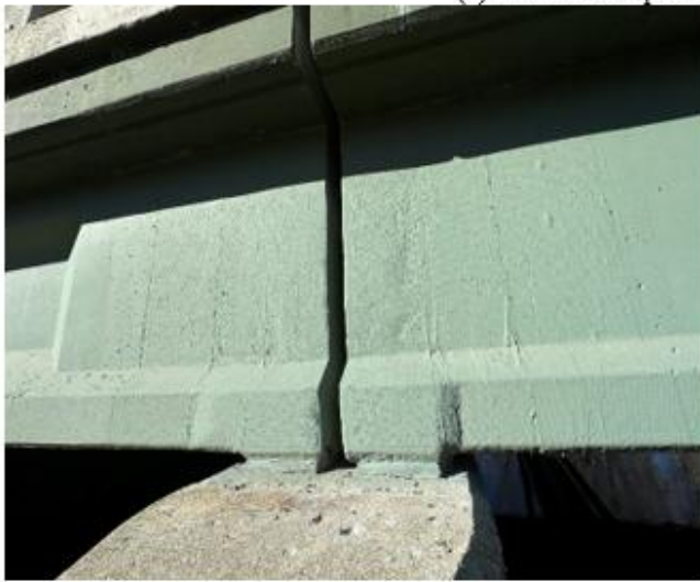
(b) Repair with FRP U-wraps and CSC
