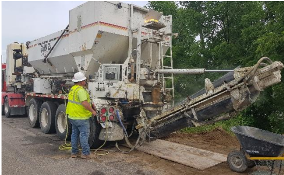
(a) Mobile volumetric concrete mixer
