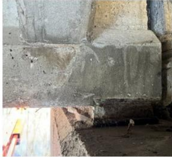
(b) An example of a correctly completed beam end repair
