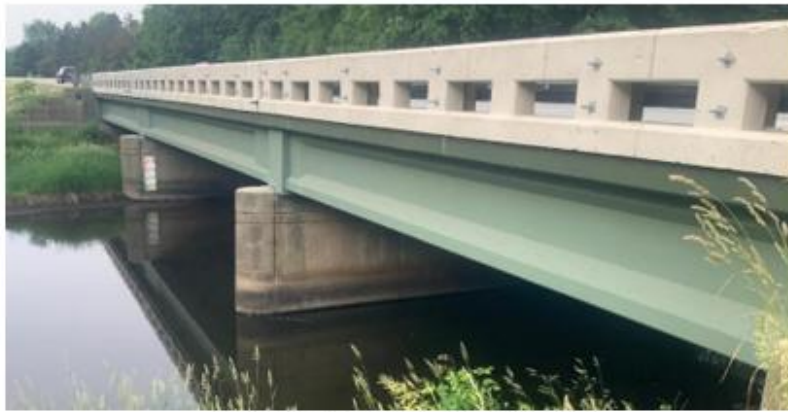
(a) Fascia beam protected with CSC
