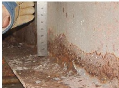
Condition State 3 (Corrosion)
