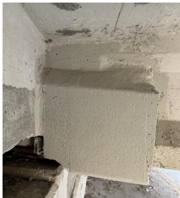
(a) Overcast up to the top flange
