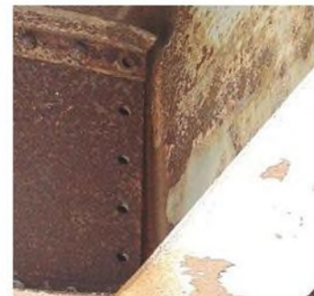
Condition State 4 (Connections)
