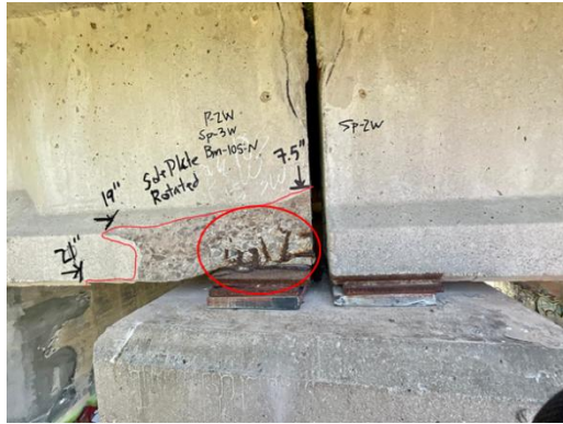
(a) Moderate spall
