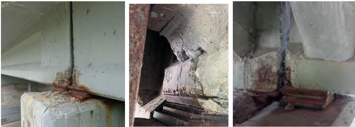
(a) Spall and corroded bearing (b) Cracking, delamination, and spall (c) Spall behind the bearing
