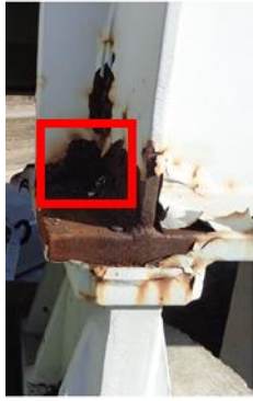
(a) Web section loss between the beam end and the stiffener
