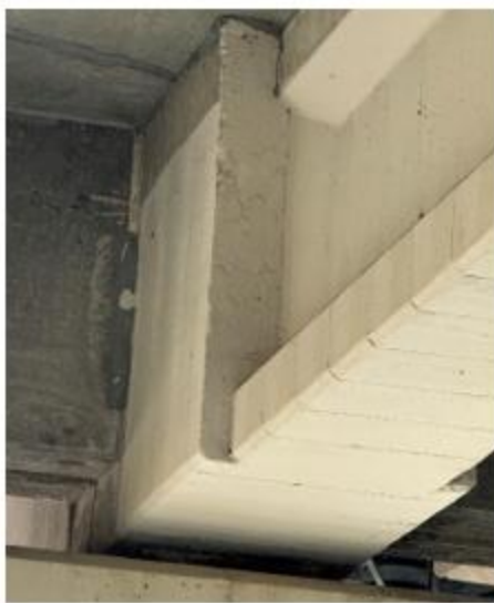
a) General view of an interior beam end with an overcast
