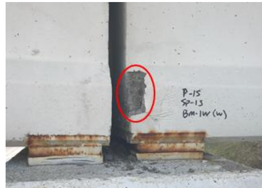
(b) Section loss at the beam end
