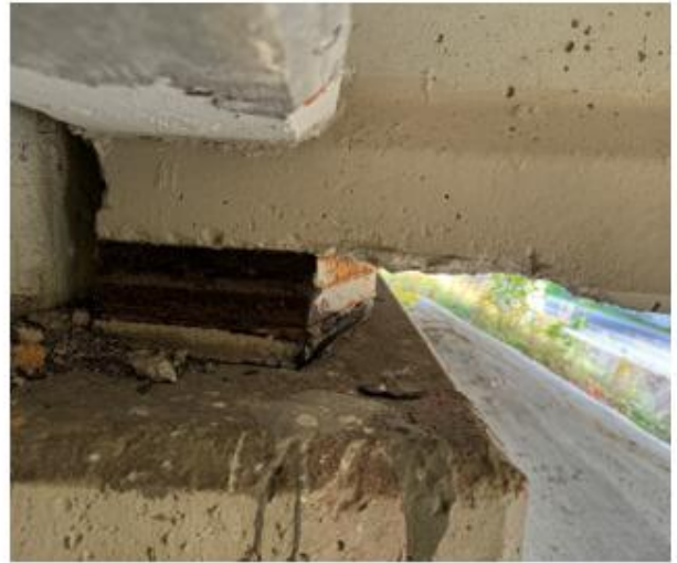
(b) Close-up of beam end showing bearing and a section with concrete removed from the bottom flange
