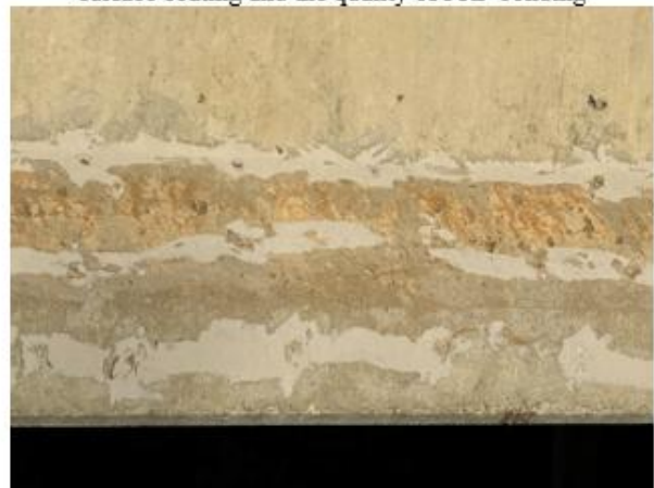
(c) The condition of the exterior beam without surface coating
