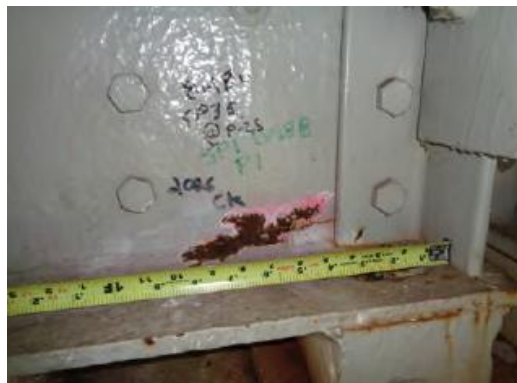
Figure 2-4. Welded repair recommended because of a 4.5-in. long crack and 34% section loss.
