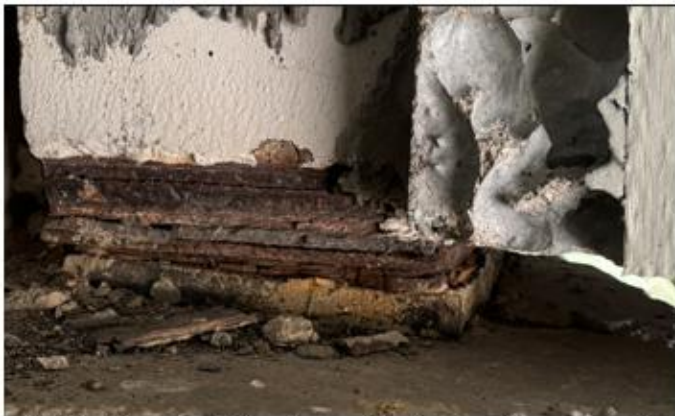
(c) Heavily corroded bearing and the bottom flange over the bearing protected with a concrete surface coating
