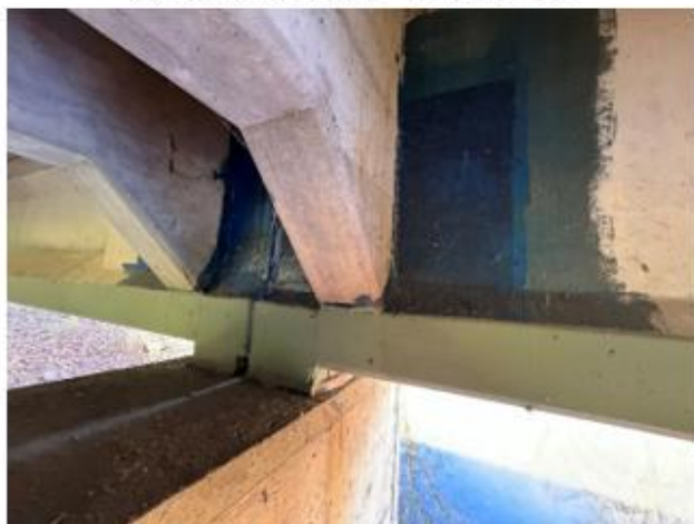
(d) Beam end with partial-height repair, FRP, and CSC
