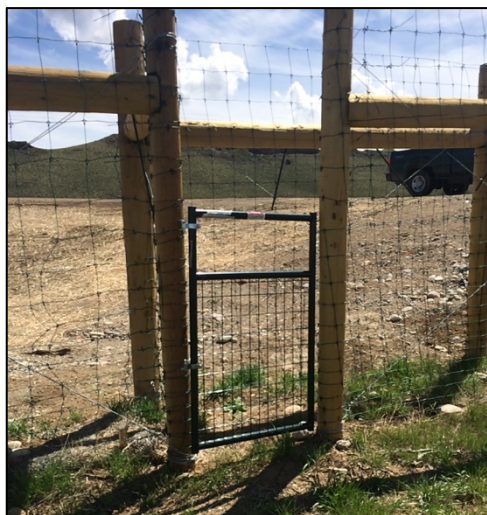
Figure 36. Pedestrian walk-through gate equipped with swing gate.
