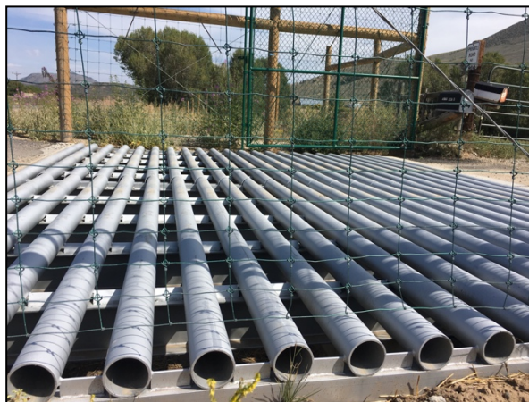
Figure 16. Round bar deer guard design installed at select locations during Phase 2 construction.
