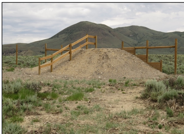
Figure 17. Examples of escape ramp with 2:1 slope and rail fence (left) and 3:1 slope with no rail fence (right).
