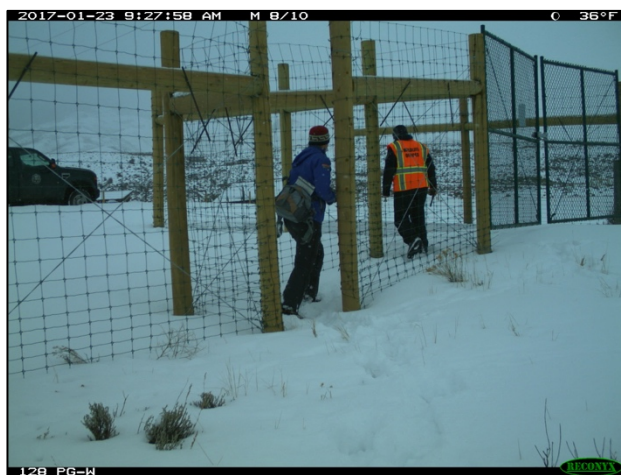
Figure 18. a) Y-shaped pedestrian gate design used in Montana (left, photo credit: M. Huijser); b) modified right-angle design used by CDOT (above).
