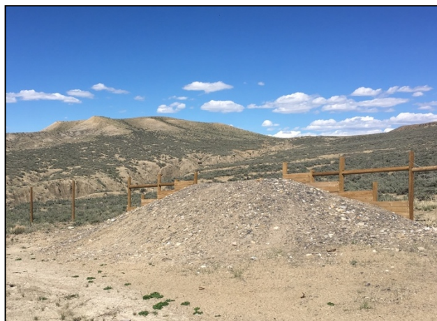
Figure 17. Examples of escape ramp with 2:1 slope and rail fence (left) and 3:1 slope with no rail fence (right).
