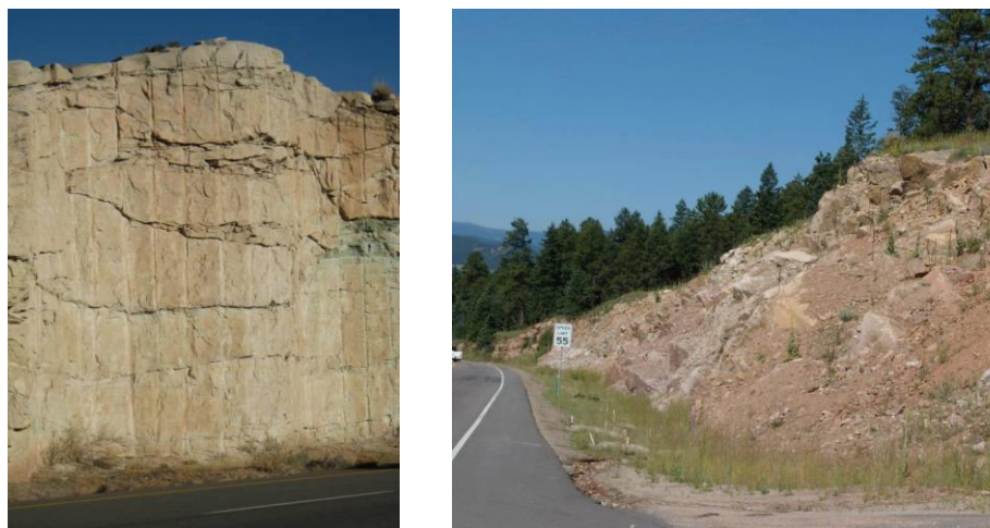
Figure 11. Presplitting in sandstone (left) and cushion-blasted granitic rock (right) [2]
