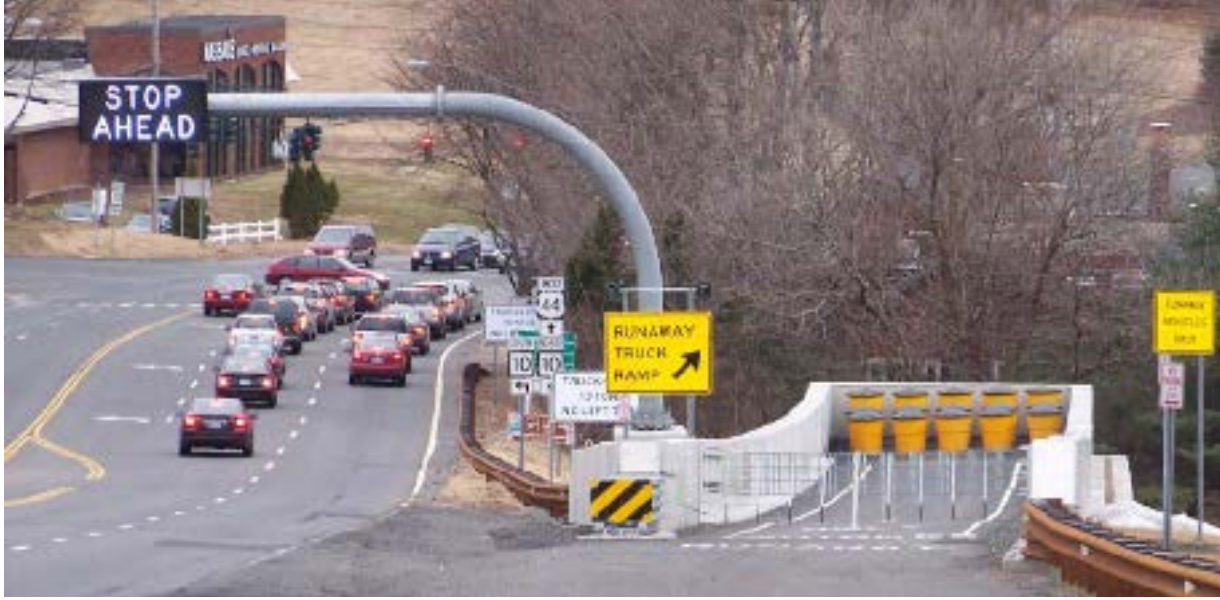
Figure 1.7. Dragnet Arrestor Bed EER with U.44/CT 10/Nod Rd. Intersection in Background Reprinted from Connecticut Department of Transportation's Truck Escape Ramp (TER) (12), 2010, Avon CT.
