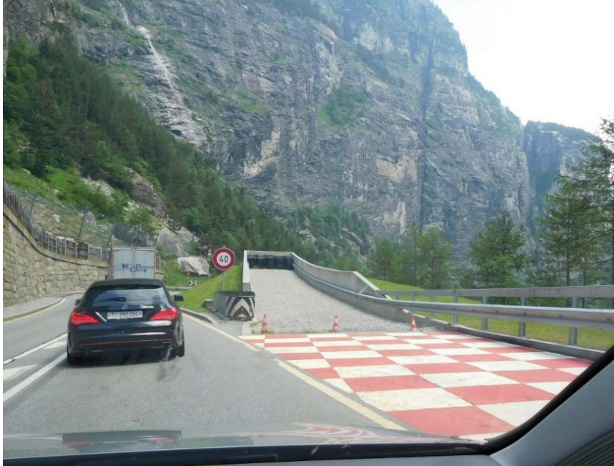
Figure 6.4. Truck Escape Ramp in Switzerland
