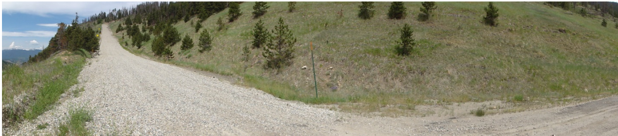
Figure 2.2. Panoramic View of the Lower Straight Creek Ramp
