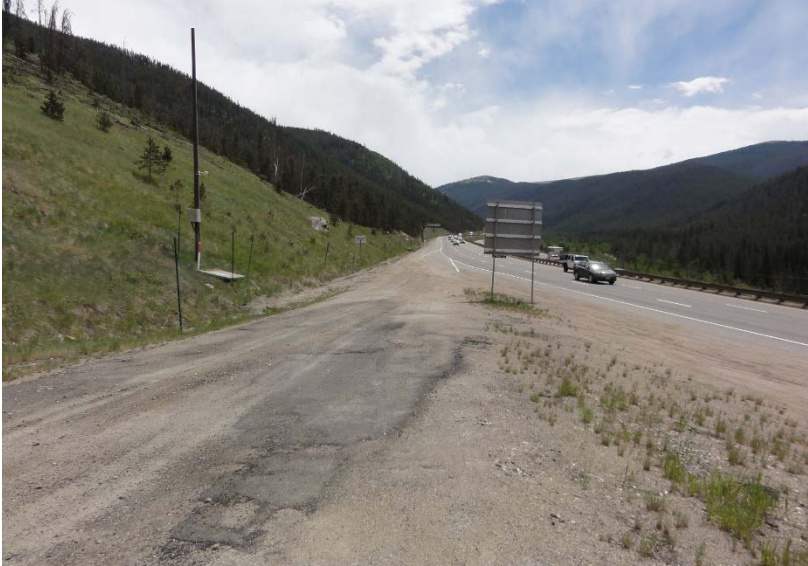
Figure 2.3. The Lower Straight Creek Ramp Entrance
