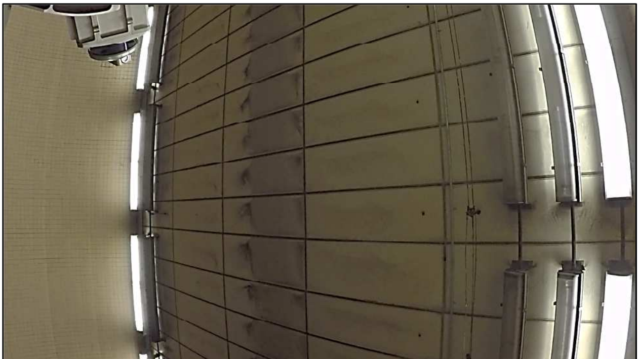
Figure 54: Hanging Lake Tunnels RGB
