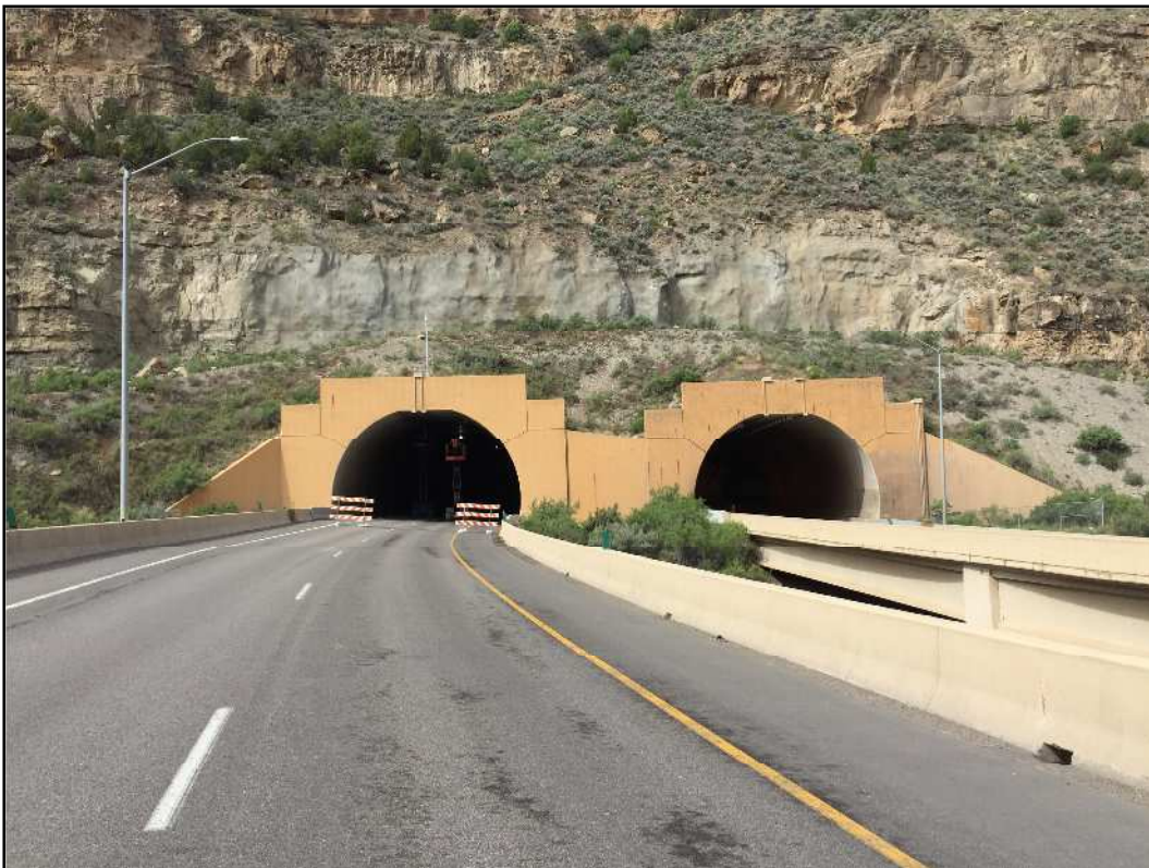
Figure 33: East portals of Beavertail Tunnel approach
