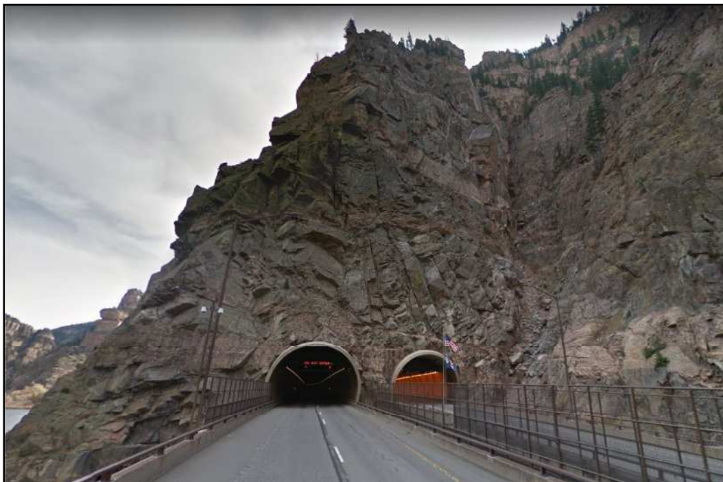
Figure 46: West portals of Hanging Lake Tunnel
