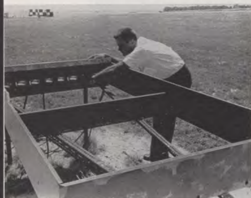
NAFEC has outstanding record in field of airport lighting. Below, engineer adjusts lights on test visual approach indicator. Right, checking "pancake" light for even intensity.
