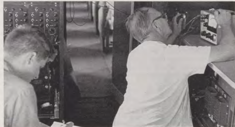
More than 1100 successful "hands-off" landings have been made in FAA DC-7 aircraft fitted with developmental automatic all-weather landing system. Above, automatic approach. Below, checking gear.
