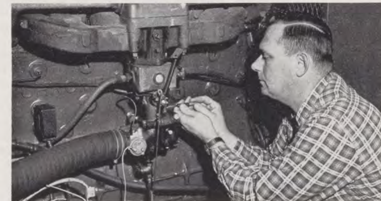
Electro-mechanical technician tunes up standby generator.
