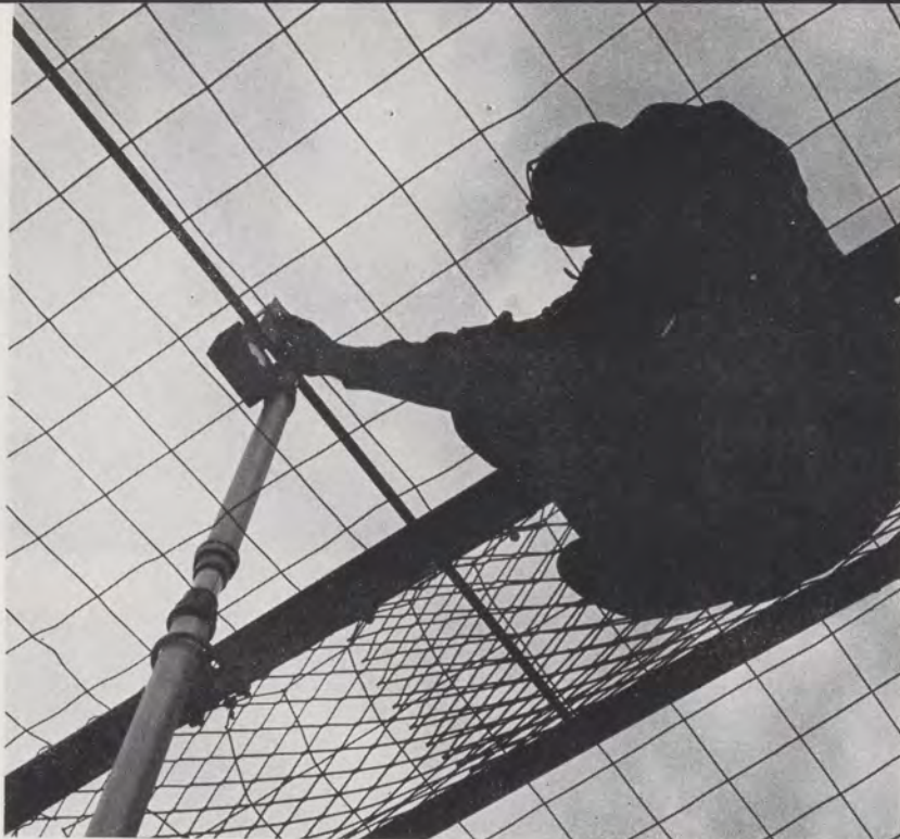
Left, on the "bedsprings" antenna of fan marker, FAA technician records current. Remote UHF transmitter above, and receiver in airport control tower below, get overhaul to keep them in top operation condition.
