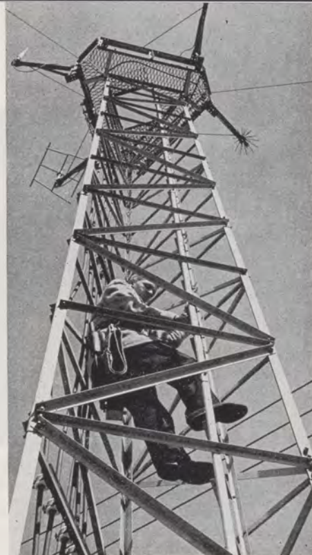
Above, an electronics technician climbs a remote control air-ground tower to check the antenna. Above right, day and night they are on the job, keeping facilities operating. Right, technician tests accuracy of the course radiated by a VORTAC.
