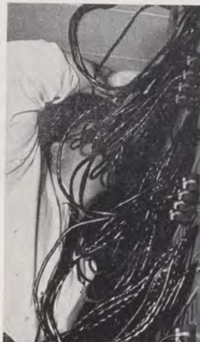
Left, technician checks for break in wire patch cord panel, part of tower communications gear. Right, Weather Bureau teletypewriter gets same meticulous care as more complicated equipment.
