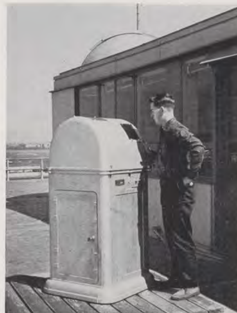
Above, weather observer checks ceilometer which measures height of cloud bases with photo-electric cell that scans sky. He can also obtain the information, plus other data, from remote console (right).
