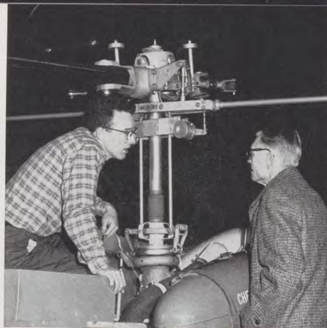
Another inspector checks technician's repair work on helicopter rotor.
