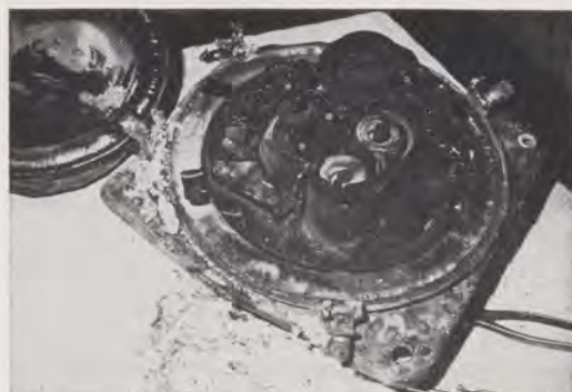
This battered recorder was recovered from a Viscount turboprop which crashed near Baltimore on November 23, 1962. Below is the CAB's machine for analyzing tapes.
