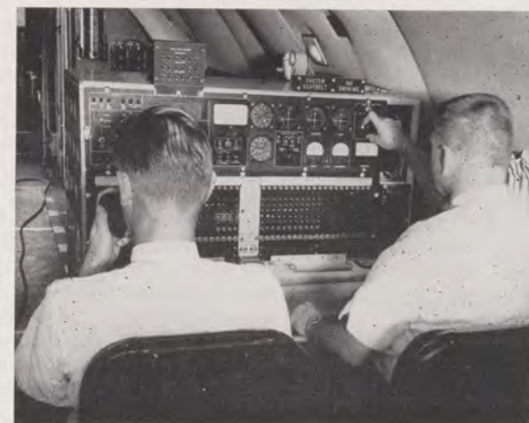
Upper left, electronic technicians of C-135 flight inspection crew monitor sensitive measuring equipment. Left, Convair crew operates control panel in checking facility performance. Above, analog recorder gives instant readout information.
