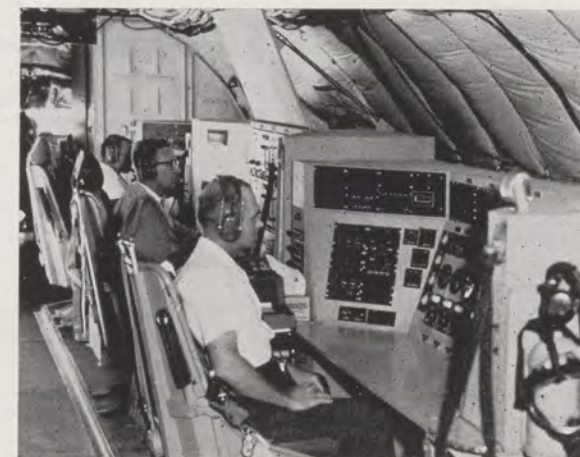
Grid covering entire nation is used with electronic computer for semi-automatic flight inspection.
