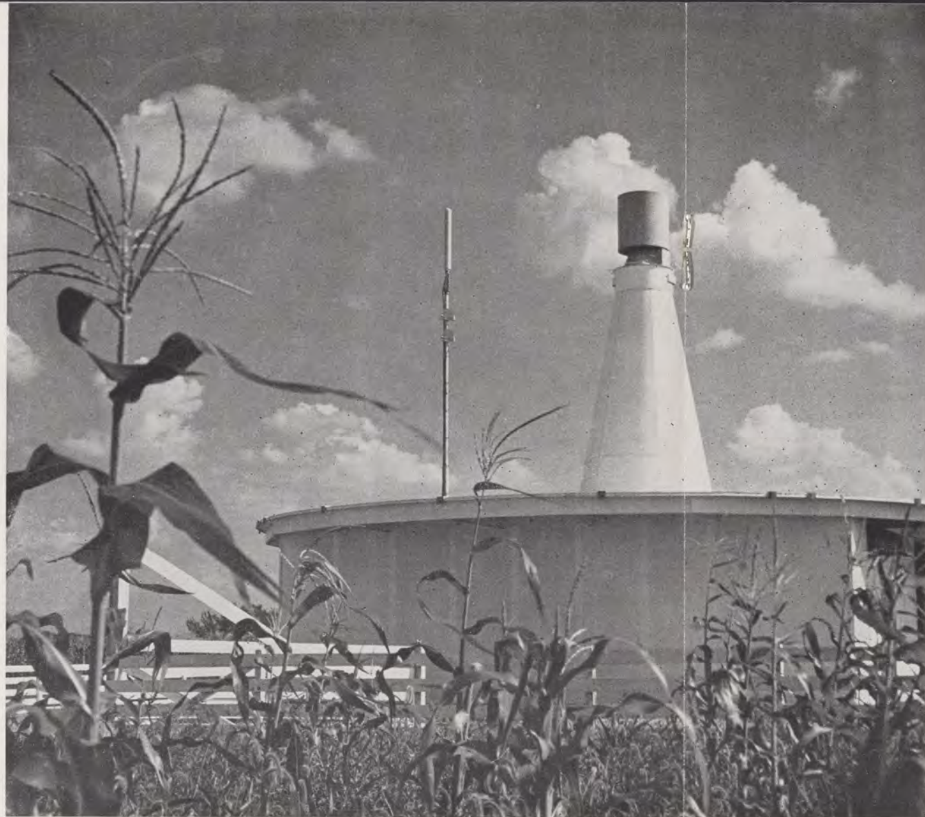
VORTACs, which provide aircraft with both distance and direction information, are key navigational facilities whose accuracy must be maintained by FAA.
