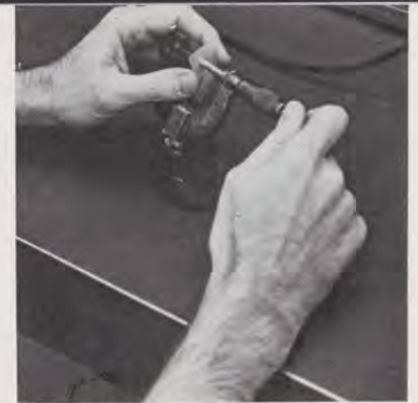
Technician in Depot Shop mikes a piece of quartz crystal as the first step in producing an accurately ground Piezo-electric frequency control device.
