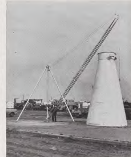
FAA design engineer checks specially-built hoist equipment used to help install TACAN antennas.
