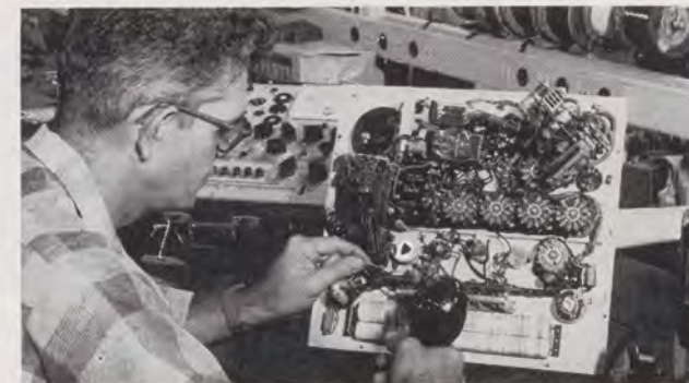
Overhaul and calibration of testing equipment, such as this tube tester, is another important job in assuring reliability of nav aids.
