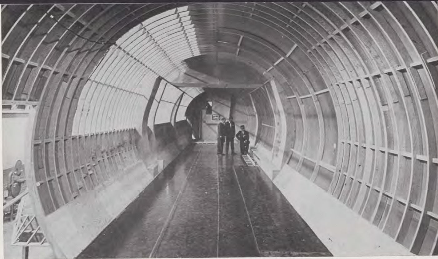
Mammoth interior of mockup of Lockheed C-141 Starlifter jet cargo plane designed with both military and civil requirements in mind.
