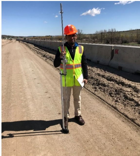
Figure 11. Interstate 25 South Gap Test Site in Larkspur
