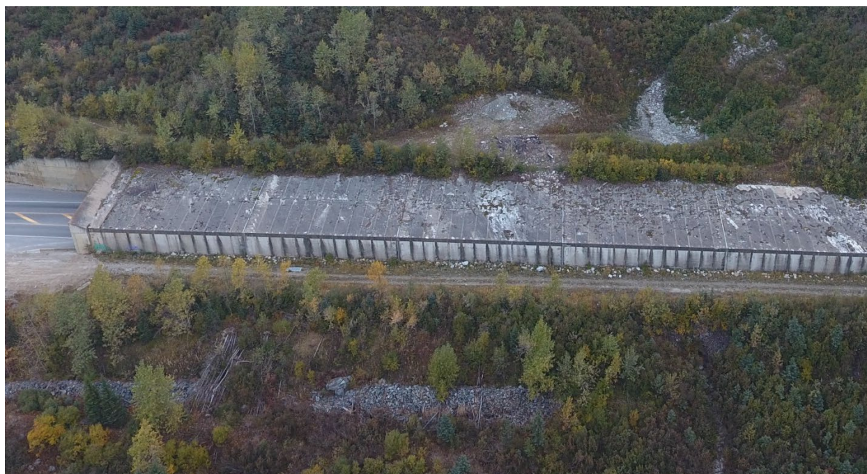
Figure 36: Single Bench snow shed in Rogers Pass, BC showing evidence of debris and rockfall impacts on the concrete roof slabs (Photo: Dynamic Avalanche Consulting)
