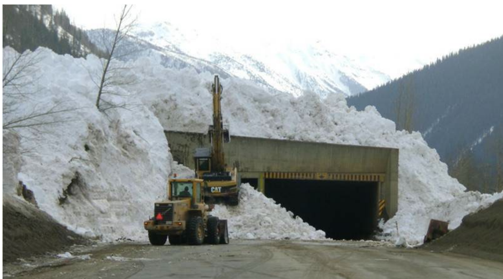
Figure 41: Single Bench overflow at the west portal due to a glide slab avalanche from the adjacent Mounds avalanche path, April 10, 2012. (Photo: Parks Canada Agency)
