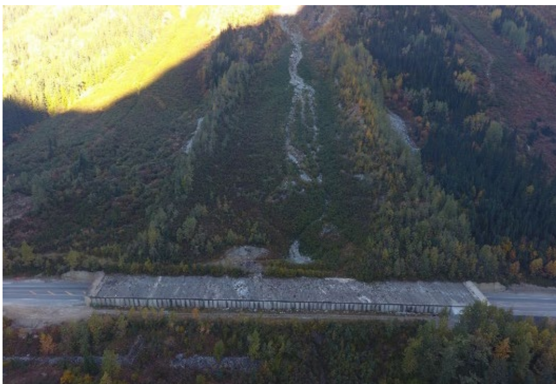
Figure 40: Single Bench avalanche path above the Single Bench snow shed. Single Bench avalanche path is the main path in the center of the photo, directed over the shed and confined by lateral guiding berms. The Mounds avalanche path is immediately west (photo left) of the shed. The Crossover avalanche path affects the shed from the opposite (south) side of the valley, requiring protection of the downslope shed wall (Photo: Dynamic Avalanche Consulting)
