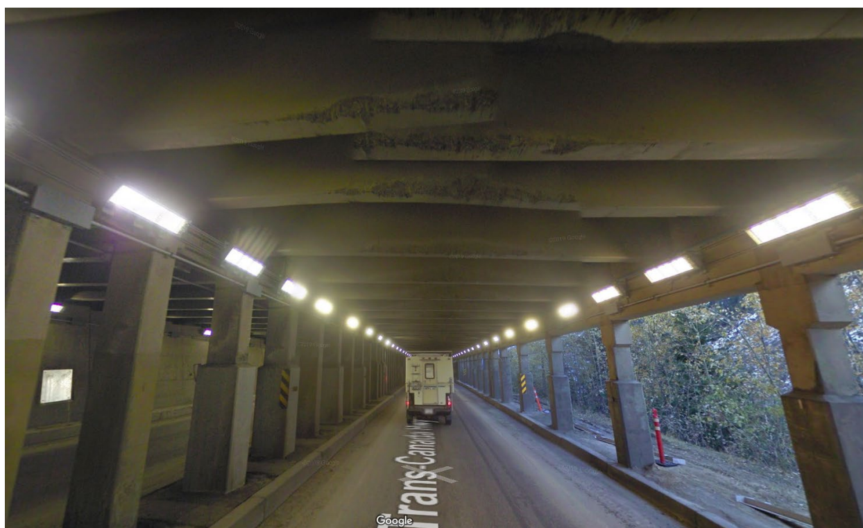
Figure 32: Overhead damage to the Tupper #1 snow shed has occurred where the original metal arch-shaped Pioneer shed joins the flat-roofed concrete Tupper #1 shed (Photo: Google Earth, 2020).
