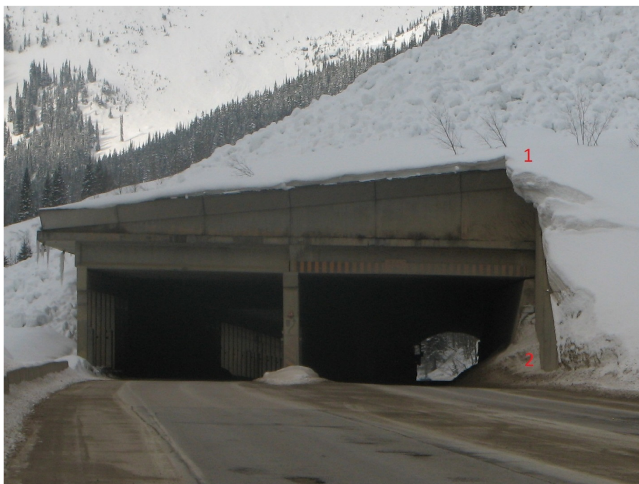
Figure 35: Two snow shed maintenance issues: (1) overhanging cornice snow and (2) snow accumulation at the portal (Photo: Alan Jones)
