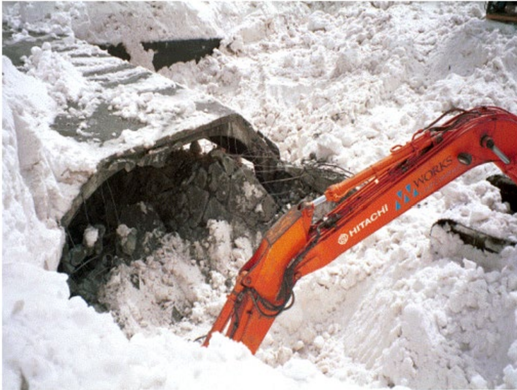
Figure 28: An avalanche on October 7, 1996 damaged the east portal of Homer tunnel. Impact pressures of 650-700 kPa were estimated, and resulted in damage to the reinforced-concrete portal structure (Conway et al., 2000).
