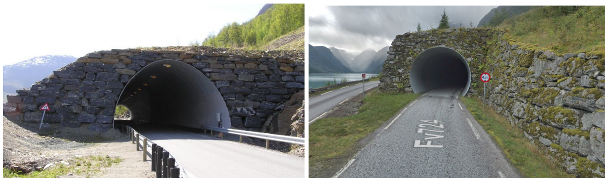
Figure 24: A snow shed near Ellevoll, in Troms, Norway (left) and in Olden, Vestland as examples of a CMP snow shed design. Photo from Tore Humstad and Google Maps, 2020 17 .
