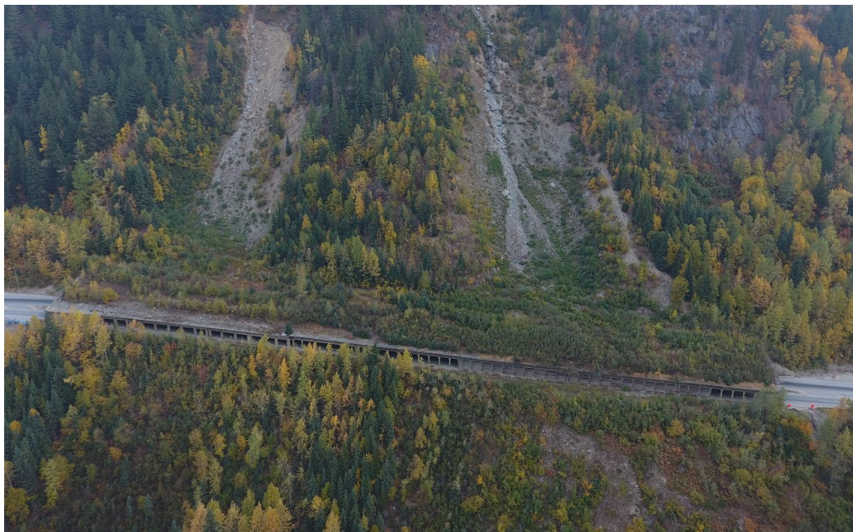
Figure 37: Debris and vegetation accumulation on top of the combined Tupper #1 (right) and Pioneer (left) snow sheds observed in 2017. A major shed rehabilitation program by Parks Canada has removed this debris and improved the management of surface and subsurface water (Photo: Dynamic Avalanche Consulting).
