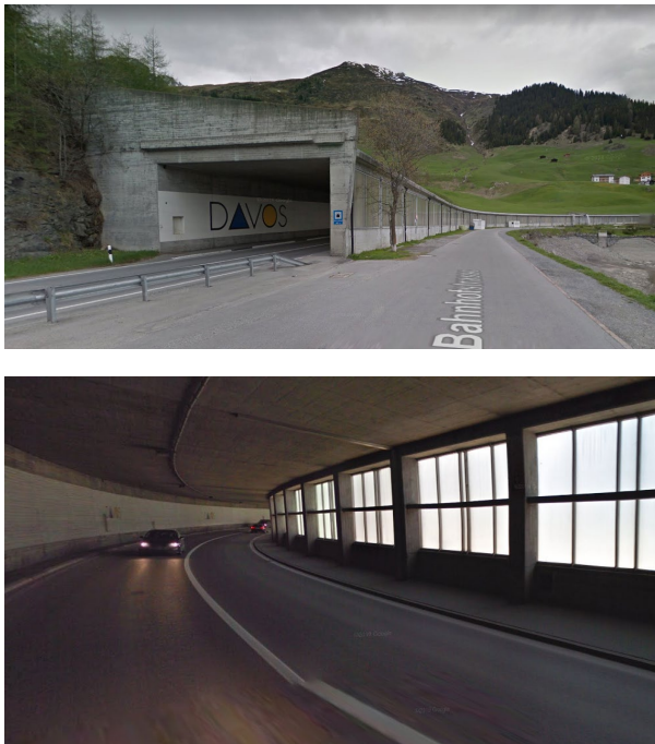
Figure 21: Snow shed Salez in Davos (constructed 1982, length 400 m) as viewed from the outside (Photo Google Earth, 2020), the inside and the cross section (from Tiefbauamt / Civil Engineering Office Graubünden, Switzerland)
