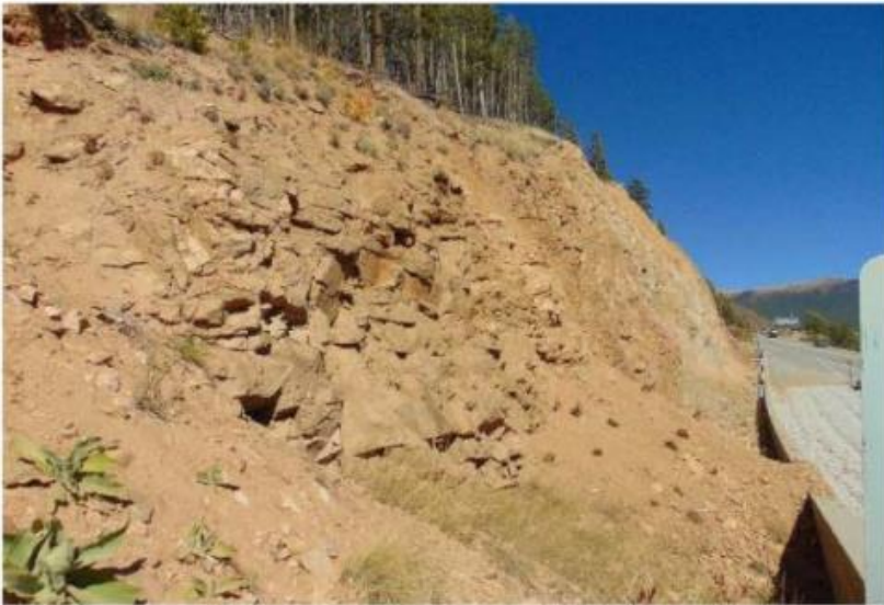
Fractured rock and loose rock on slope and behind barrier, view to east-northeast
