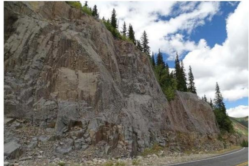
Draped mesh and bolts
