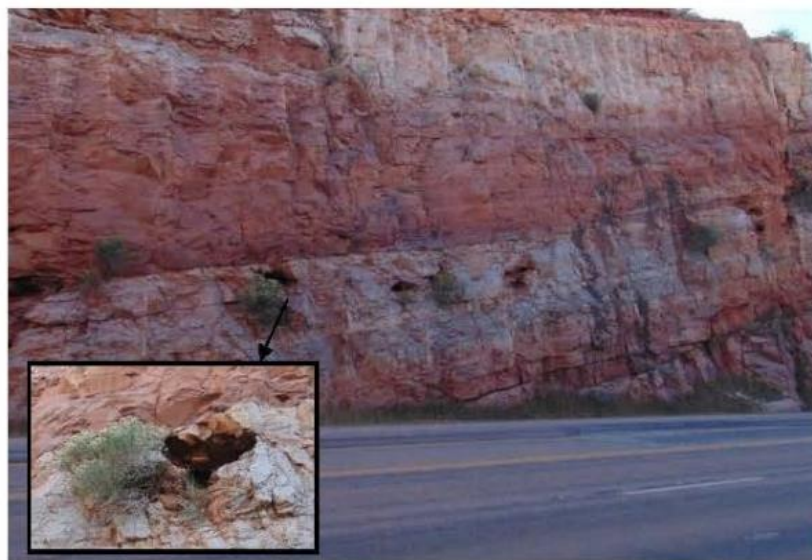
Dissolution cavities and boulders in ditch
