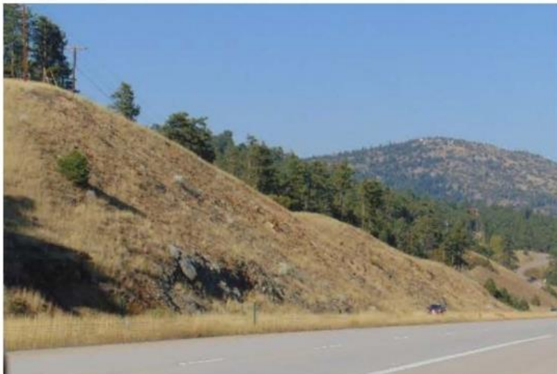
Cut slope mixed soil above rock
