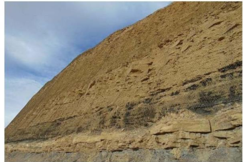
Draped mesh and soft carboniferous (coal) layer
