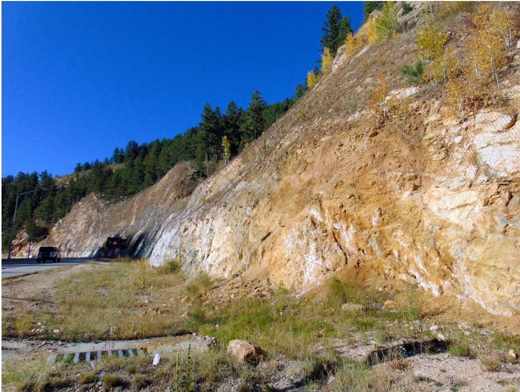
Figure 8. SH 119 MP 6 Catchment Ditch
