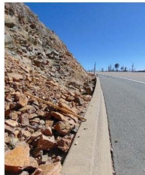
Rock filling behind barrier
