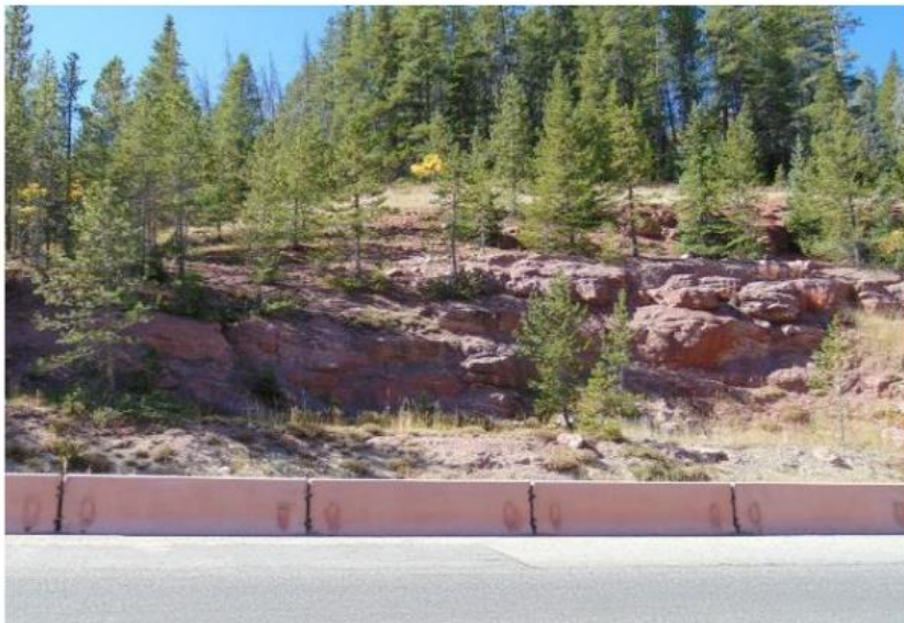
Bedding plane cuts with planting pockets
