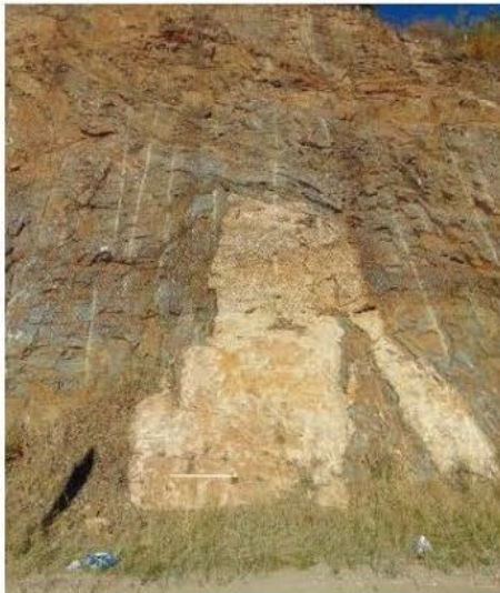
Draped mesh over half cast blast features
