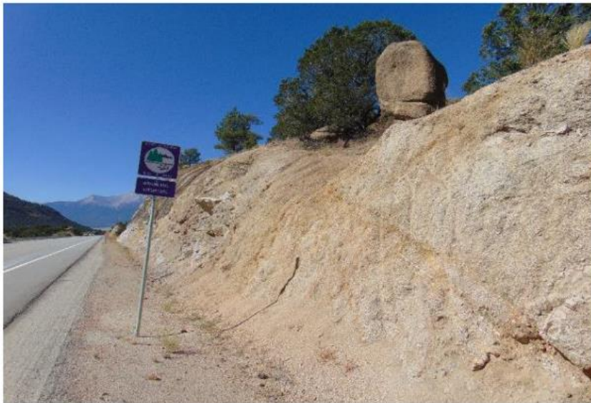
Machine marks in cut below perched boulder
