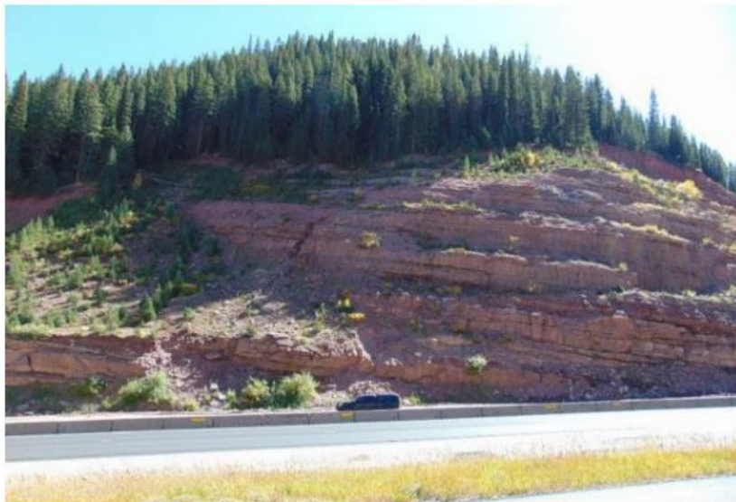
Terraced, bench slopes with revegetation
