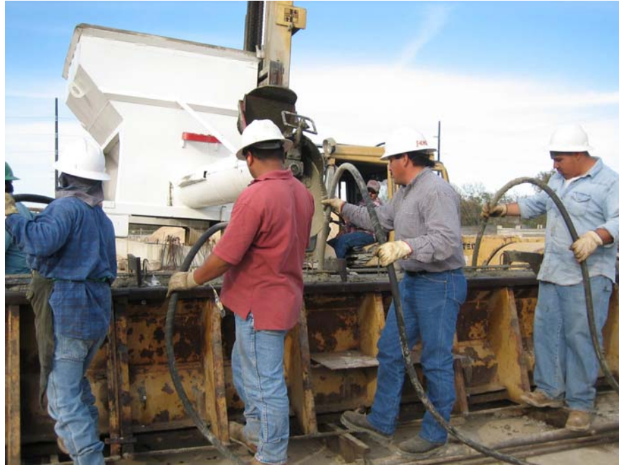
(b) Compaction using Needle Vibrators in Beam B4
