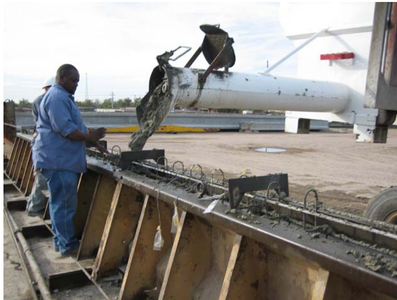
(a) Concrete Placed in Beam B4 by a Hopper
