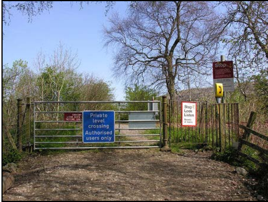
Figure 25. Private Highway-Rail Grade Crossing in Great Britain
