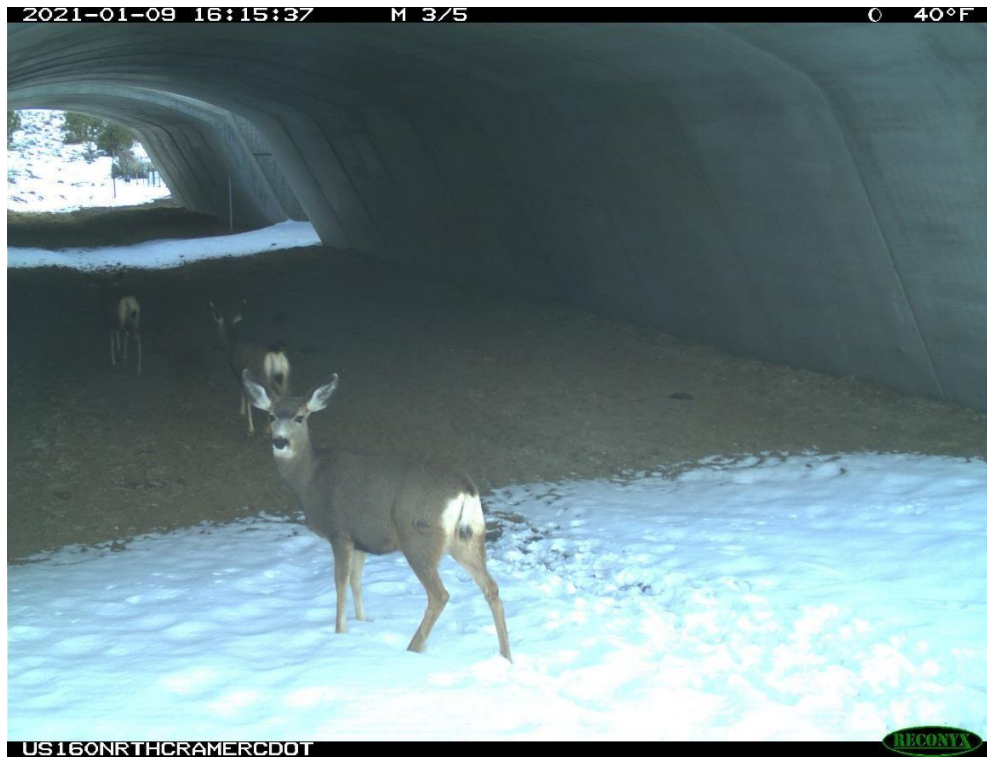
Mule Deer success movements through the wildlife crossing structure.
