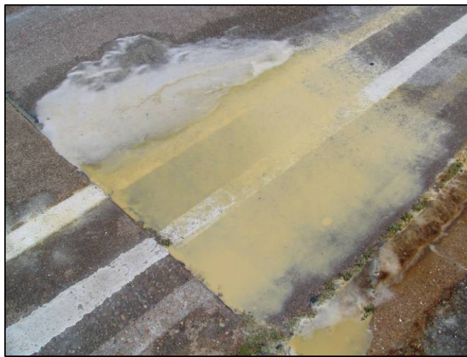
Figure 26. Liquid Mixture Remaining after Removal.
