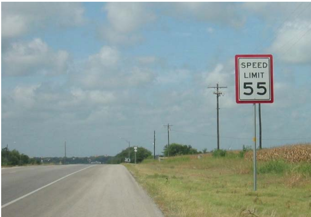
Figure 4-4. Site 1—Caldwell after 3 Inch Red Border Treatment.
