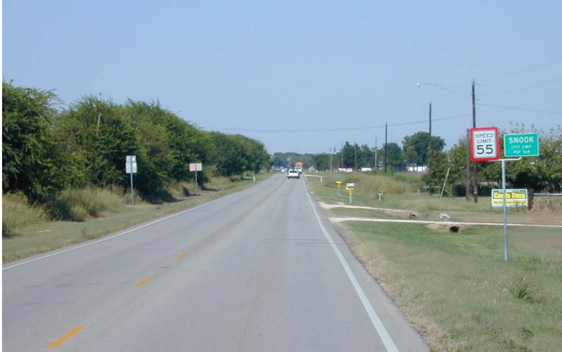
Figure 4-5. Site 2—Snook after 3 Inch Red Border Treatment.
