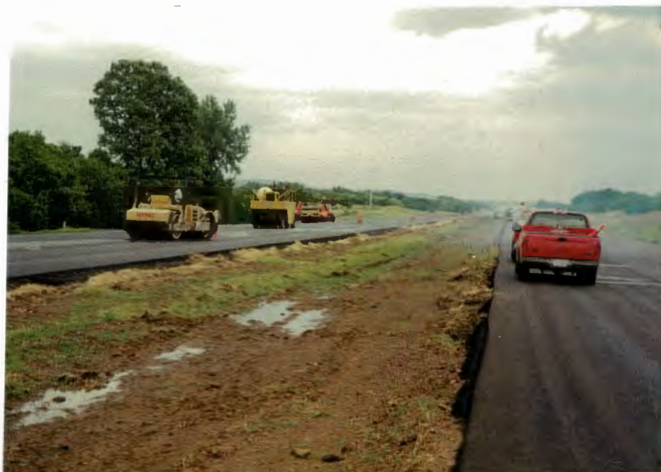
Photo 8. Compaction of 4005 Project
