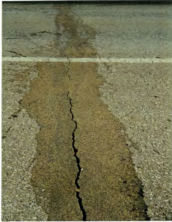
Photo 5. Transverse Crack
