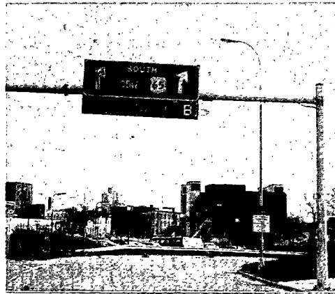
Bulb-Type Matrix and Static Sign Elements Used in Combination in Minnesota
