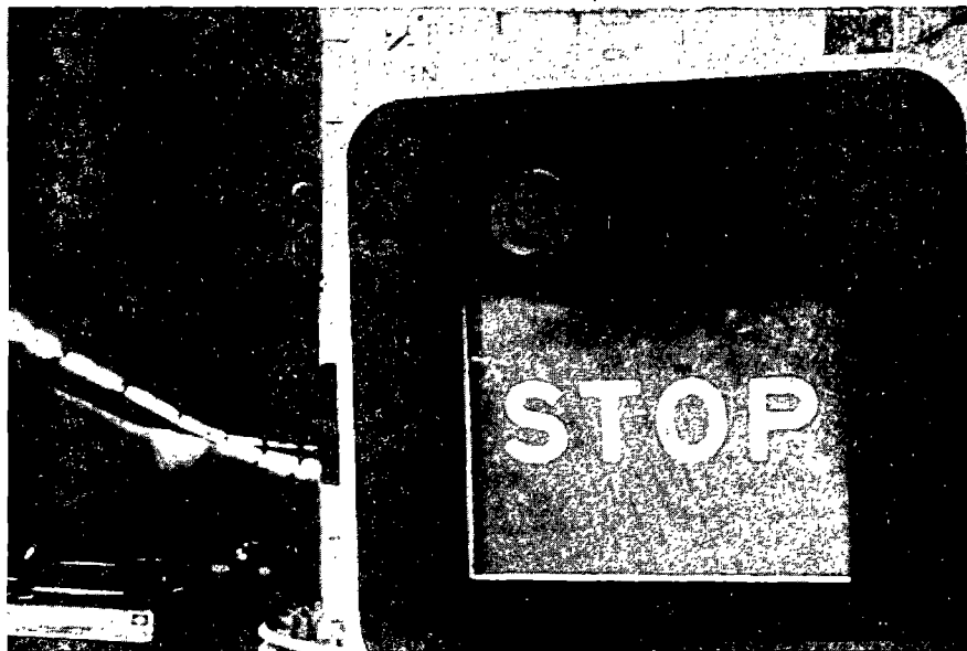
Figure 13-7. Scroll Sign Mounted at the Portal of the Lincoln Tunnel in New York
