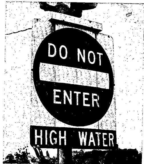
Figure 13-3. Electromechanically Operated Fold-Out Sign at High Water Crossing
