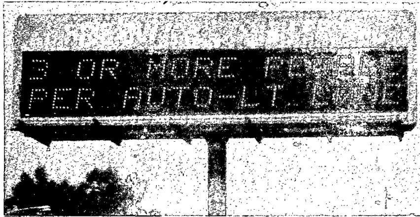
Figure 13-9. Bulb-Type Matrix Sign in Los Angeles, California
