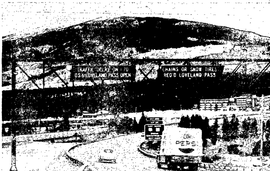
Figure 13-8. Rotating Tape Signs on I-70 near Dillion, Colorado
