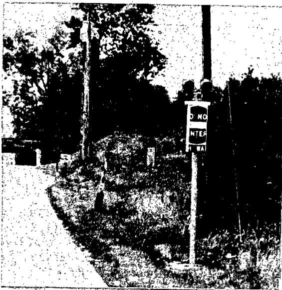
Figure 13-3. Electromechanically Operated Fold-Out Sign at High Water Crossing
