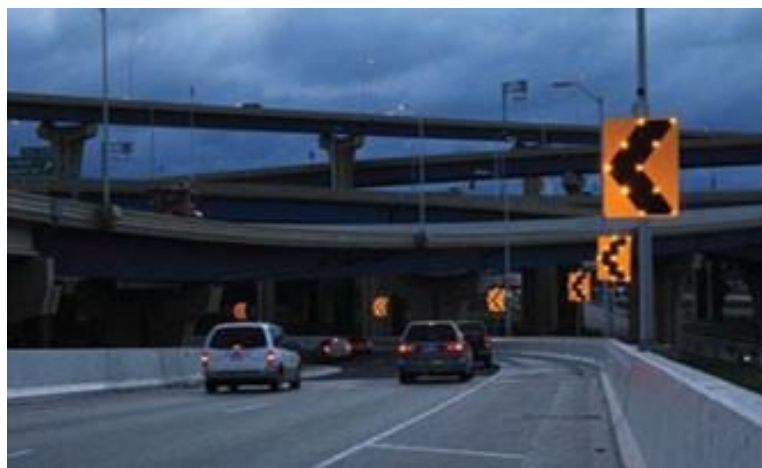
Figure 6.3: Sequential Dynamic Curve Warning Systems (SDCWS) (FHWA, 2016)
