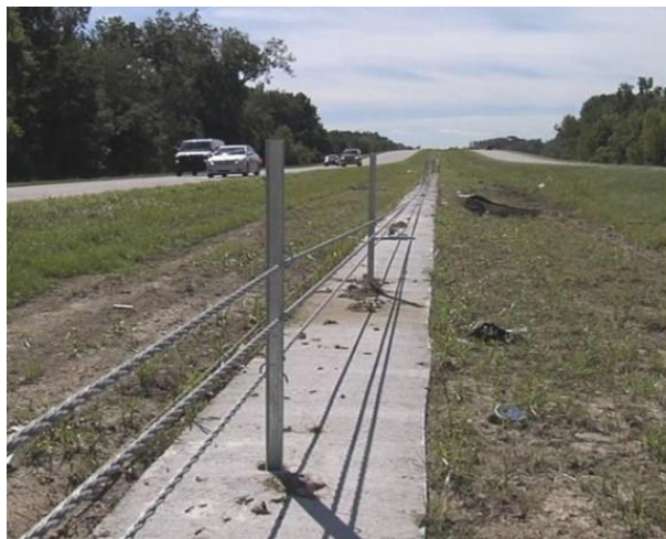
(a) Cable median barriers Source: Schmaltz (2016)
