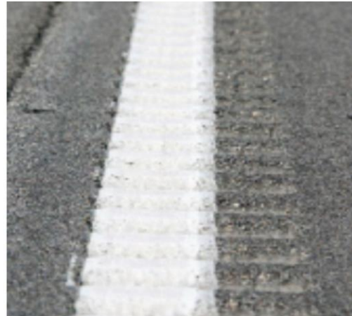
(b) Edge line rumble strips (FHWA, 2018)
