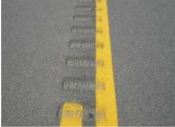
(a) Centerline rumble strips (FHWA, 2023)
