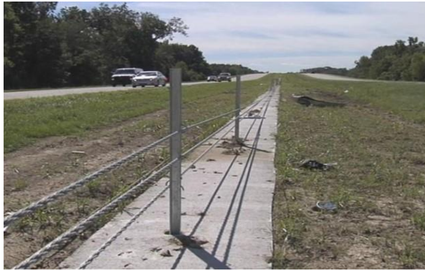
Figure 6.8: Cable Median Barrier ( Schmaltz, 2016)
