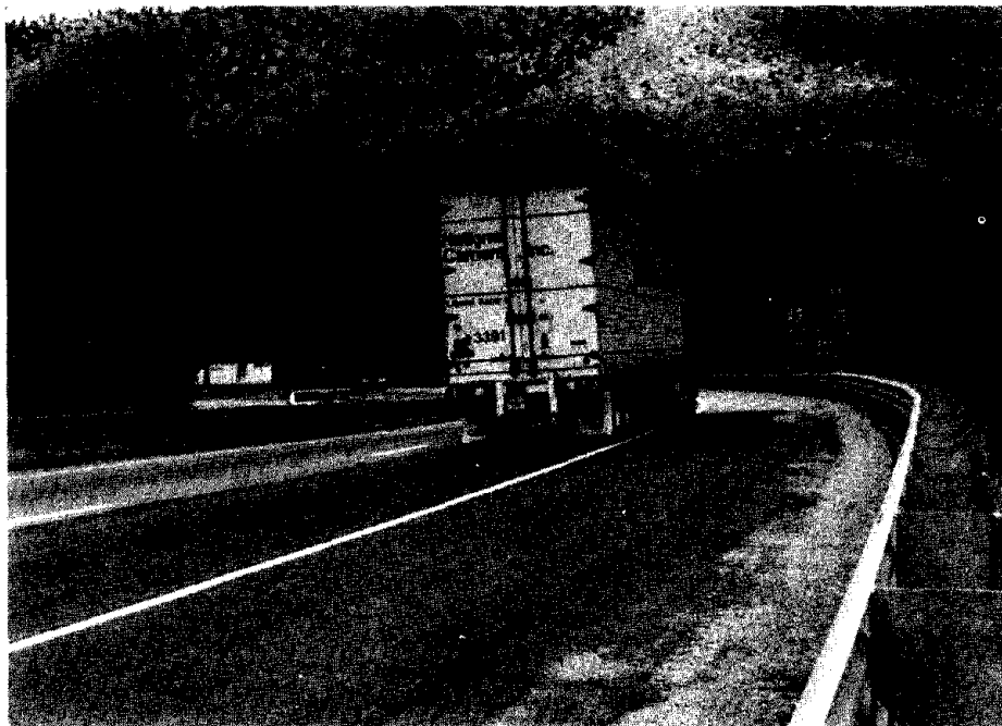
FIGURE 50: Modified Thrie Beam guardrail in advance of SERB guardrail.
