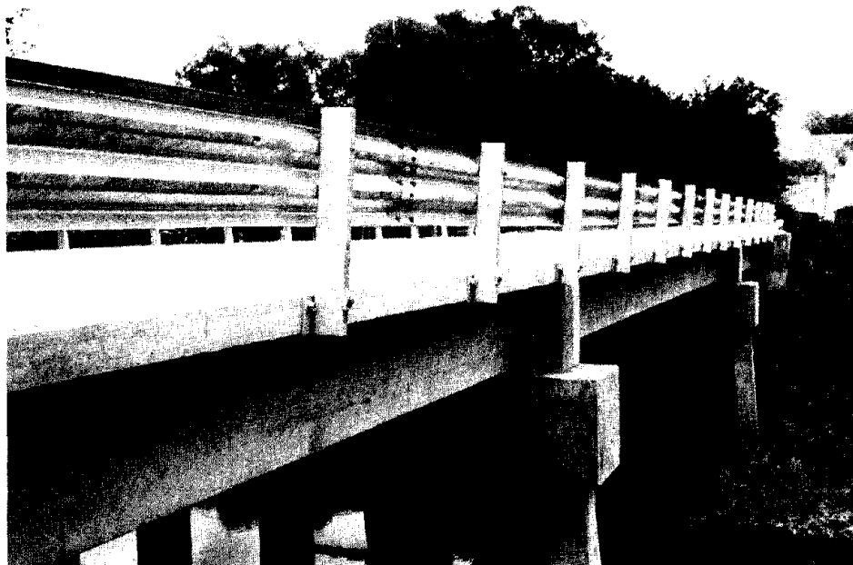
FIGURE 12: Completed SL1 Bridge Rail.
