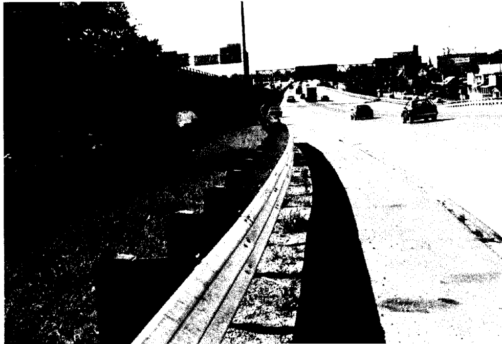
FIGURE 55: Modified Thrie Beam on 8-inch x 6-inch wood posts in Grand Rapids, Michigan.
