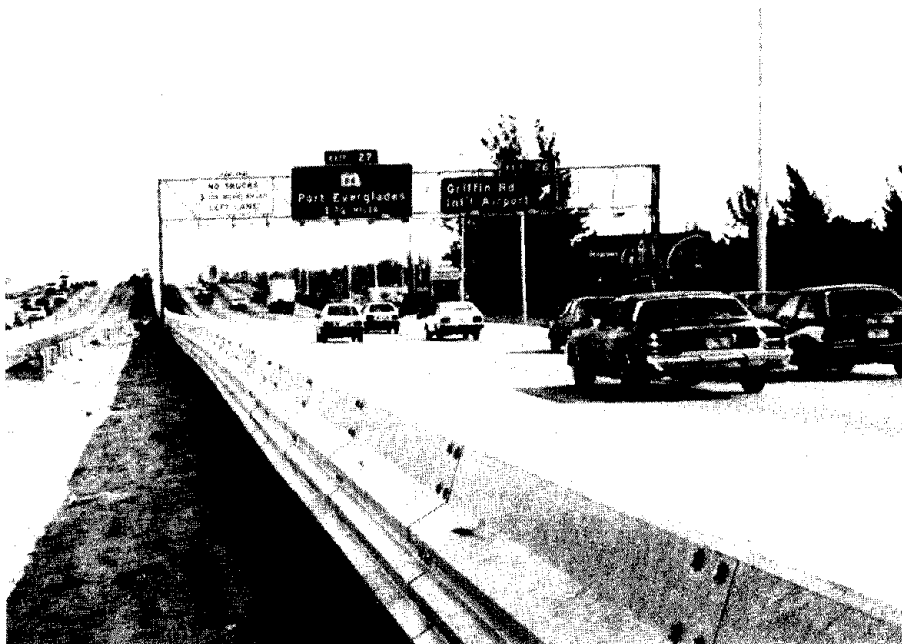
FIGURE 47: Completed section of IBC Barrier.
