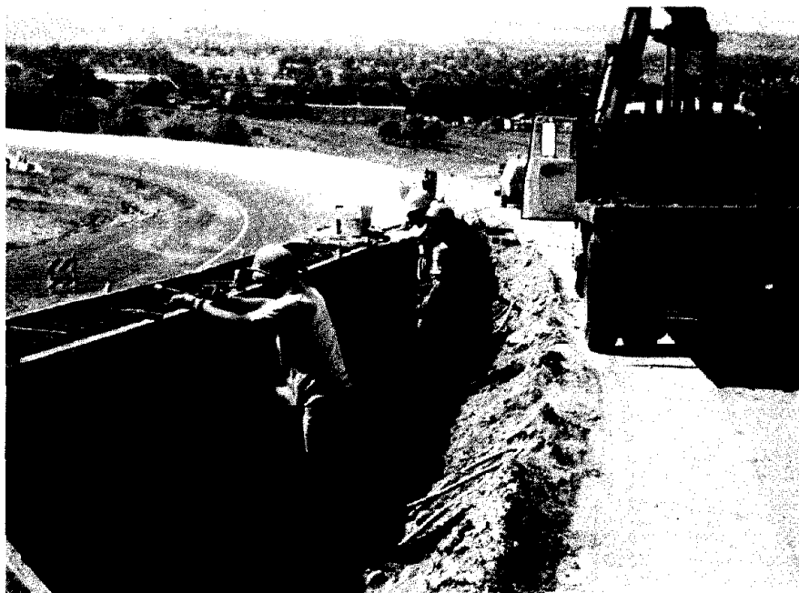
FIGURE 38: ...then placed into steel forms.
