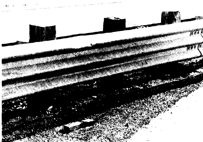
FIGURE 6: Total permanent damage after one years' service and approximately 20 hits.
