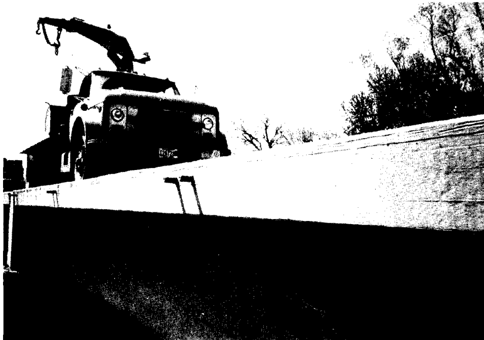
FIGURE 13: On new construction, accurate placement of the base plate anchor bolts is essential.
