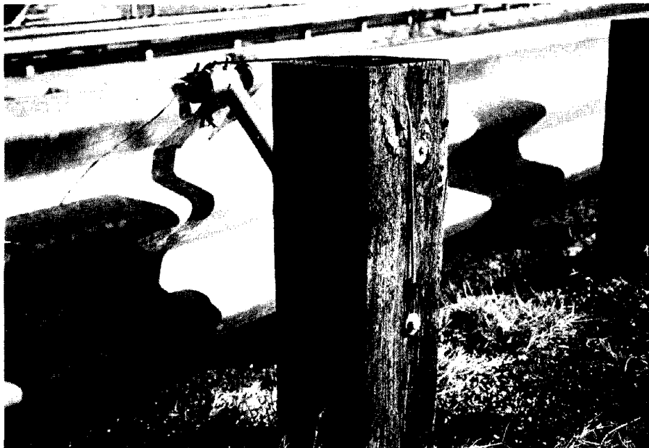
FIGURE 4: Extended restraining cable prevents lag-bolt pullout, but back edge of post should be reinforced to eliminate problem shown above.
