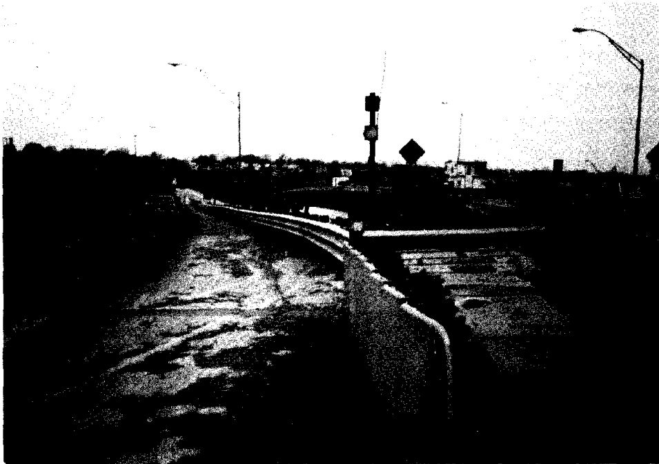
FIGURE 10: SERB begins at gore area and extends along the right side of the ramp.
